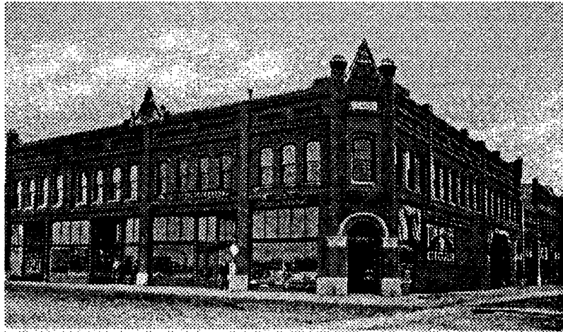
Southeast Corner of 4 th & Main. Building has been radically altered
