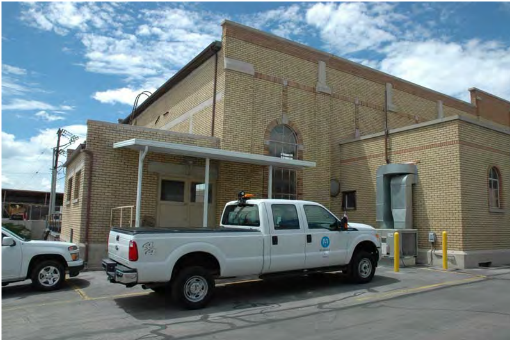
Photograph 5 of 17 Southeast corner of Murray City Diesel Power Plant. Camera facing northwest.
