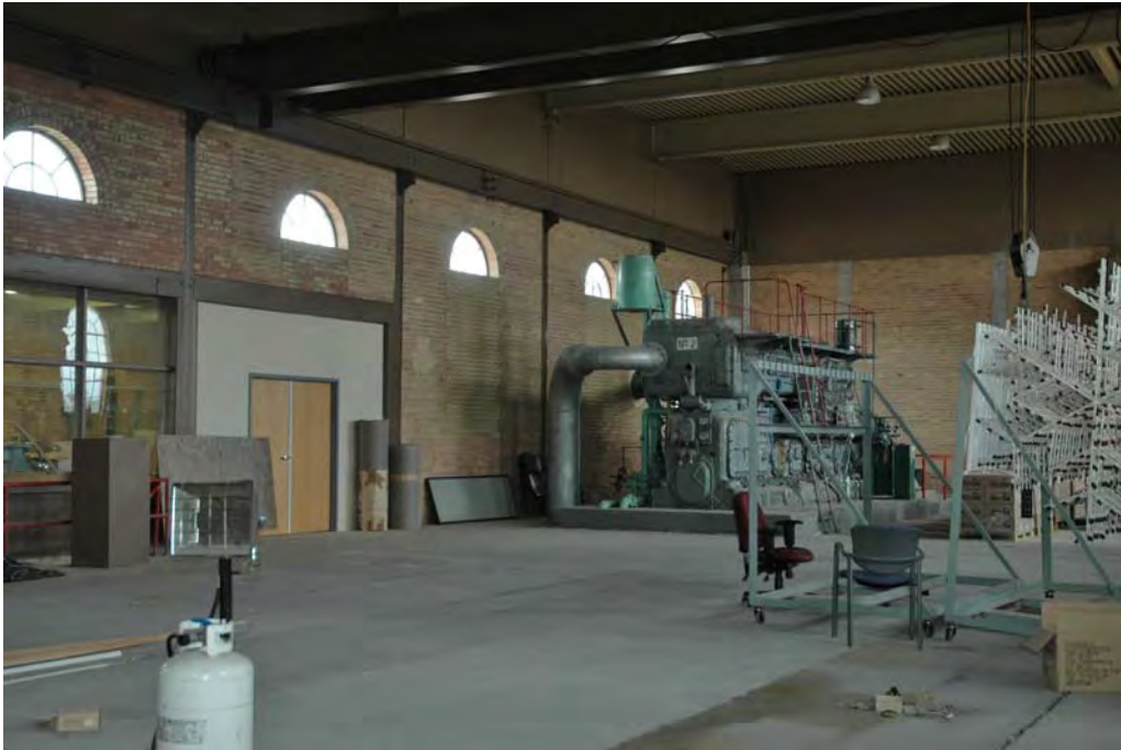
Photograph 10 of 17 Murray City Diesel Power Plant, interior, main floor. Camera facing southeast.
