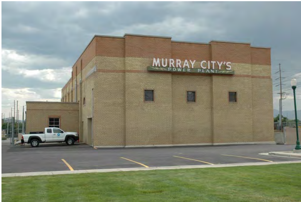
Photograph 1 of 17 North elevation of Murray City Diesel Power Plant. Camera facing south.
