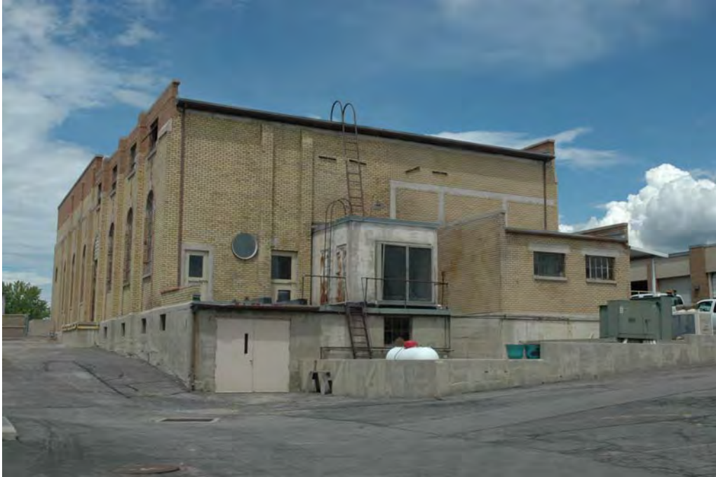
Photograph 4 of 17 South elevation of Murray City Diesel Power Plant. Camera facing northeast.
