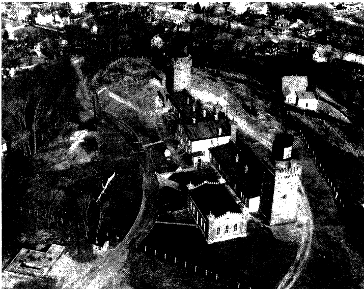
Figure 13: Bird's-eye-view of Navesink Light Station, circa 1940s, USCG Historian's Office.
