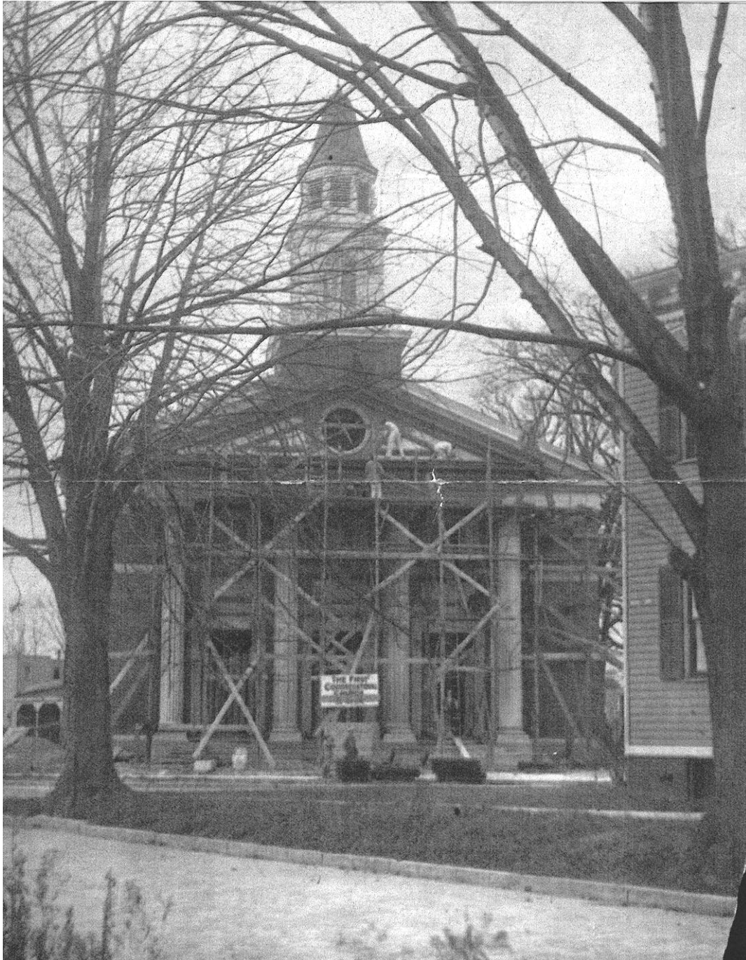
First Congregational Church under construction (ca. 1918)
