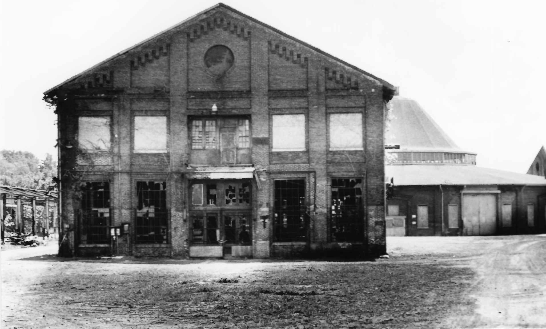
Photograph #2 B&O RAILROAD MARTINSBURG SHOPS Martinsburg, WV North facade of Machine/Woodworking Shop, looking south. Michael Caplinger, IHTIA, August 2001
