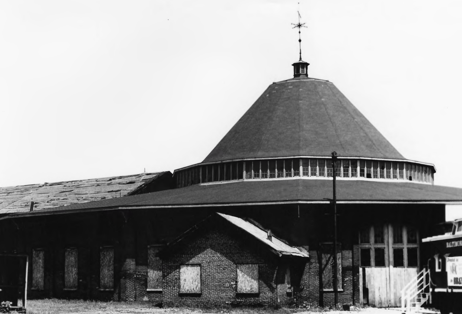
Photograph #7 B&O RAILROAD MARTINSBURG SHOPS Martinsburg, WV Southwest facade of West Roundhouse, looking northeast. Michael Caplinger, IHTIA, August 2001
