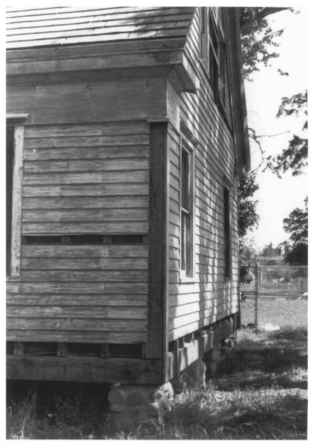
Hall Blvd., Beaverton, Wash. Co., OR \*House detail, improvements = rock pi s and foundation work, paint removed, and new single (Cedar ) roof.
