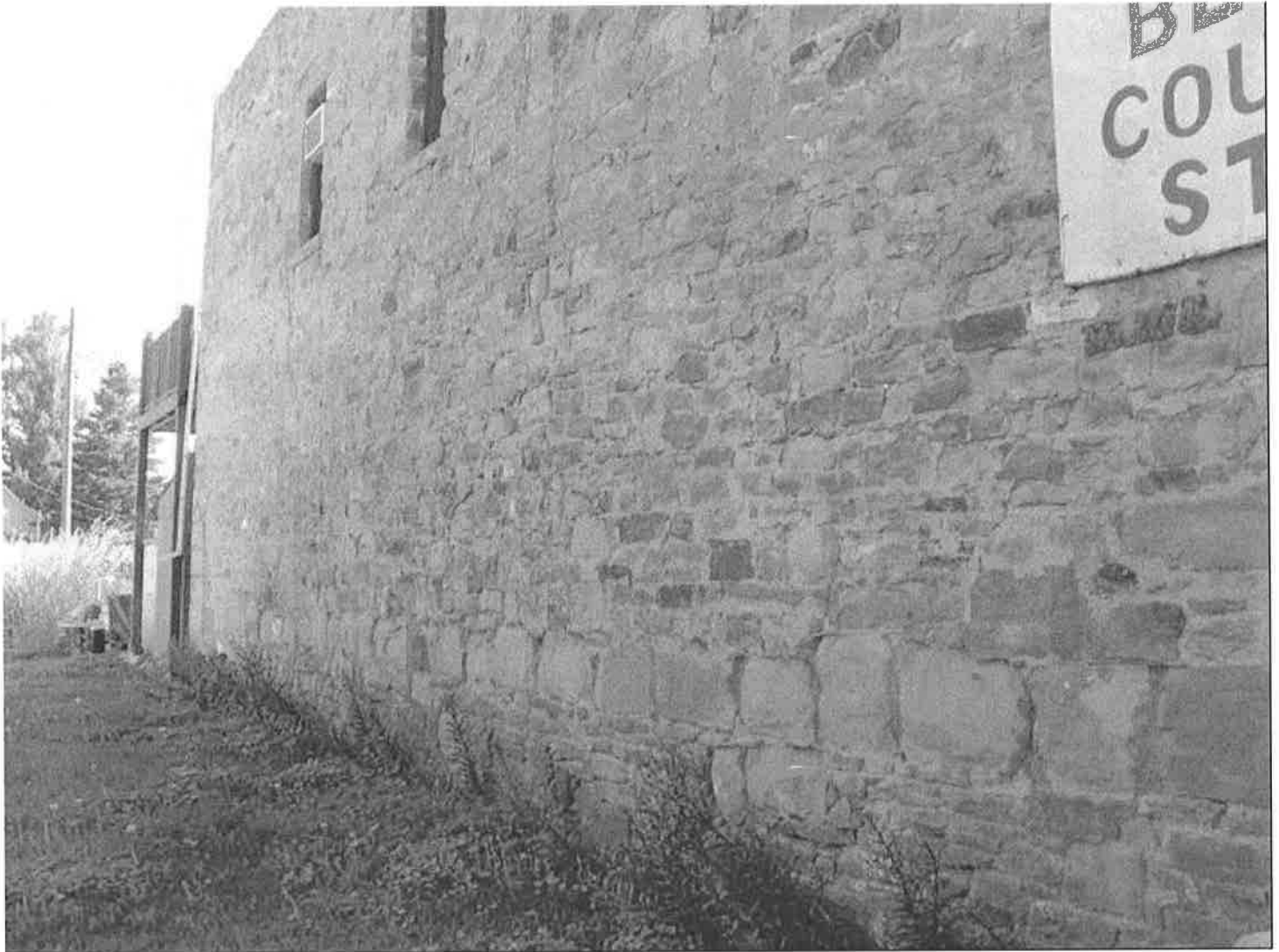
Photo 0003. Detail of east elevation. View to the southwest.
