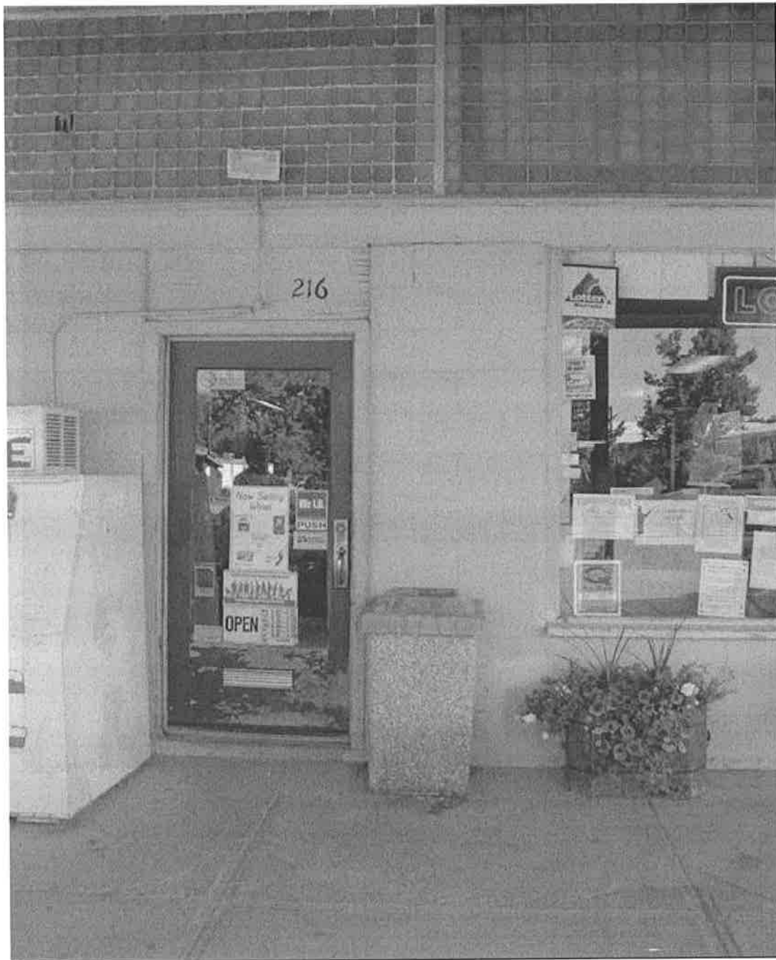
Photo 0009. Detail of entry. View to the south.
