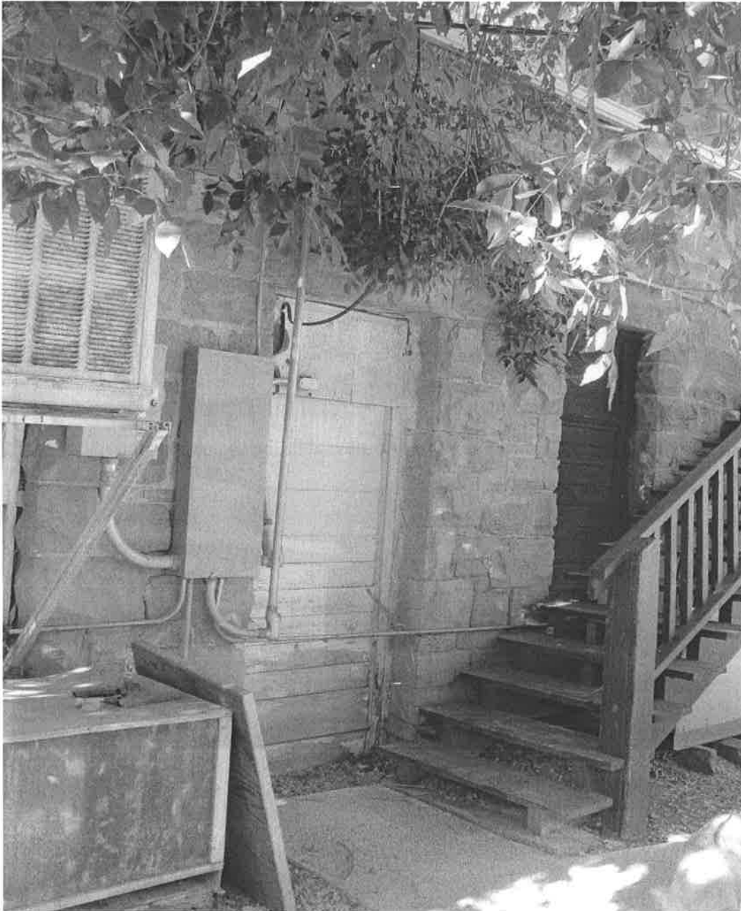
Photo 0006. Detail of entry. South façade. View to the northeast.
