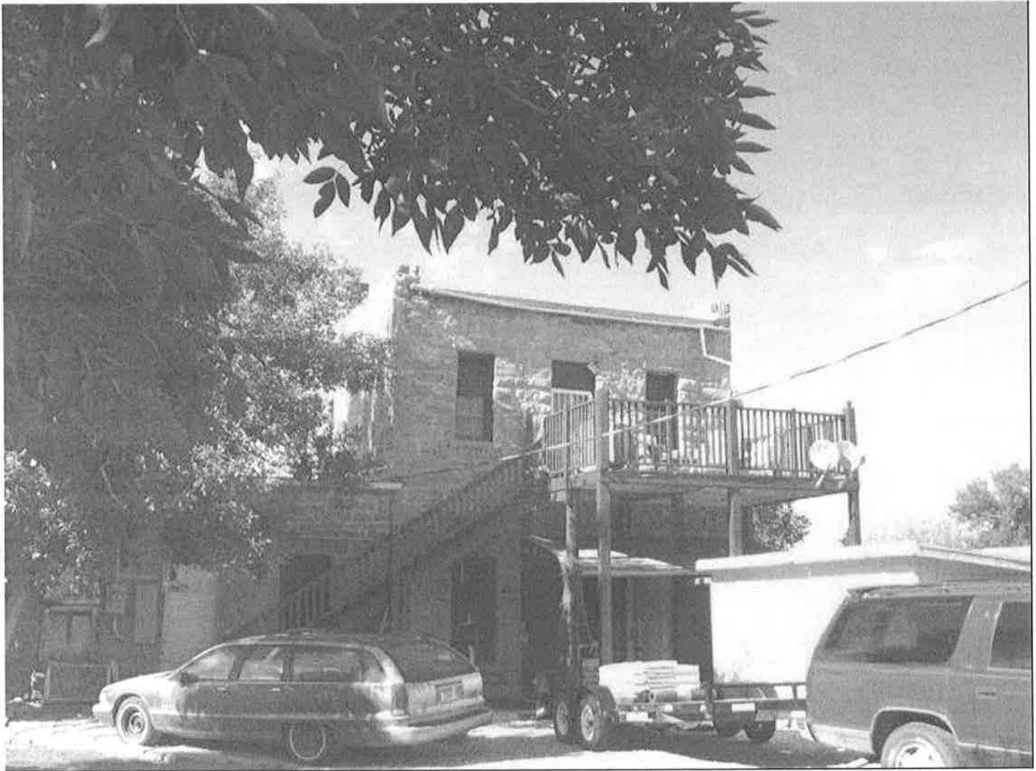
Photo 0005. Overview of south façade. View to the northeast
