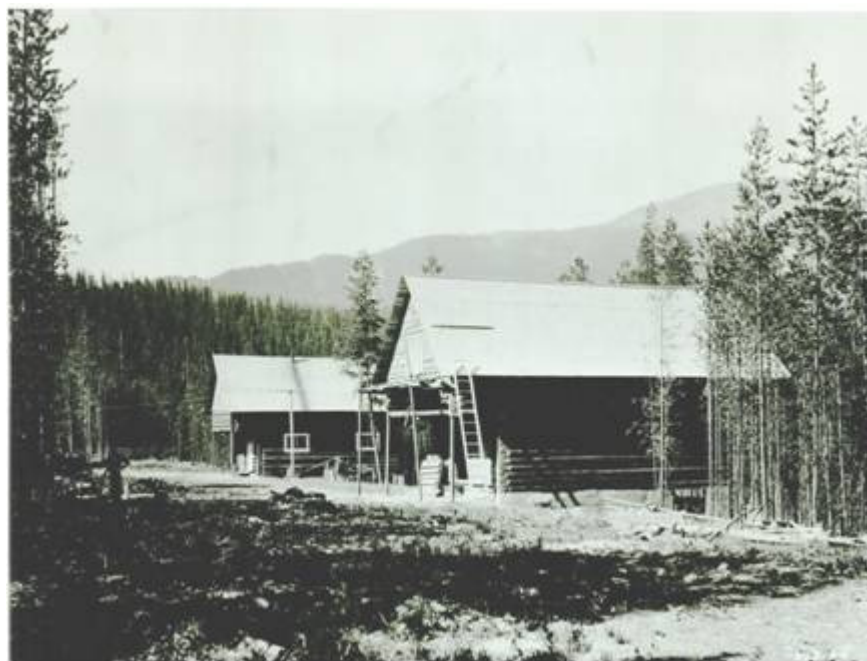
Figure 31. Warehouse under construction with the completed office building behind (HF FNF).
