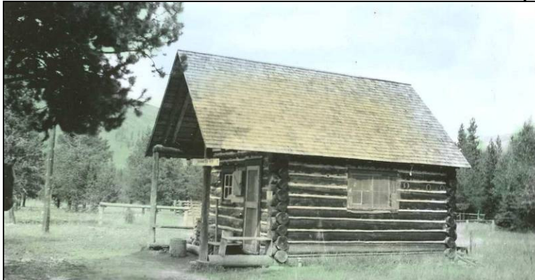
Figure 26. Undated photograph of Hahn Cabin, a “C-1” style building executed in logs (Photo No. 2756 FNF HF).
