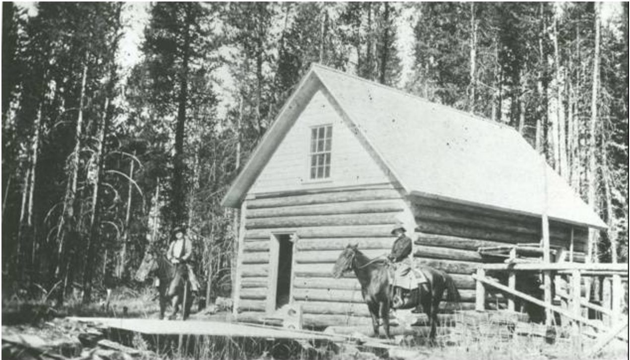
Figure 32. New ranger's office/residence built in 1916 at Big Prairie Ranger Station. After construction of yet another ranger dwelling in the early 1930s, this building was used for a time as a bunkhouse. It is currently referred to as the "Packer's dwelling" (Photo No. 1066 HF FNF).
