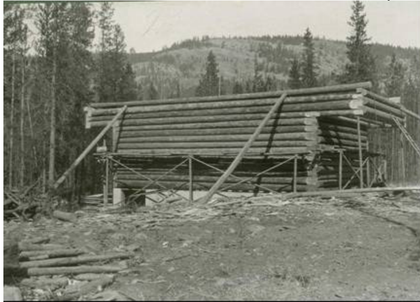
Figure 30. Spotted Bear Ranger Station office under construction, 1923 or 1924 (Photo No. 0482, HF FNF).
