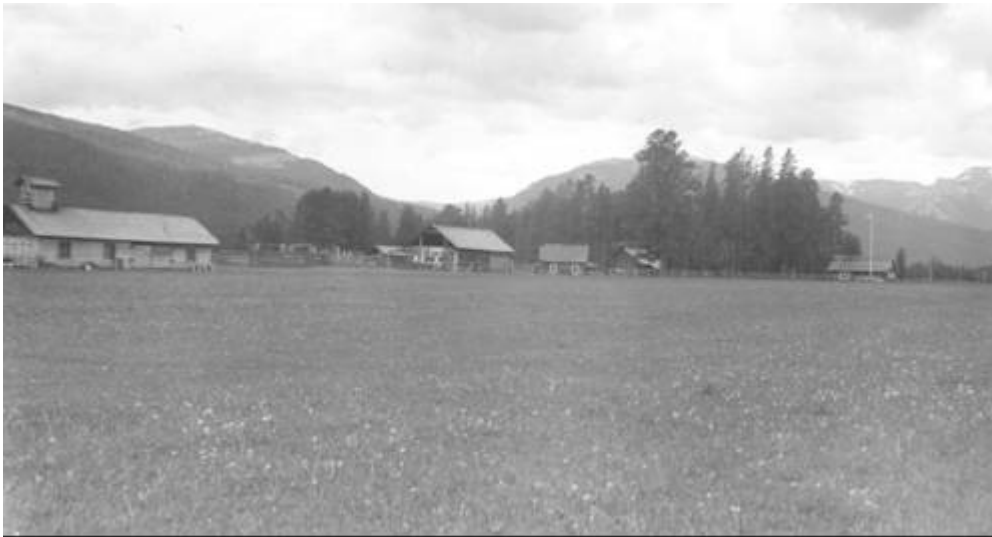
Figure 35. Overview of the Big Prairie Ranger District headquarters complex looking northwest, taken from the middle of the landing strip, sometime in the early 1960s. The warehouse (also known as the chute shed) is at the left edge of the photo. Also visible: the building known currently as the “packer’s dwelling” and the 1938 bunkhouse; the combination building and flagpole are near the right edge of the photo (Photo No. 2202 HF FNF).
