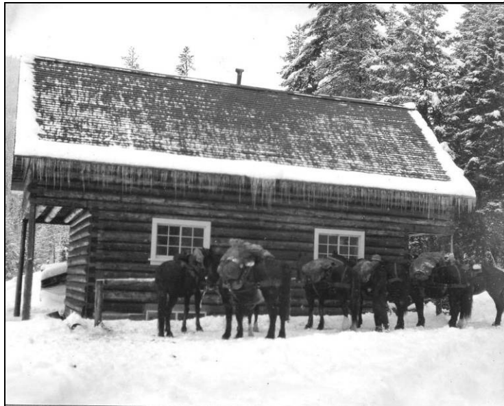
Figure 29. Black Bear station, November 15, 1927 (Photo no 0352 FNF HF). Black Bear Cabin is one of five similar buildings with a design unique to the Flathead National Forest.
