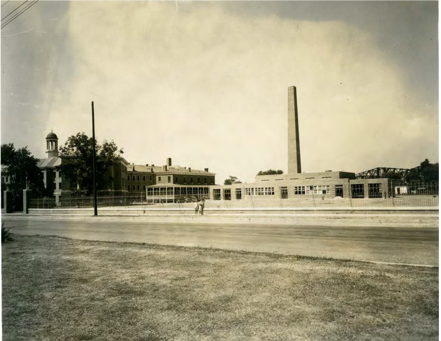
Photograph taken September 1, 1939, showing from left to right the U.S. Marine Hospital (Building 1- with the 1937 main building and 1934 rear wing visible), Nurses Quarters (Building 2), and Steam Laundry (Building 3)
