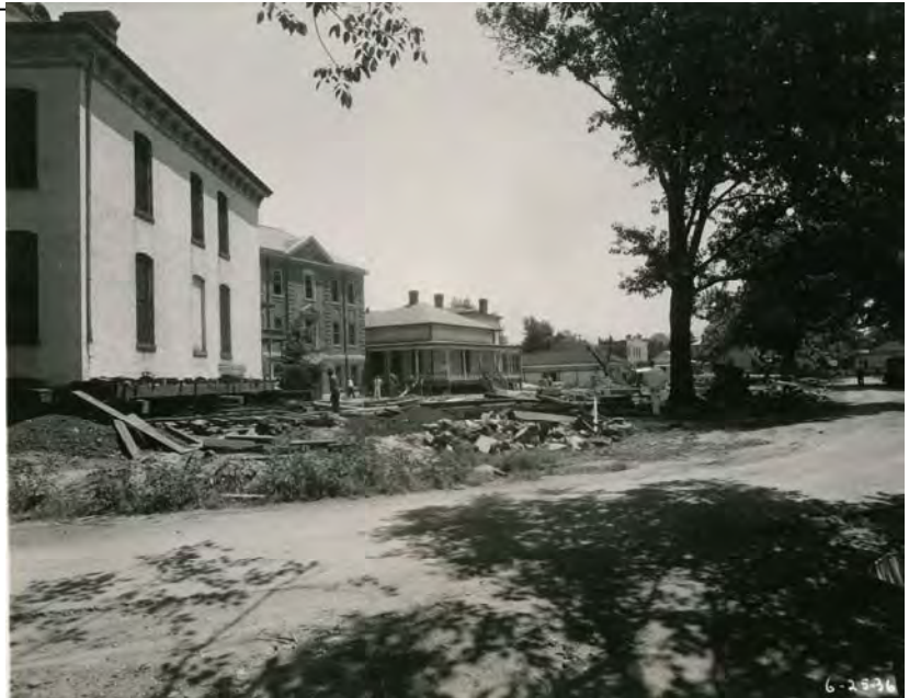
View during construction in 1936, showing 1884 Executive Building in the process of being relocated. Note presence of completed 1934 building (Building 1) and relocated Nurses' Quarters (Building 2) beyond.
