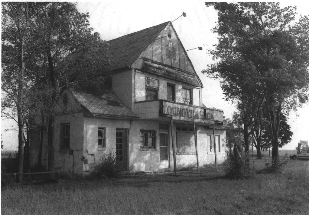
Abandoned and derelict Youngville Café in 1995, View to the Northeast
