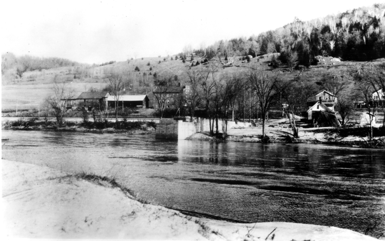
Figure 2. Undated photograph (pre-1946) of the Fox Stand and outbuildings, view northeast across the White River (private collection).
