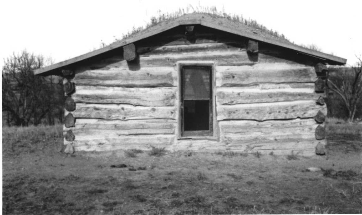
"HO" Ranch Log House, Meade County, S. D., No. 2
