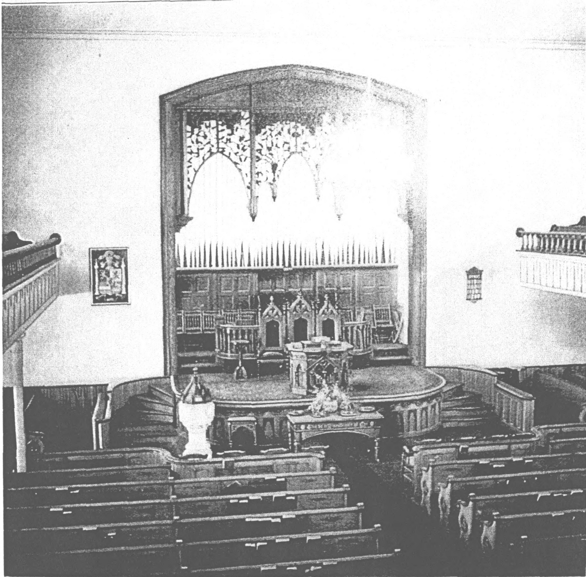
Historic Photograph 9 of 9: A photograph of the church interior following a major redecoration in 1921 reveals that the elaborate ceiling and trompe l'oeil wall decorations have been replaced by plain, light-toned finishes. The organ pipes have also been repainted in white, along with parts of the gallery fronts and support columns. Also note the installation of the delicate Art Nouveau pipe-shade over the organ.
