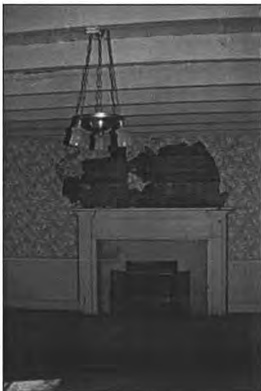
Figure 4: Thomas Williamson House in 1996. West Parlor, First Floor, facing west.
