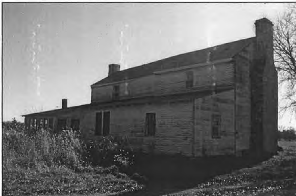
Figure 3: Thomas Williamson House in 1996. North elevation, facing southeast.
