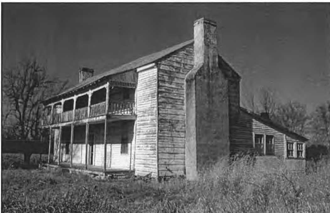
Figure 2: Thomas Williamson House in 1996. East elevation, facing northwest.
