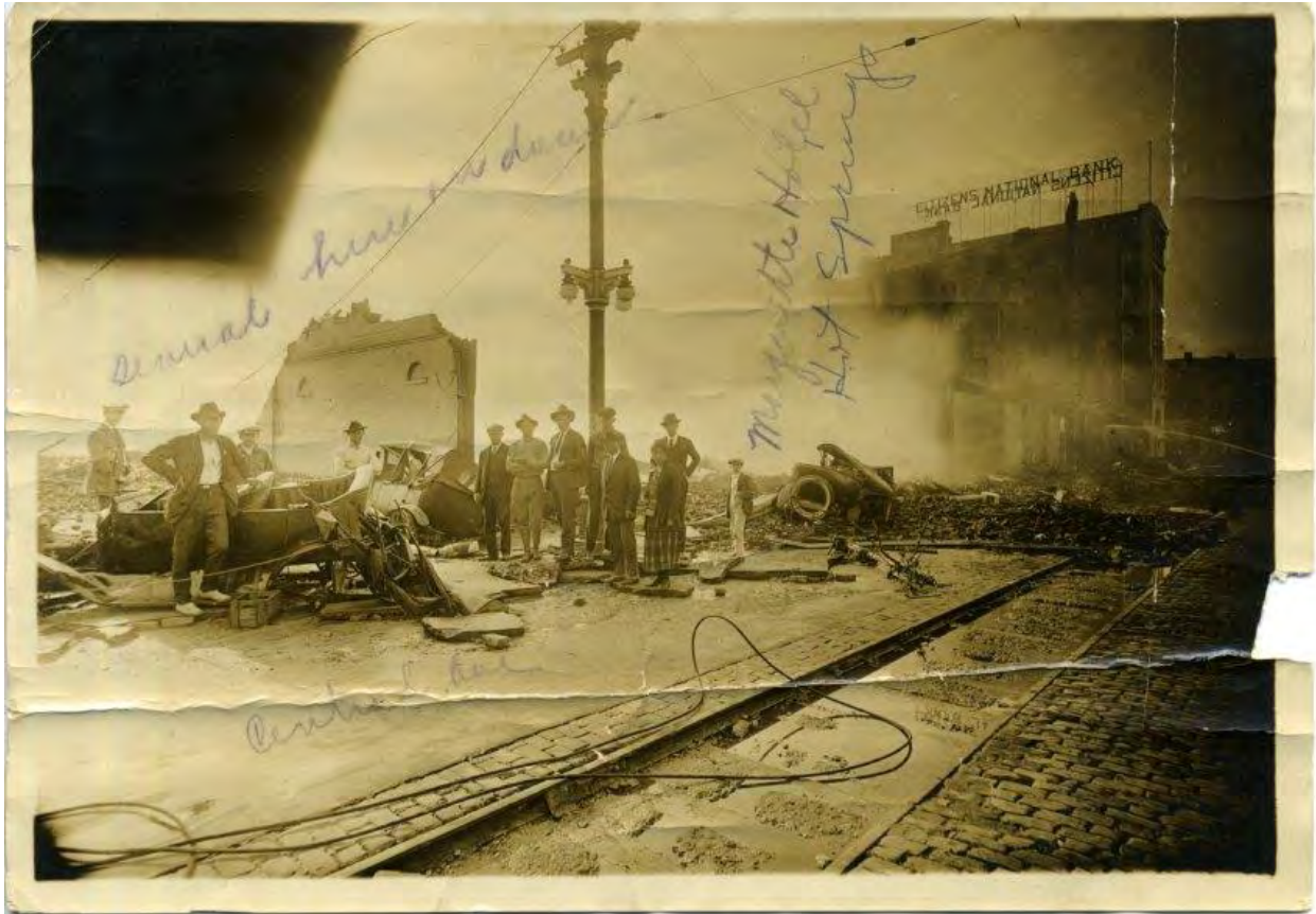
Figure 10. Fire damage at the 700 block of Central Avenue, May 14, 1923 (Garland County Historical Society Archives, Photograph Collection).
