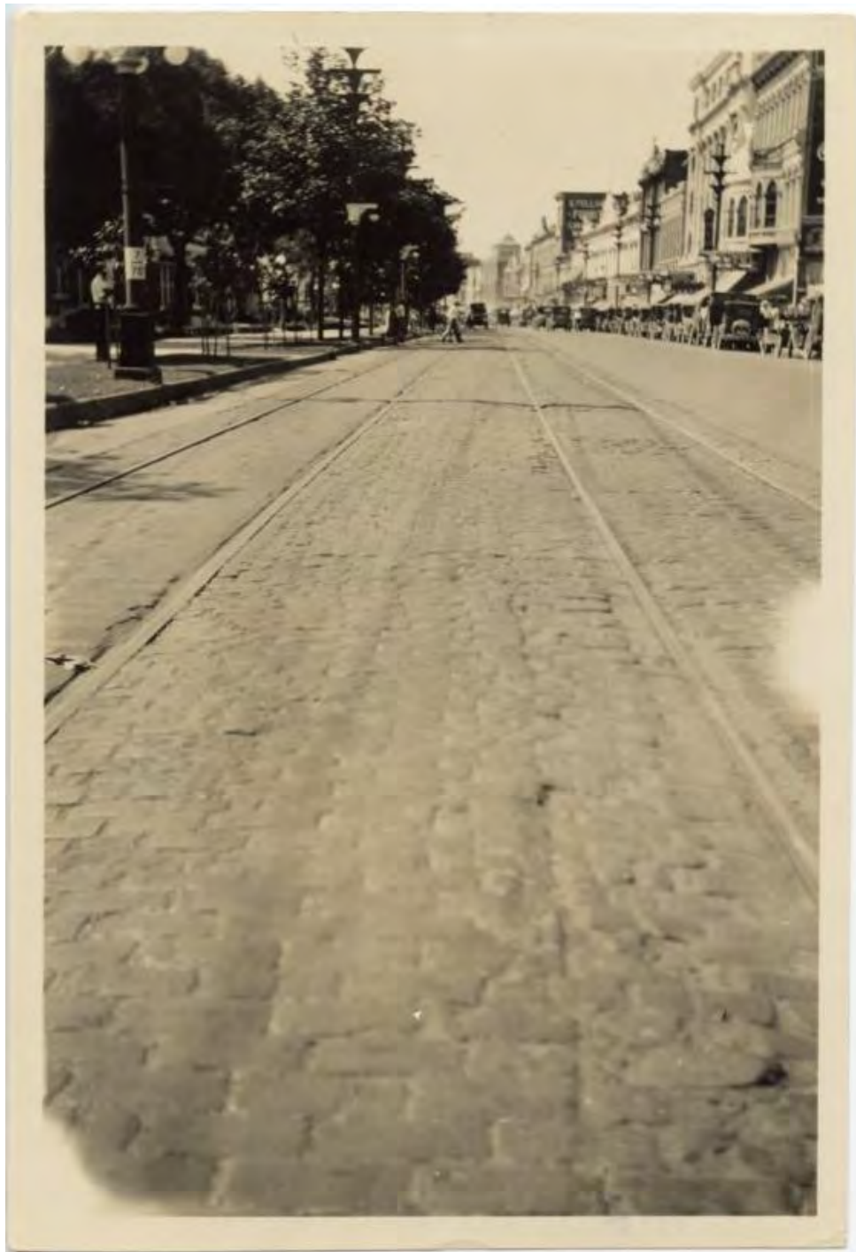
Figure 7. Brick pavers at streetcar tracks along Central Avenue, c. 1915 (Garland County Historical Society Archives, Photograph Collection).
