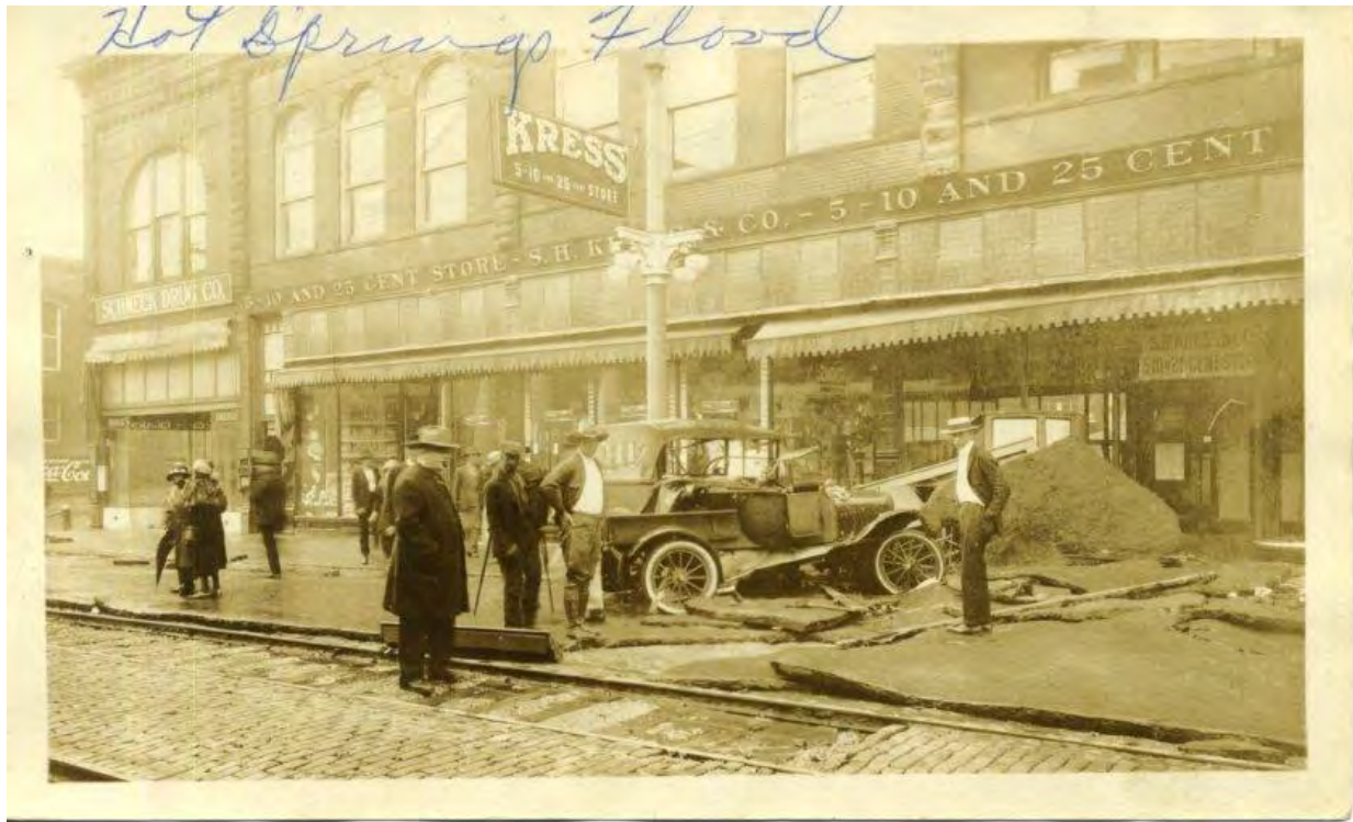
Figure 9. Flood damage along 600 block of Central Avenue, May 14, 1923 (Garland County Historical Society Archives, Photograph Collection).
