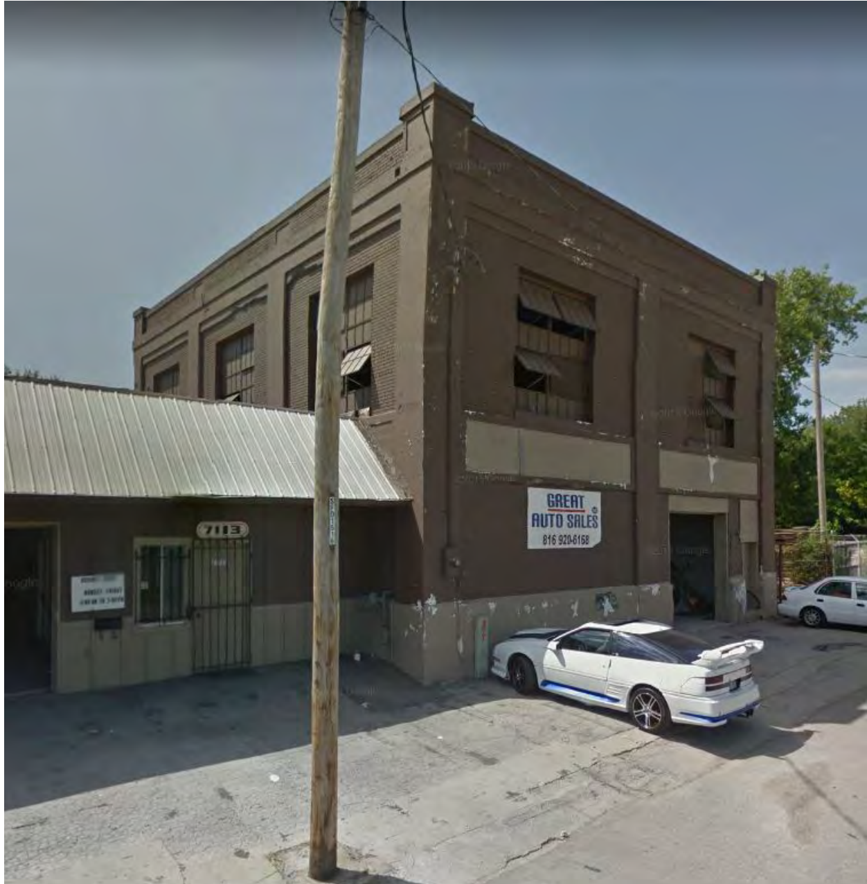
Figure 15. Substation F (constructed 1928), 7109 E. 12 th Street, 2017. Source: Google Street View. Accessed September 2017.
