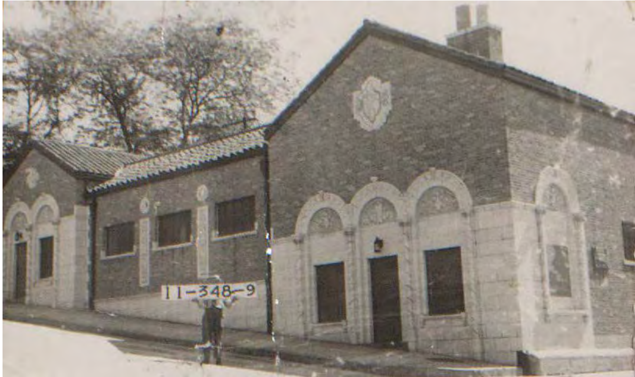
Figure 16. Substation H (constructed 1931), 4600 block of Broadway, 1940 Tax Assessor photograph. Source: Missouri Valley Special Collections .
