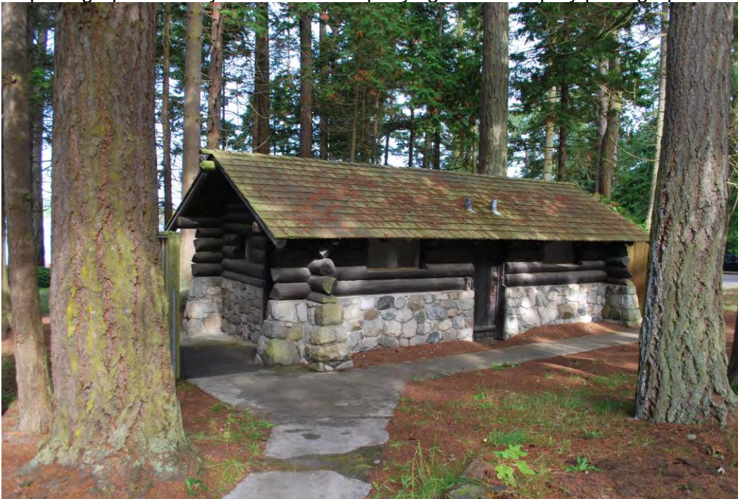
Photo 1 of 14: Latrine (ID#1), view to northwest taken 8/1/2012.
