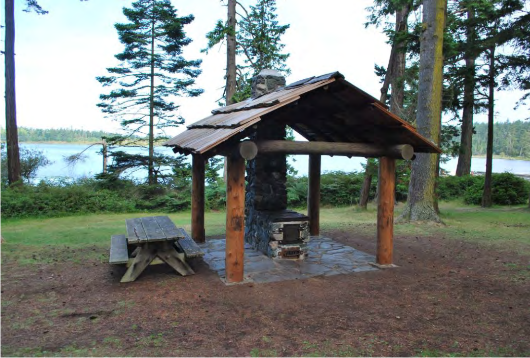
Photo 6 of 14: Campstove Shelter (ID#4), view to west taken 8/1/2012.
