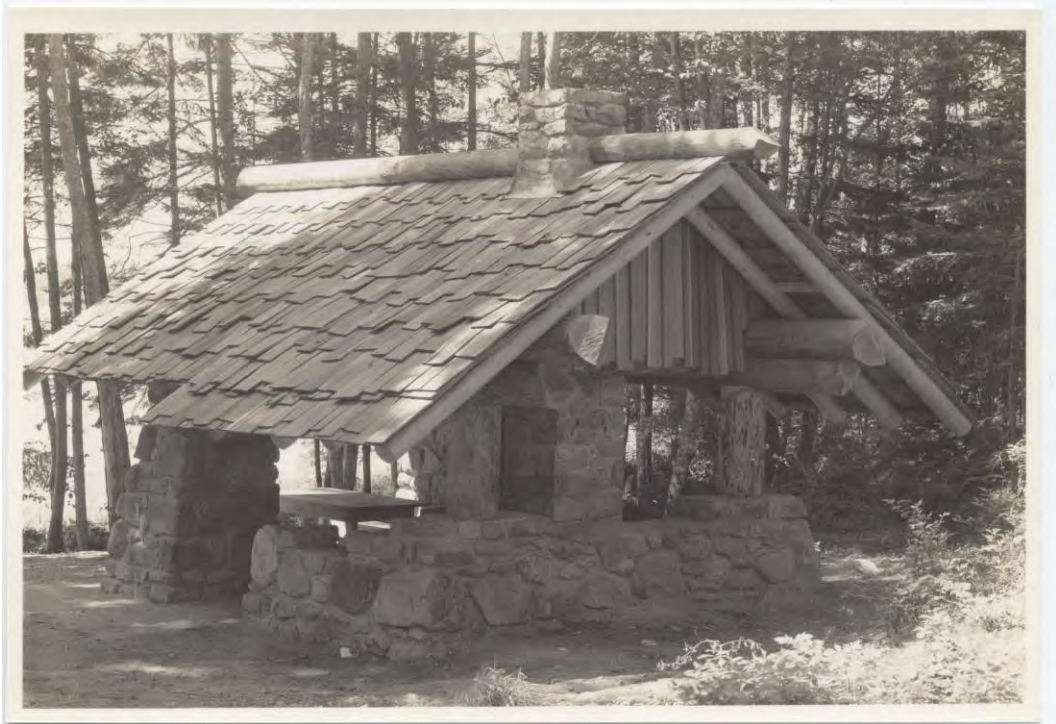
Completed Shelter Kitchen (ID#3), view to northwest.
