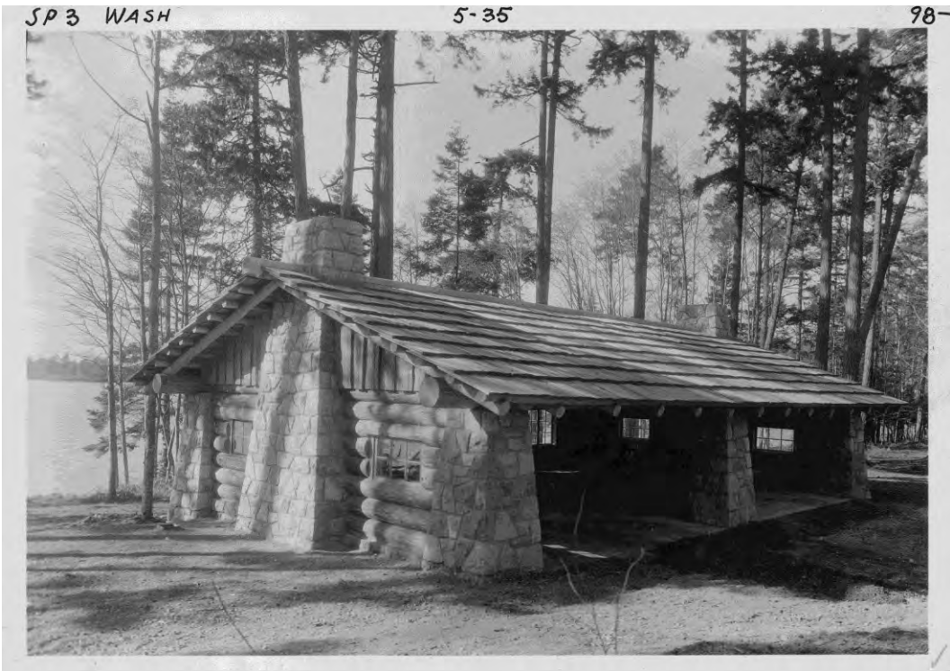
Completed Combination Building (ID#2), view to northwest.
