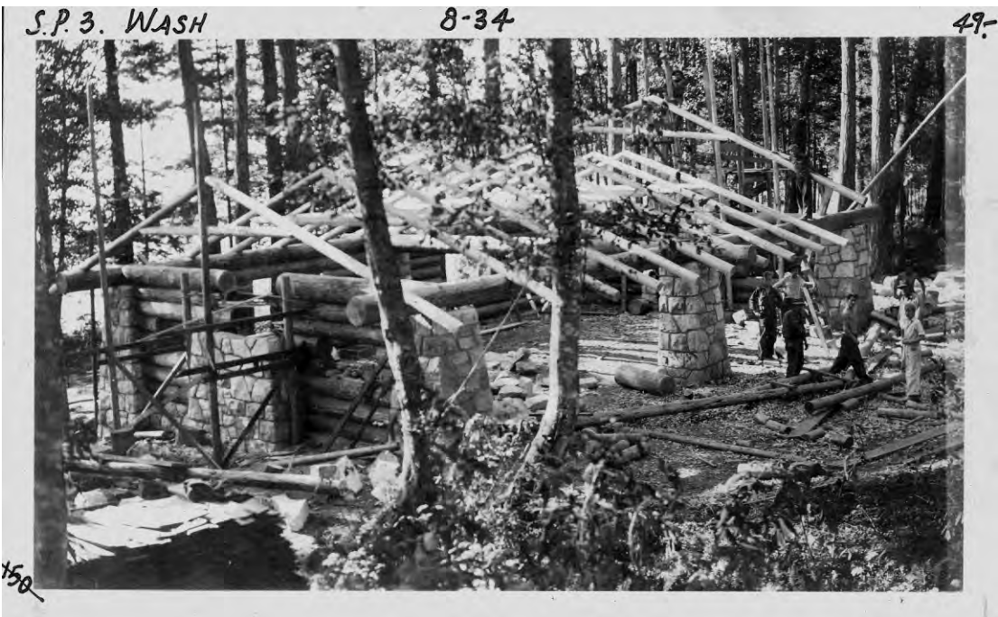
Combination Building (ID#2) under construction, view to northwest.
