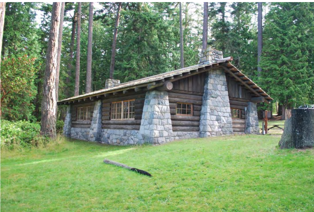
Photo 3 of 14: Combination Building (ID#2), view to northeast taken 8/1/2012.
