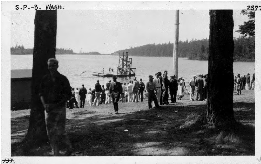
General view towards Cranberry Lake from a point southwest of the former Bathhouse.
