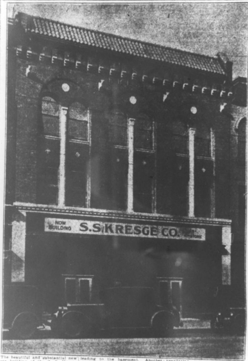
The beautiful and substantial new leading to the basement. Another ventilating system is
