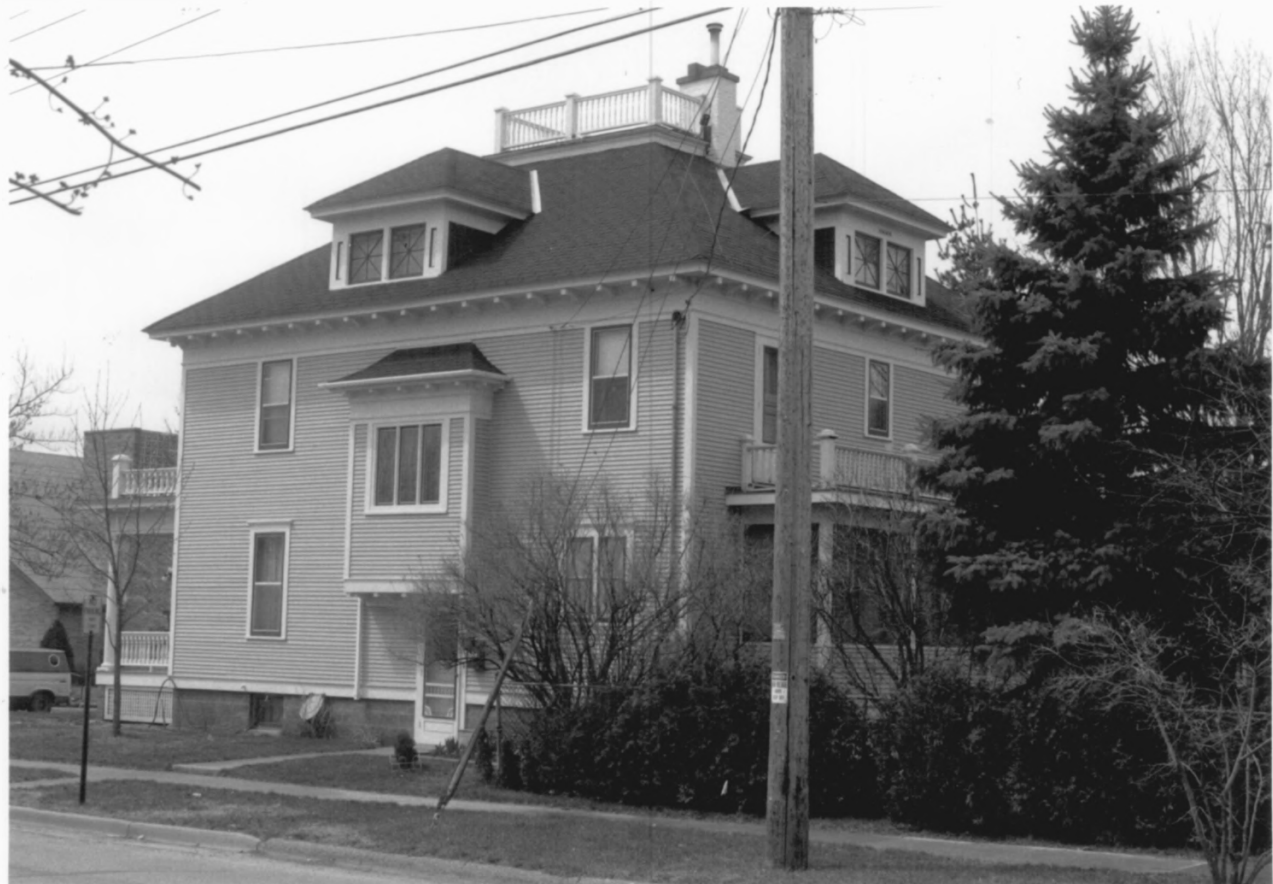
E. Daly House, Wisconsin Rapids, Wood County, Photo #4 of 7 [wca]
