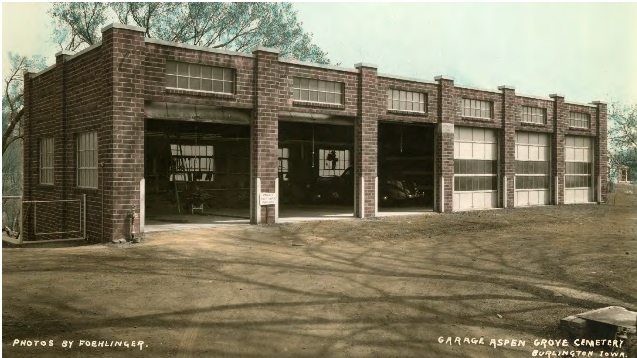
South side view of the service building. Aspen Grove Cemetery photograph collection.
