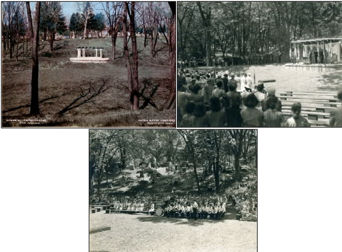
Historical photographs of the platform (top two views showing the pergola then in place) and the seating in the amphitheater that faced the stage platform (bottom).
