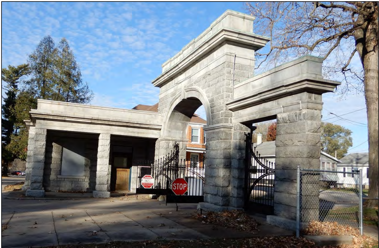
Potter Memorial Building and Gateway at Corse Street, looking NNE. Photograph taken by Tallgrass Archaeology LLC, November 8, 2019.
