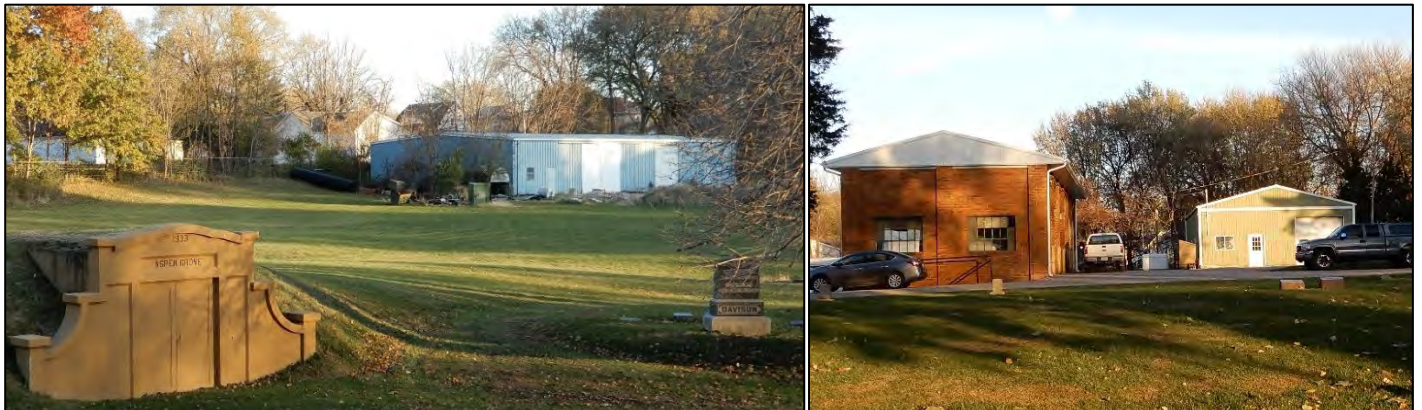
Larger maintenance shed, view from the 1933 receiving vault (left) and the smaller maintenance shed to the right of the 1930s service garage (right). Taken by Tallgrass, November 8, 2019.
