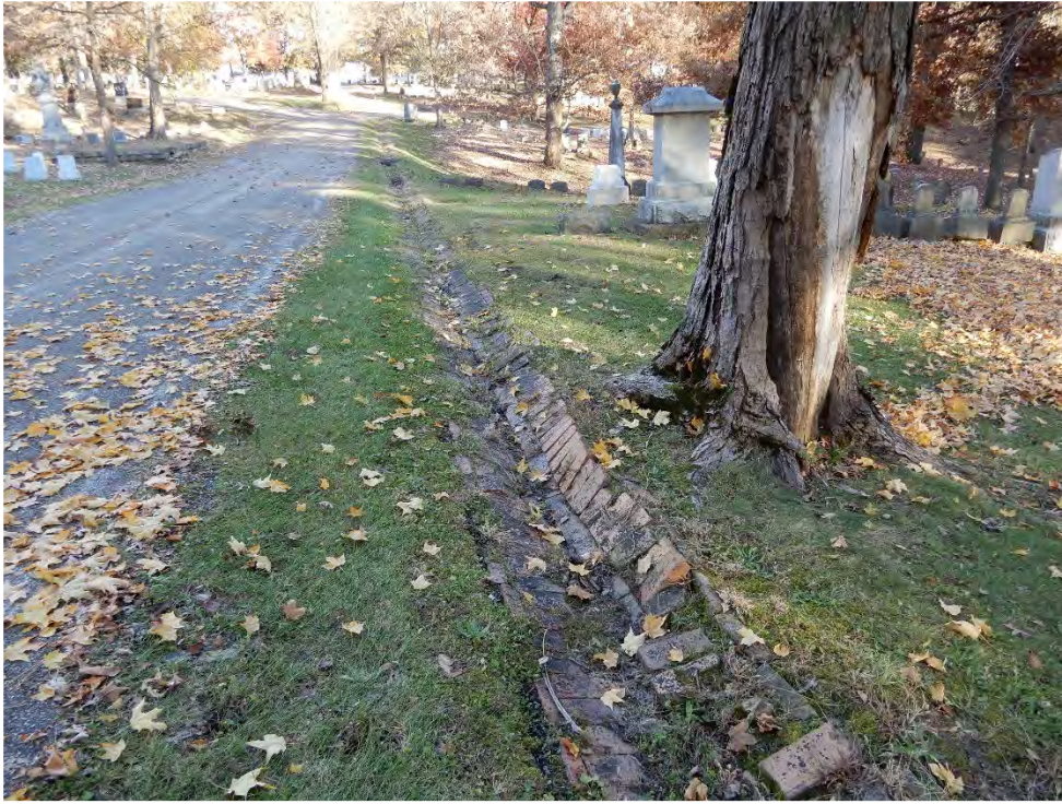
Brick drain in Aspen Grove Cemetery. Taken by Tallgrass, November 8, 2019.
