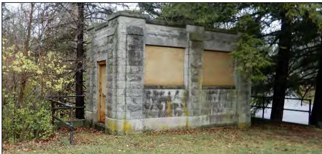
View of former convenience building. Photograph taken by Tallgrass, November 25, 2020.
