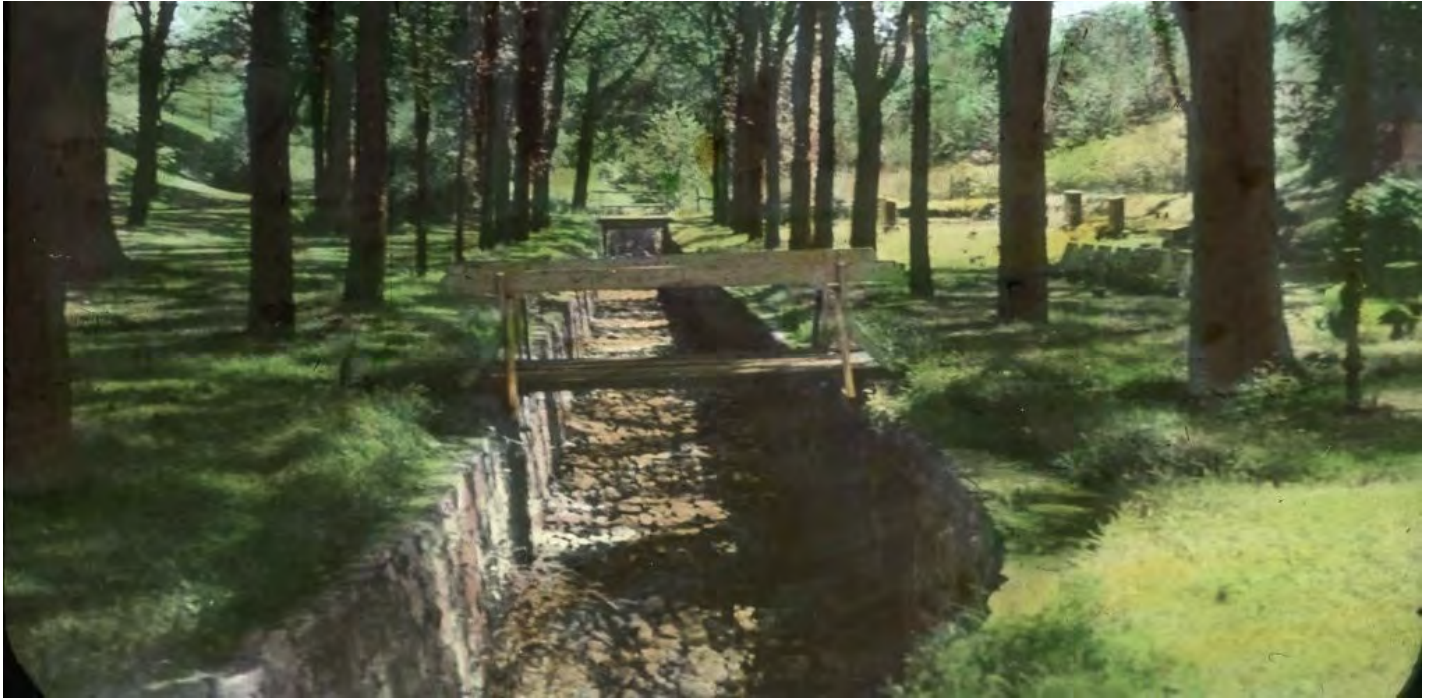
Historical photograph of open section of the stone-lined storm drain.
