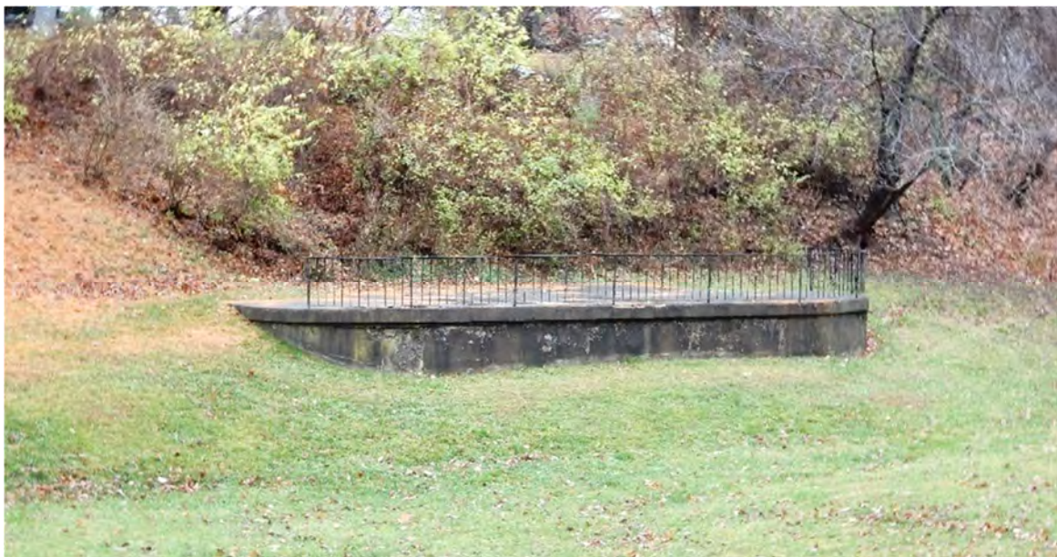
Current view of platform, all that remains of the amphitheater.
