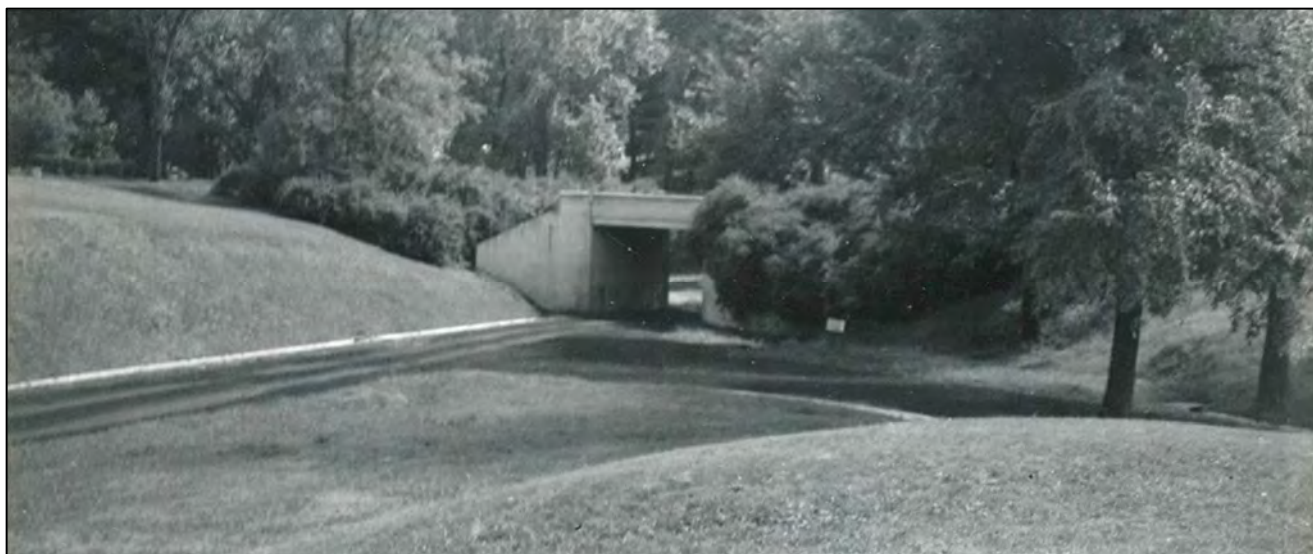
Undated historical photograph of the overpass. Source: Aspen Grove Cemetery photograph collection.
