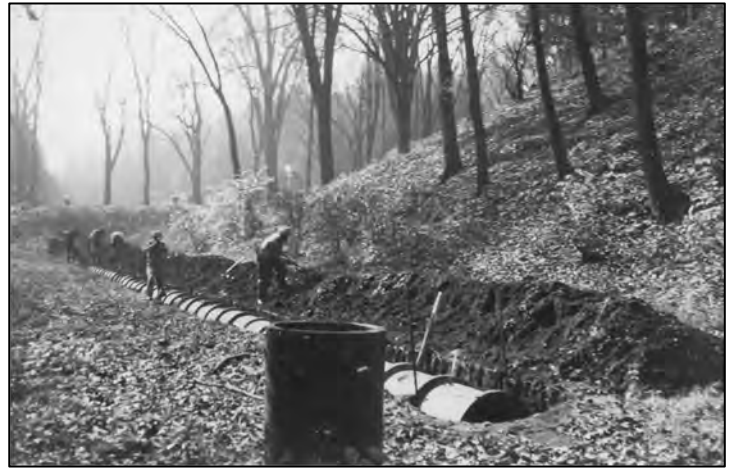
Photographs of workers in the early twentieth century installing underground vitrified pipeline in the ravine. Source: Aspen Grove Cemetery photograph collection.
