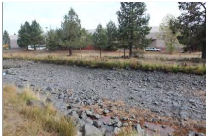
The Fred Meyer Shopping Center at Third Street is on the south side of the Central Oregon Canal. The shallow canal bed is cut on the south side (right) and is bermed on the north side. Looking southeast. 391
