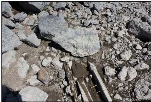
Looking down into the bed of the canal at a crossbeam nearly covered with silt. It is made of three boards, arranged in a box pattern and attached with nails. 61
