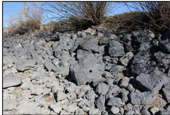
The COCHD displays dozens of 2.25" holes drilled for explosives. 258
