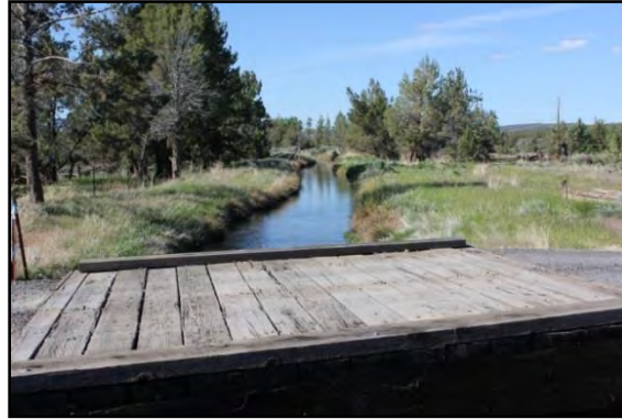
North of the community of Powell Butte, the canal rapidly drops in elevation and is about 13' wide and flows under many wooden bridges for driveways.
