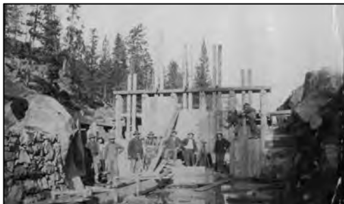
Crew building the shared diversion structure at the Deschutes River for the two canals, ca. 1903. 92
