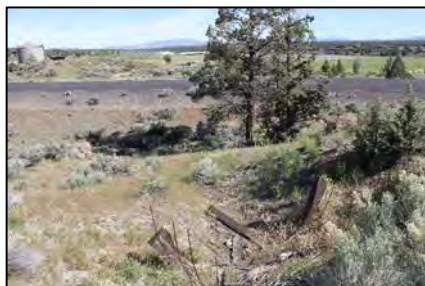
Photo looking southwest from the stilling pond on the east bank of the Dry River, across the site of the Powell Butte Siphon, stave pipe and trestle. Some remains of the historic flume outlet structure are in the foreground. 407
