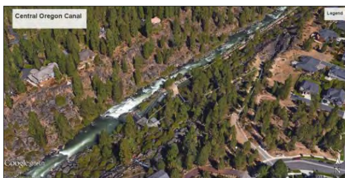
Diversion gate and fish screen at the eastern bank of the Deschutes River and the above-ground pipe conveying water for the Central Oregon Canal, at the southern edge of Bend. 26
