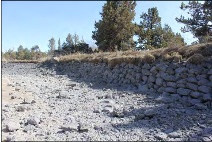
Photo 19 of 20: Carefully stacked rock on steep south side slope, looking east.
