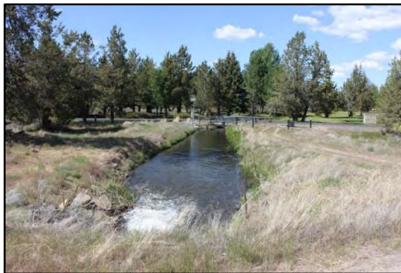
Water flows under the north berm in a metal pipe to the 'B' Lateral, looking north toward Bear Creek Road. 70
