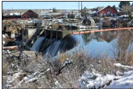
The 1912 North Dam on the Deschutes River, photographer looking east. 251
