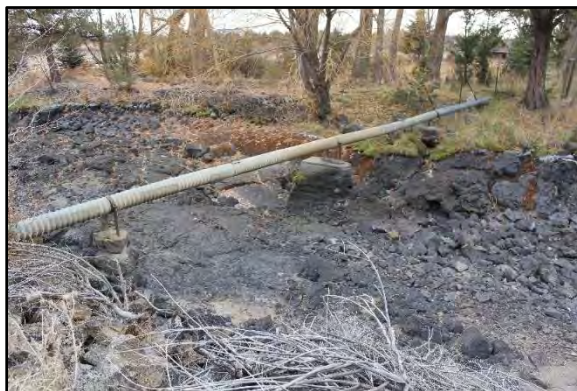
Looking northwest to a metal irrigation water delivery pipe supported on three historic rock piers. 62
