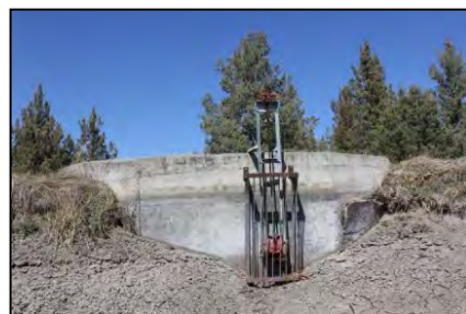
Looking north to a non-historic headgate (Headgate #20 in Table 1) that is caged with reinforcing bars to prevent rocks from clogging it. 80
