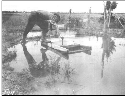
A man works on an evaporation pond and weir next to a lateral and irrigated field on the Central Oregon Canal near Alfalfa 364
