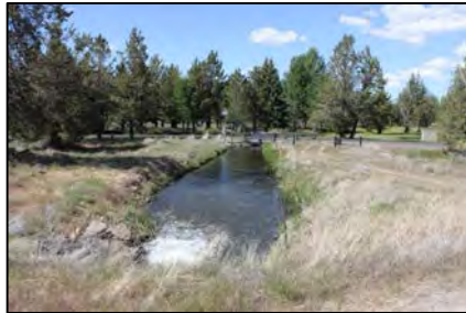
Water flows under the north berm in a metal pipe to the 'B' Lateral, looking north toward Bear Creek Road. 71
