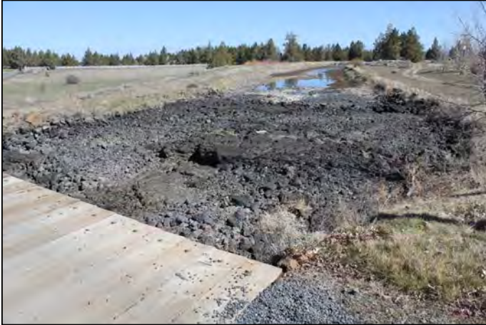
Photo 7 of 20: Looking east from the Bear Creek Ranch Bridge, cut on the south side and berm on north side.
