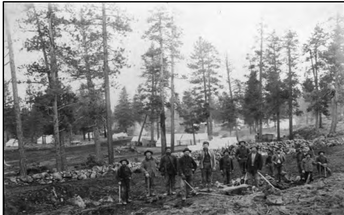
Photo taken in early 1905 of laborers and their tent camp along the Bend stretch of the Central Oregon Canal. 88
