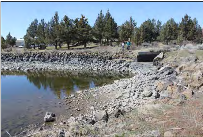
Photo 12 of 20: Looking west into the drop from Burt's Chute into pond.
