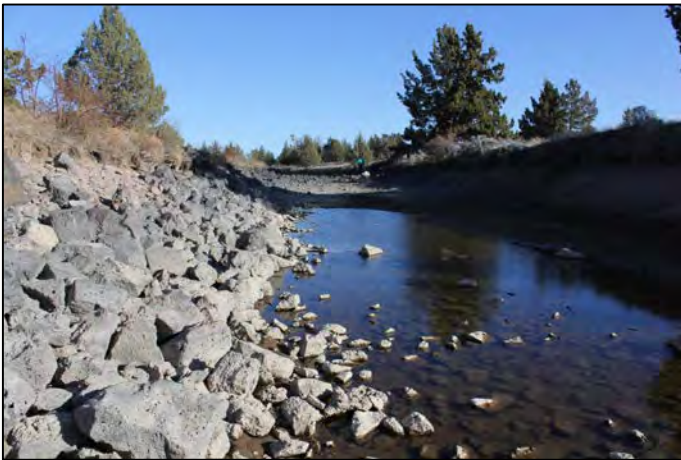
Photo 4 of 20: Looking east with a tall berm with rip-rap on the north side in a deep, narrow portion of the canal that holds water year around.
