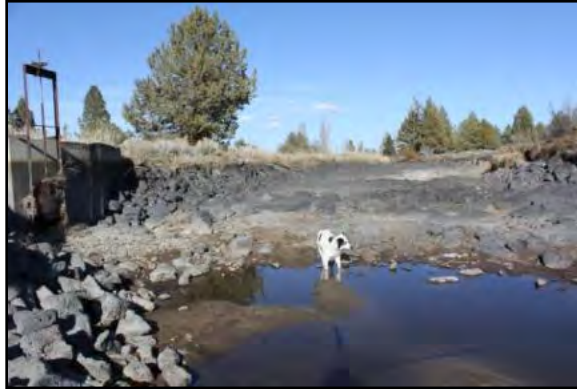
Screw assembly to operate the headgate to the 'B' Lateral looking east. . 69
