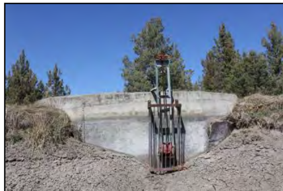
Looking north to a non-historic headgate (Headgate #20 in Table 1) that is caged with reinforcing bars to prevent rocks from clogging it. 79
