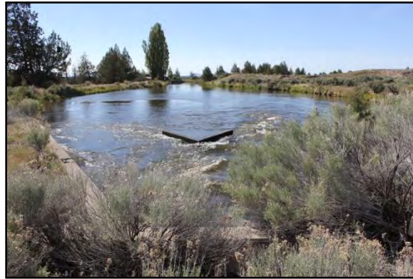
The water forcefully rushes out of the Powell Butte Siphon pipe on the eastern ridge of the Dry River and enters a dispersion pond at elevation 3229 and begins its northerly route toward Powell Butte. Looking north. 403
