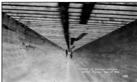
1923 photo of men standing in the enlarged Central Oregon canal flume. 223
