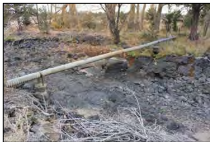
Looking northwest to a metal irrigation water delivery pipe supported on three historic rock piers. 63
