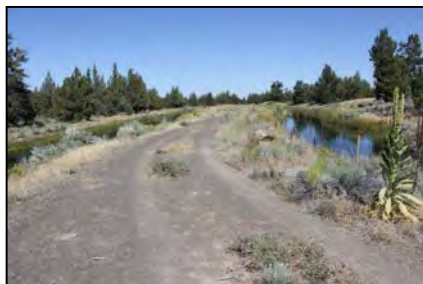
The 'I' Lateral is on the south (right) and the main Central Oregon Canal is on the north, left. Looking east. 400
