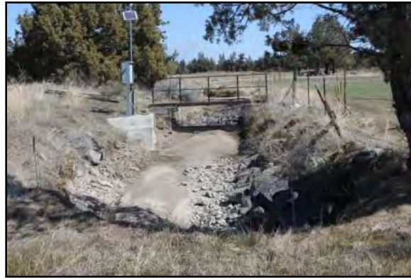
'C' Lateral looking north from the canal is crossed by a pedestrian catwalk. A solar panel is on the pole. 72
