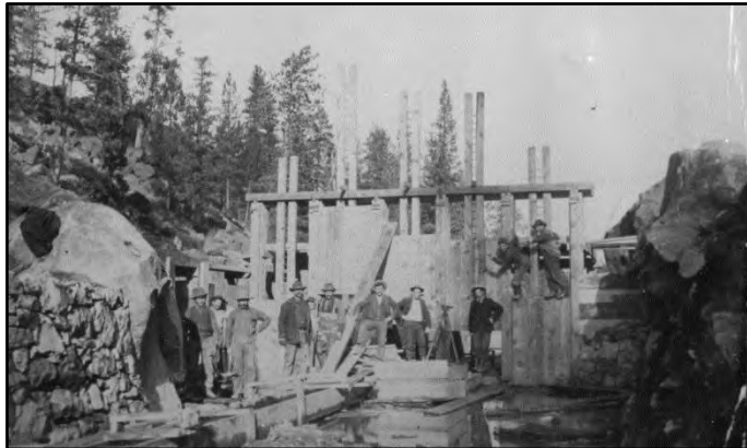
Crew building the shared diversion structure at the Deschutes River for the two canals, ca. 1903. 91
