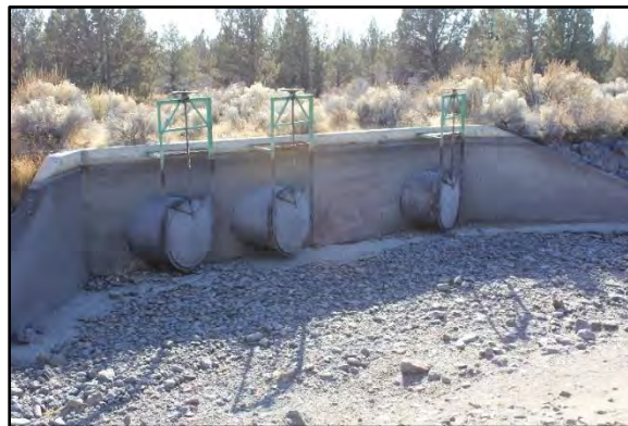
Looking south at Stearns Waste, three headgates and pipes to a reservoir on the south side of canal. 66
