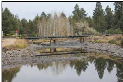
The Union Pacific Railroad tracks cross the canal west of 15 th Street, between the industrial park an urban residential area of southeast Bend. The canal remains wide and shallow with crude, inconsistent rock scattered on the sides and a rocky bed. 393
