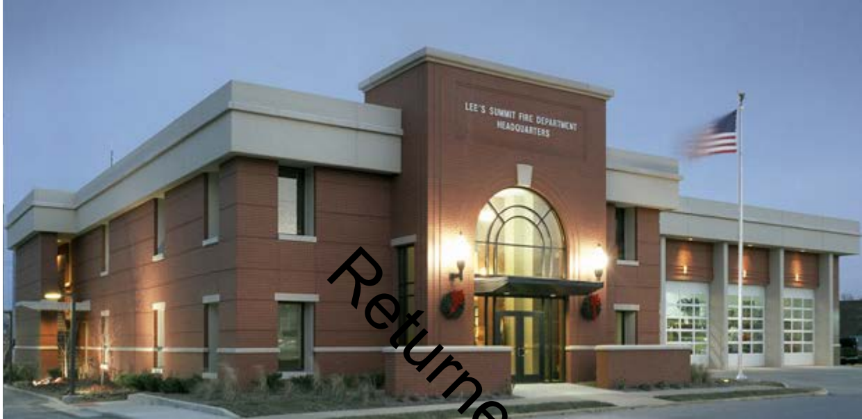
Figure 16. Lee's Summit Downtown Fire Station after renovation. Williams Spurgeon Kuhl & Freshnock Architects, Inc. "Lee's Summit Fire Station Headquarters Renovation." http://www.wskfarch.com/portfolio/18/public-safety/lees-summit-fire-station-headquarters-renovation/ . Accessed May 15, 2017.
