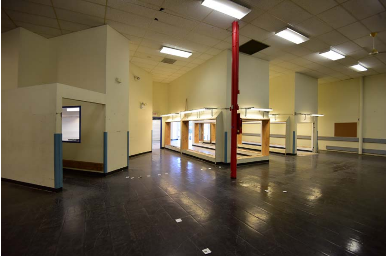
Figure 25. Lee's Summit Post Office. Workroom and post office box walls, view east. F-stop Photography, 2017.
