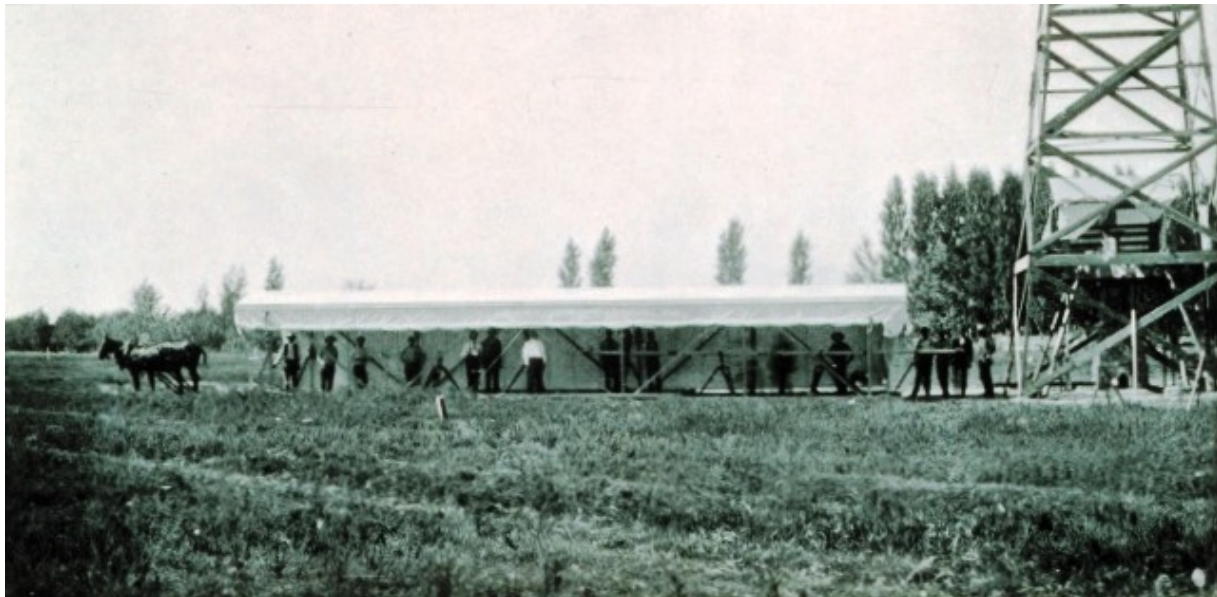
Figure 9. 1893 photograph of the North West Base Monument, scaffolding, crew, Duplex Base Apparatus at the North West Base Monument. View to northwest.
