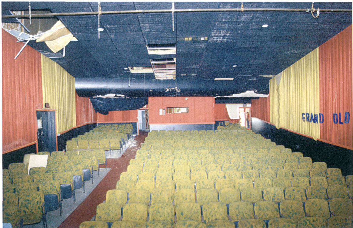
Photo 28 of 44 : View of Room 107, looking towards rear of Auditorium (southwest) from Stage.
