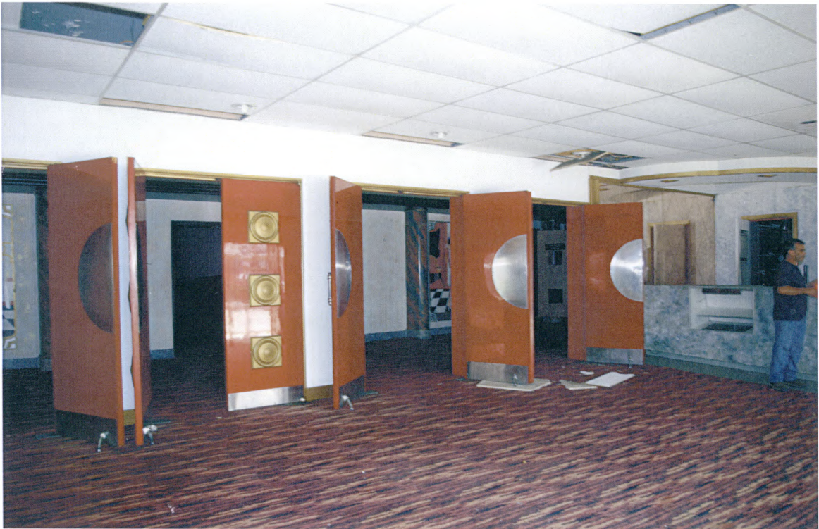
2 Photo 14 of 14: View of Outer Lobby (Room 101) looking east.
