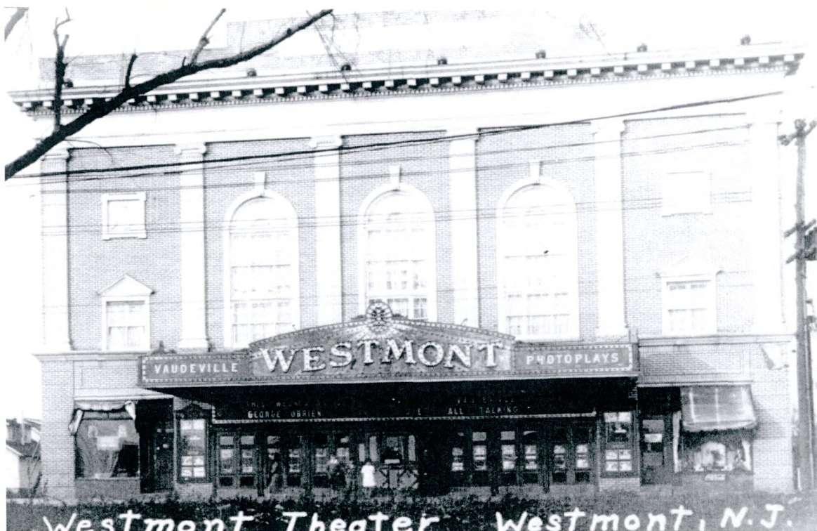
Historic Image 3 of 10: This 1929 photo shows the original door configuration beneath the 1927 marquee. Nearly identical doors survive on the 1927 Ritz Theatre on the White Horse Pike in neighboring Oaklyn (From http://westmonttheatre.wordpress.com/theatre-history/ ).
