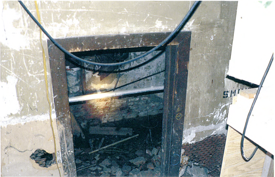
Photo 27 of 44 : View into vaudeville dressing rooms from Stage left (Room 106).
