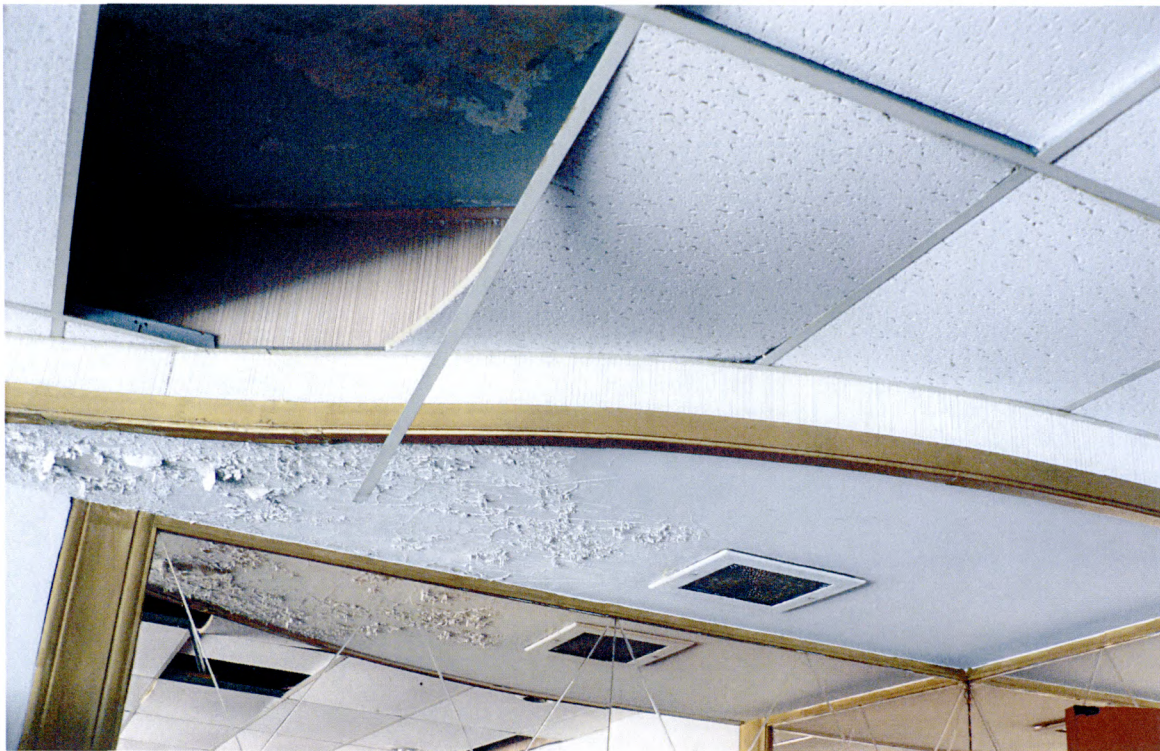
Photo 16 of 14: Ceiling detail in north corner of Outer Lobby (Room 101) showing original plaster ceiling and curving soffit above modern dropped ceiling.
