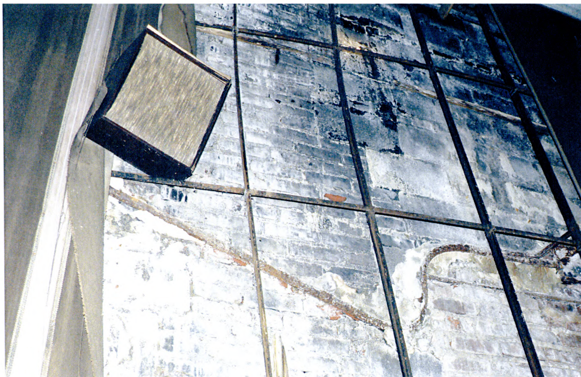
Photo 37 of 41 . Detail of side Balcony wall (looking northwest above Room 105), showing curving ground from decorative plaster work above wood wainscoting.
