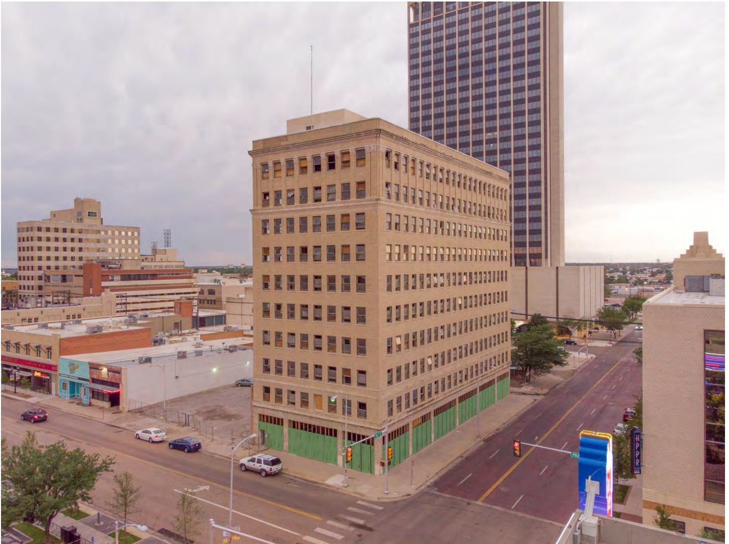
Photo 5: Northeast (primary) oblique. Camera facing southwest.
