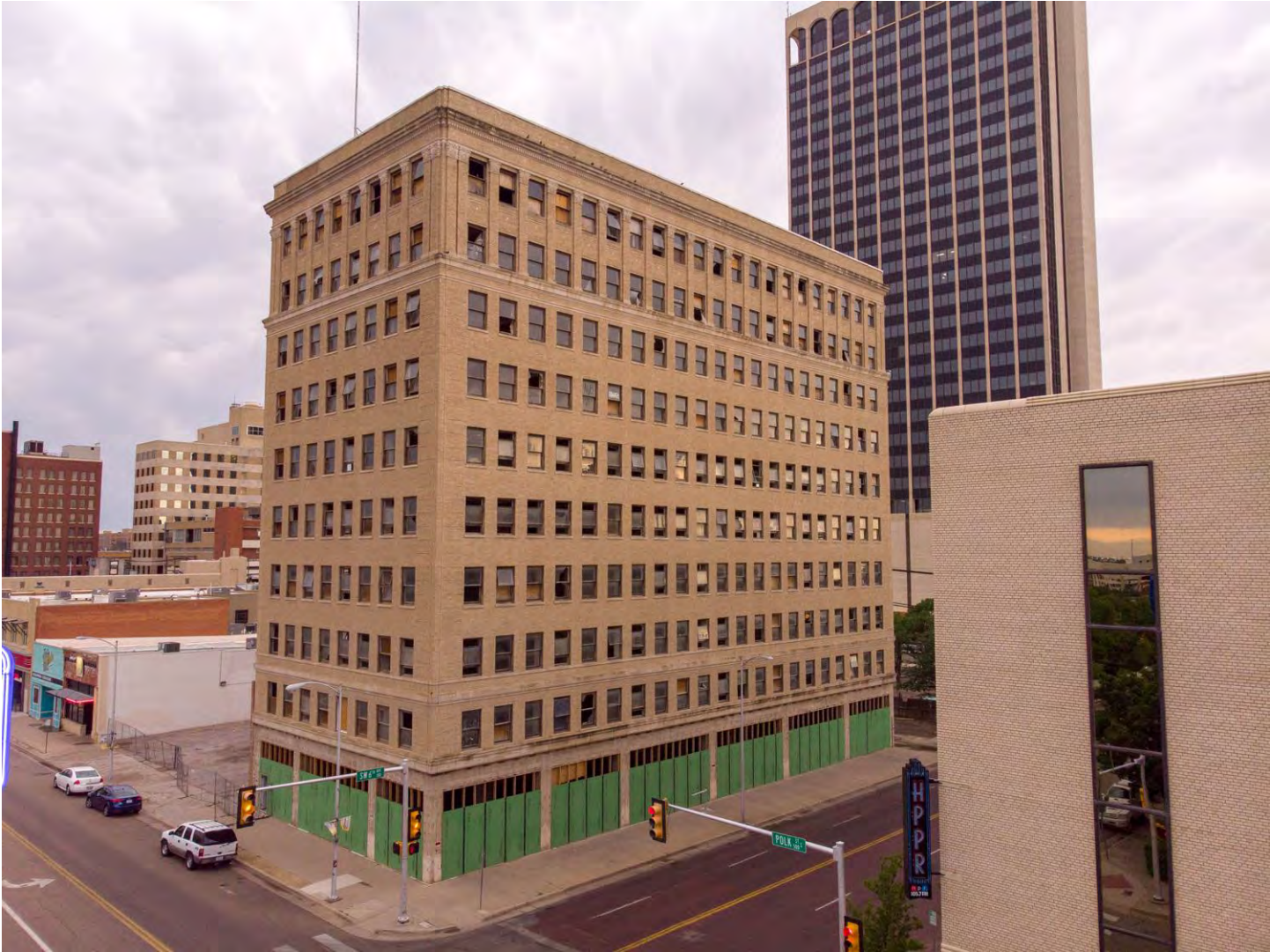
Photo 8: Northeast (primary) oblique. Camera facing southwest.
