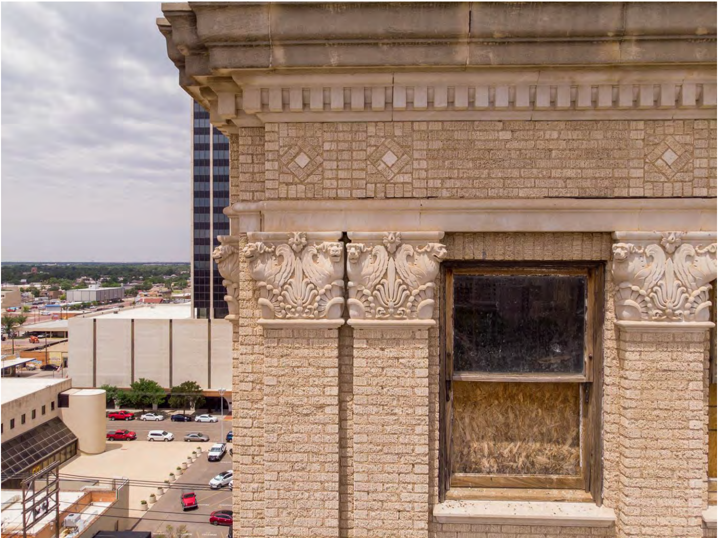
Photo 12: Detail of ornamentation. Camera facing west.
