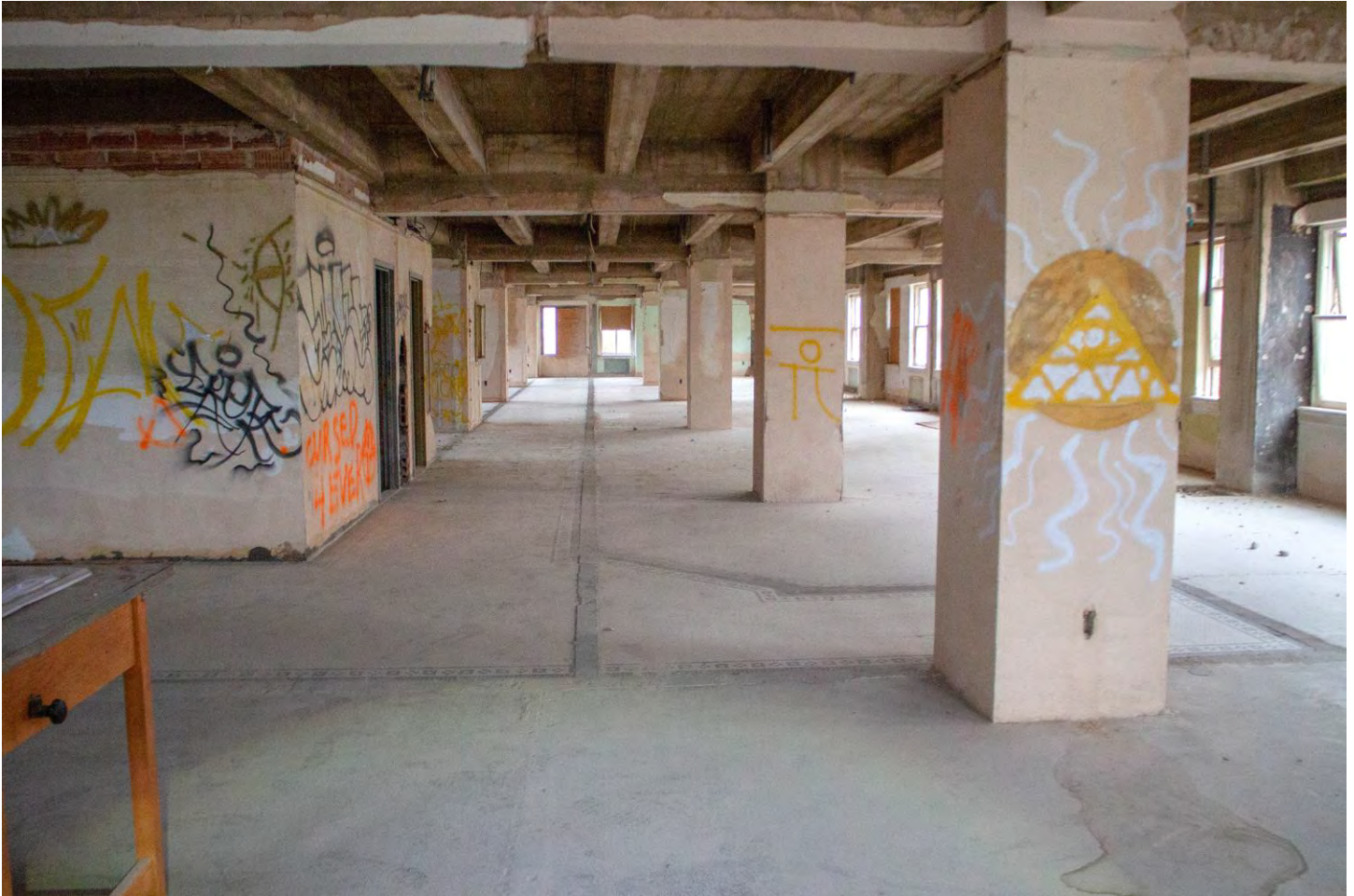
Photo 19: Second floor general view. Camera facing west.
