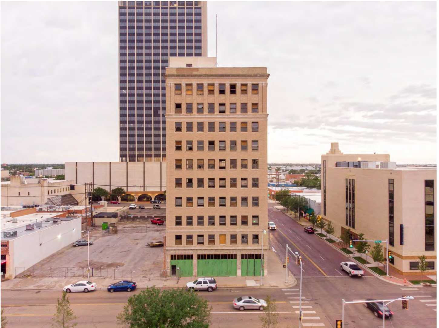
Photo 7: East (primary) elevation. Camera facing west.
