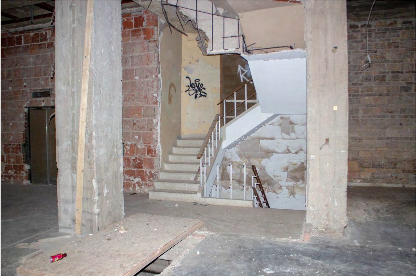
Photo 17: First floor primary lobby stair. Camera facing southeast.
