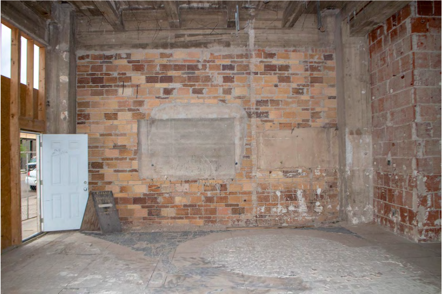
Photo 16: First floor lobby. Camera facing south.
