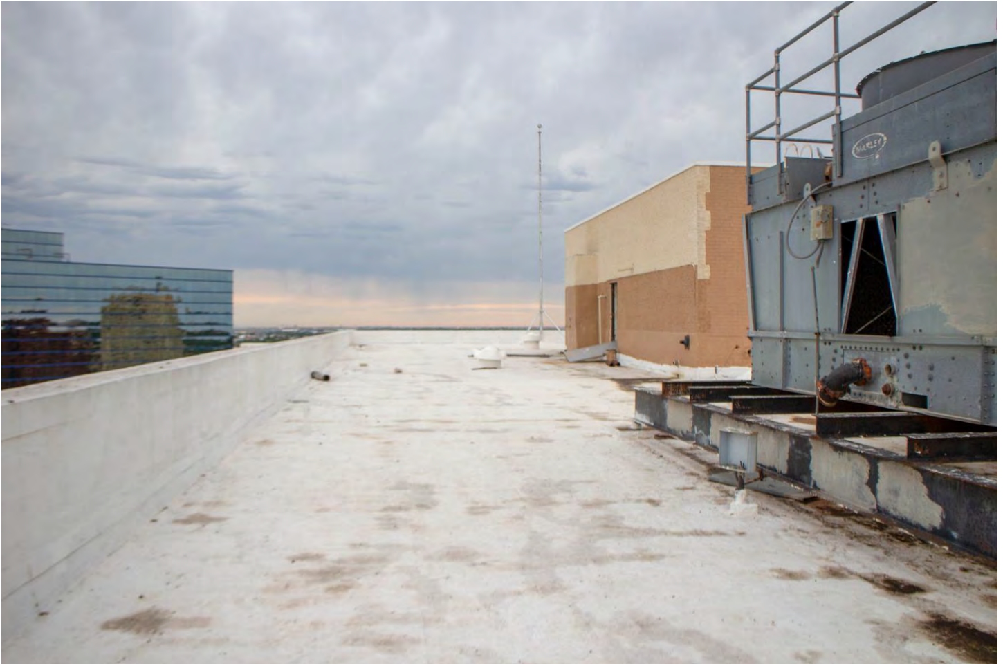
Photo 29: General view of roof. Camera facing west.
