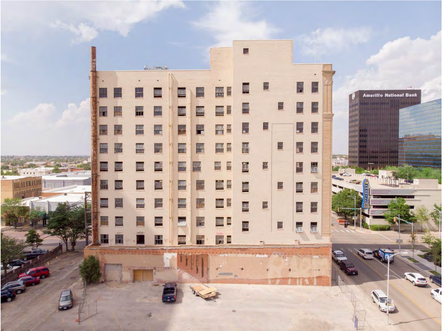
Photo 10: South elevation. Camera facing north.
