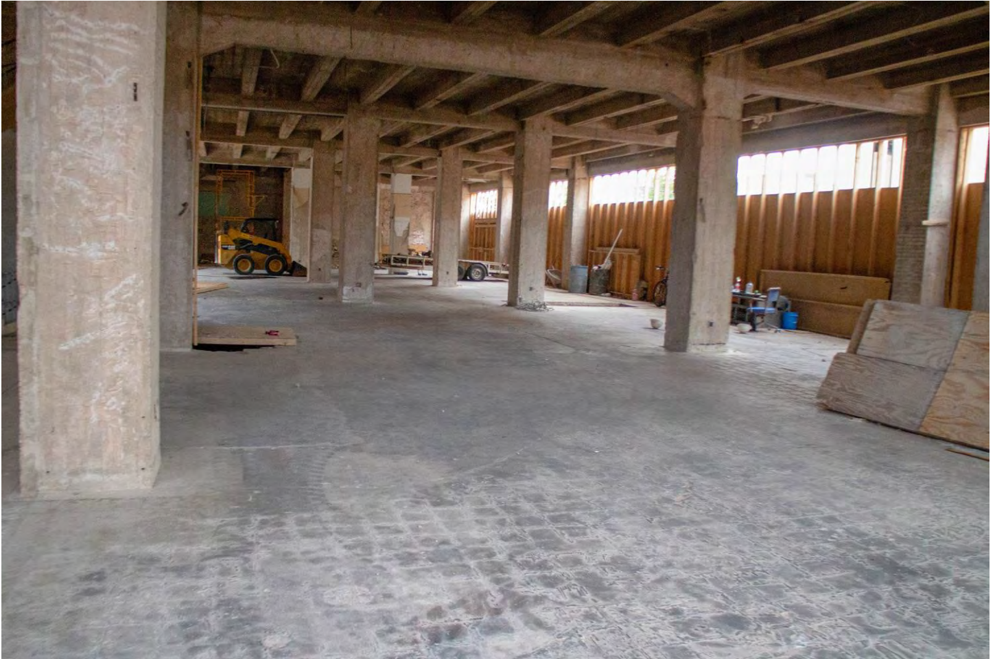
Photo 15: General view of first floor. Camera facing west.
