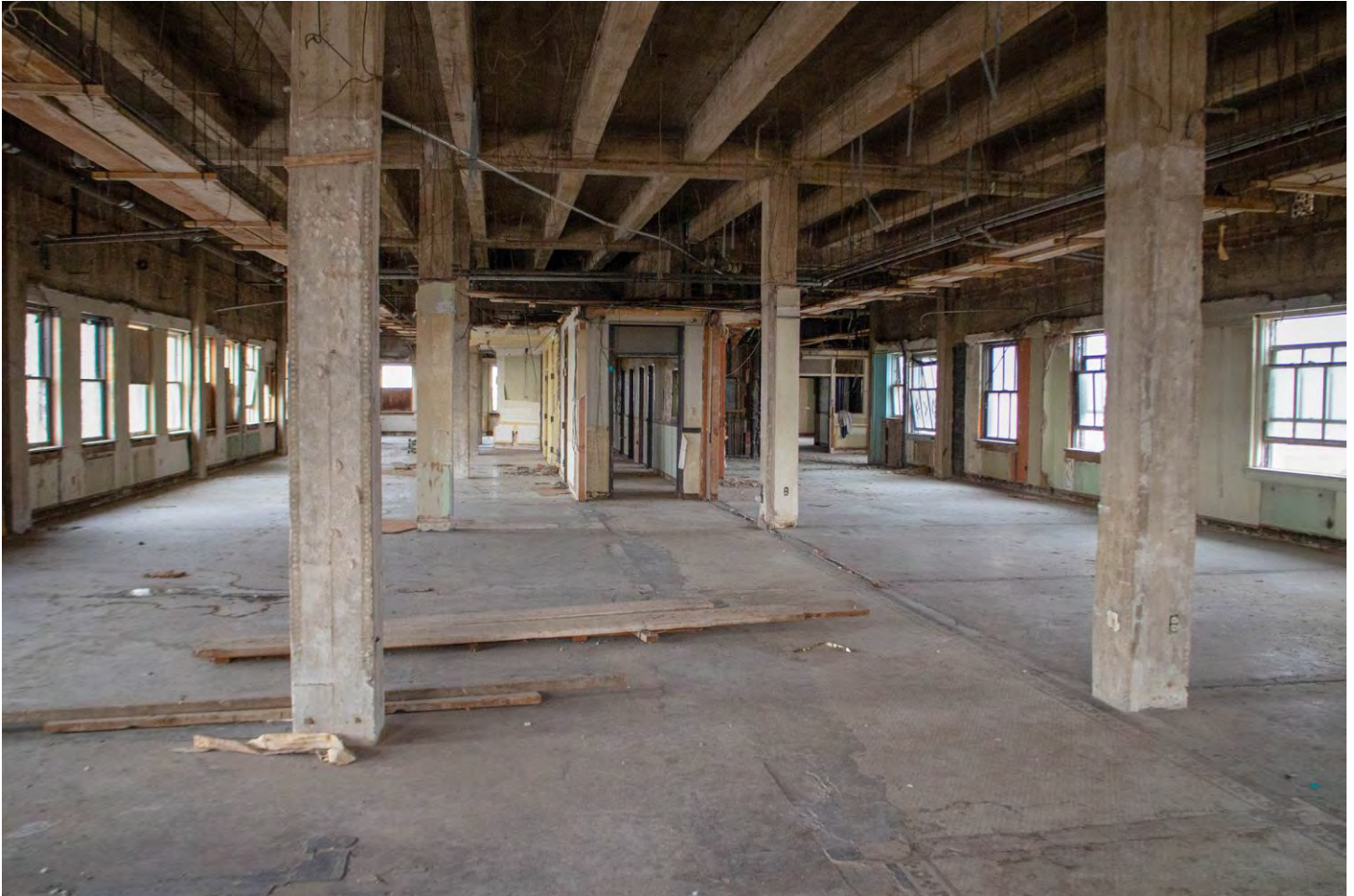
Photo 26: Tenth floor with fragment of original corridor. Camera facing east.
