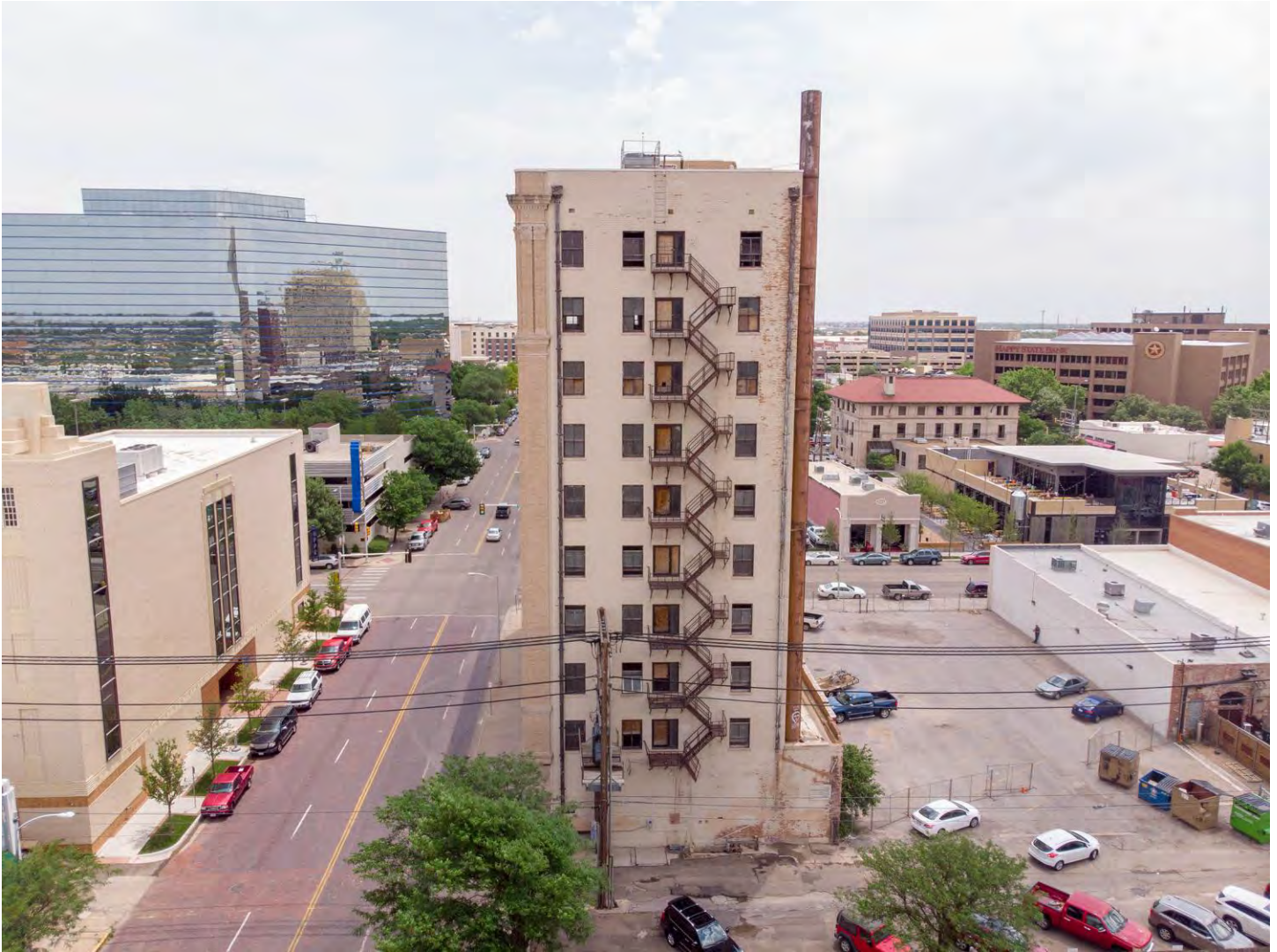
Photo 9: West (rear) elevation. Camera facing east.
