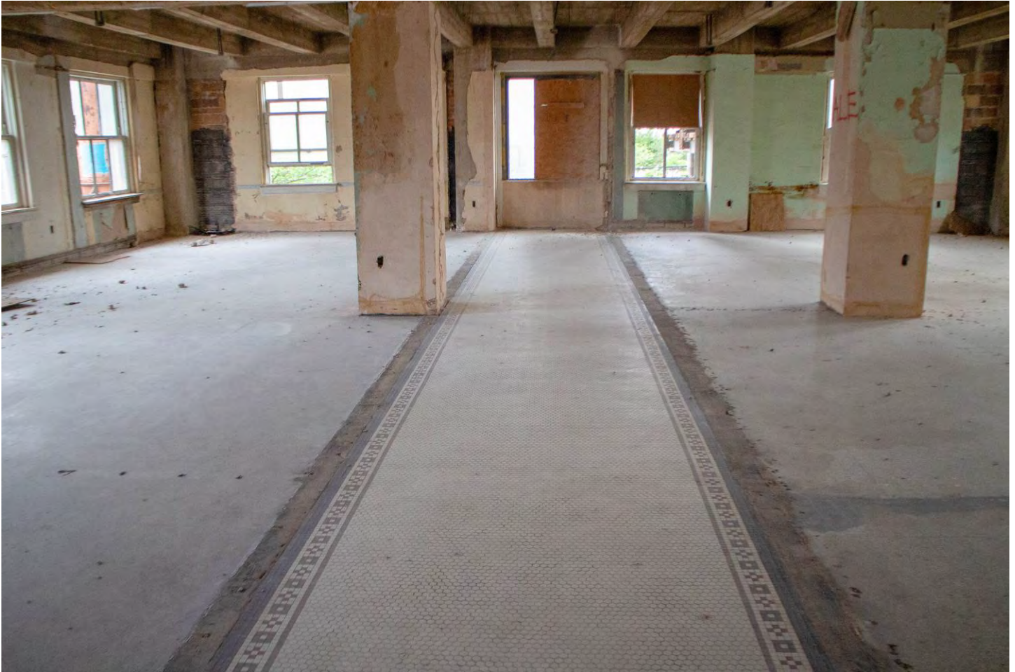
Photo 20: Second floor detail of mosaic tile floor and terrazzo. Camera facing west.
