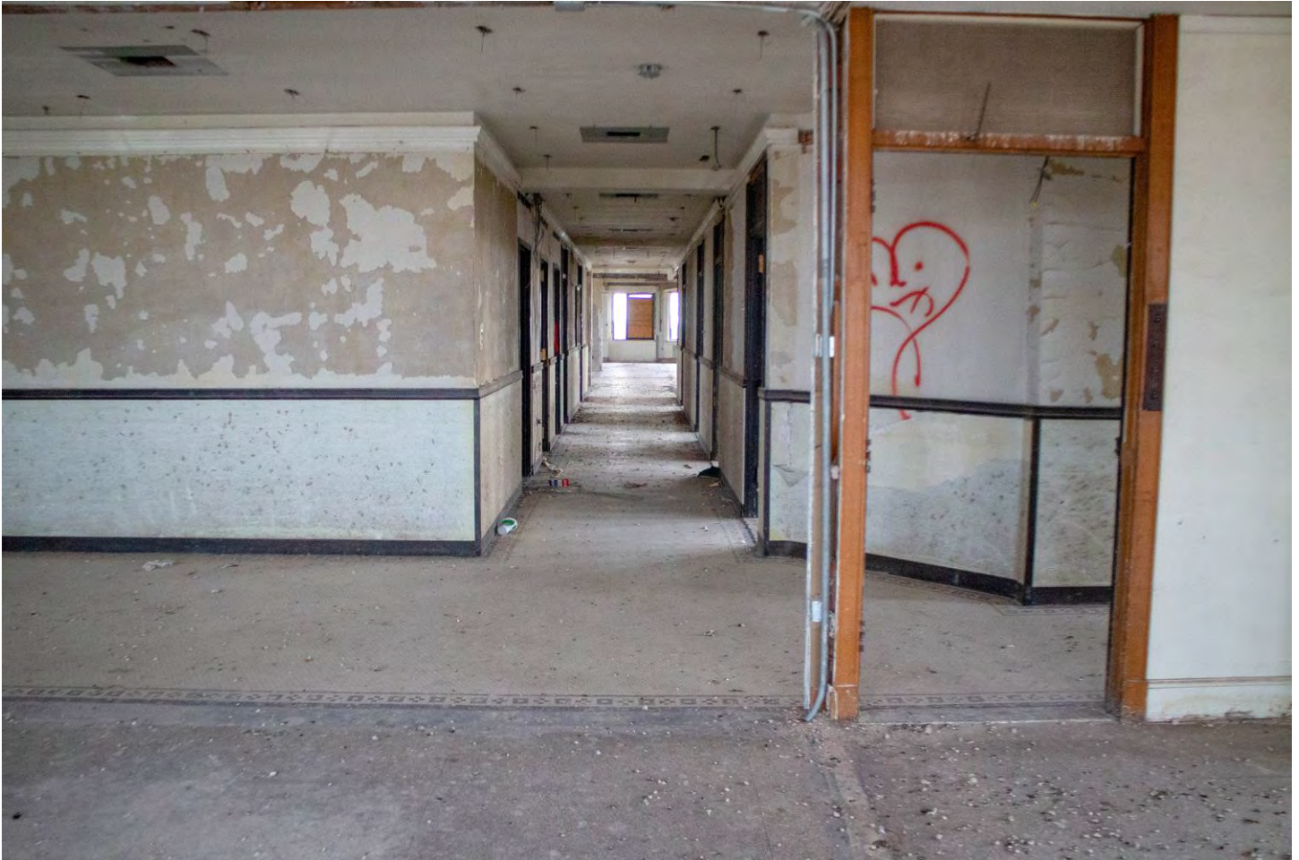
Photo 25: Ninth floor with fragment of original corridor. Camera facing west.
