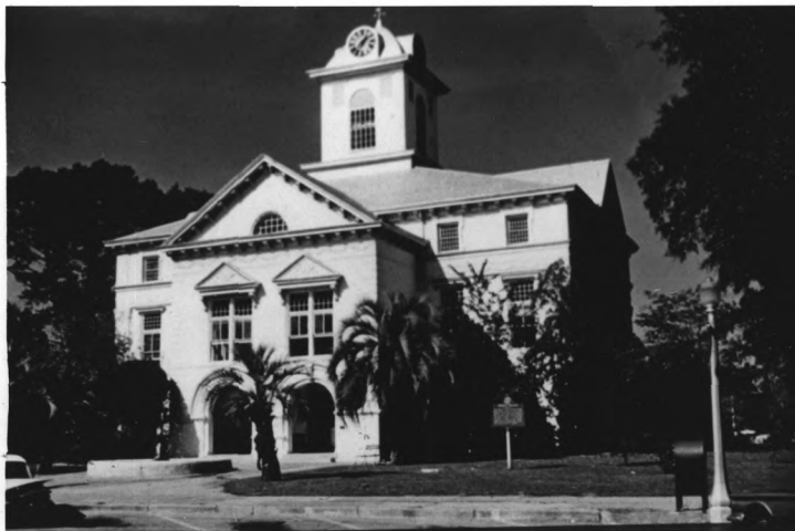
BROOKS COUNTY COURTHOUSE
