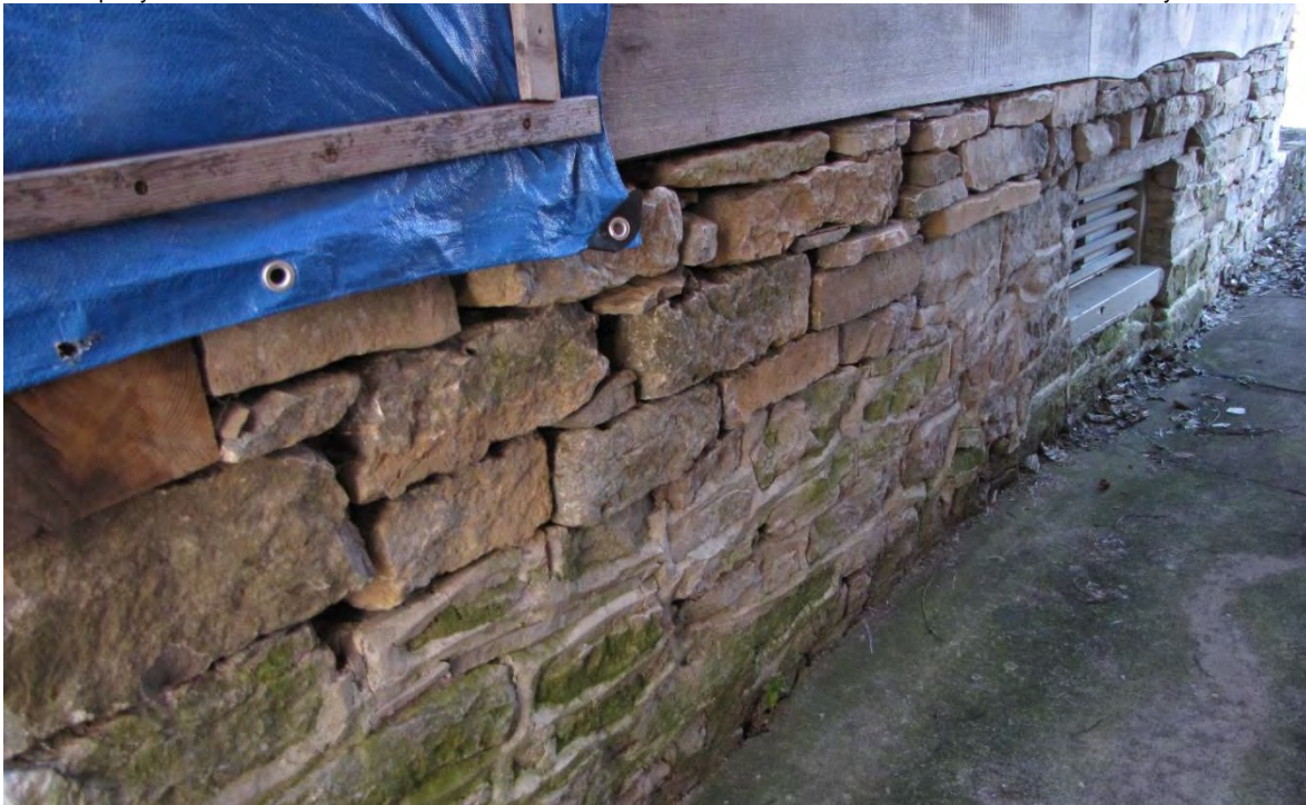
Foundation including recent repairs using dry stone technique.
