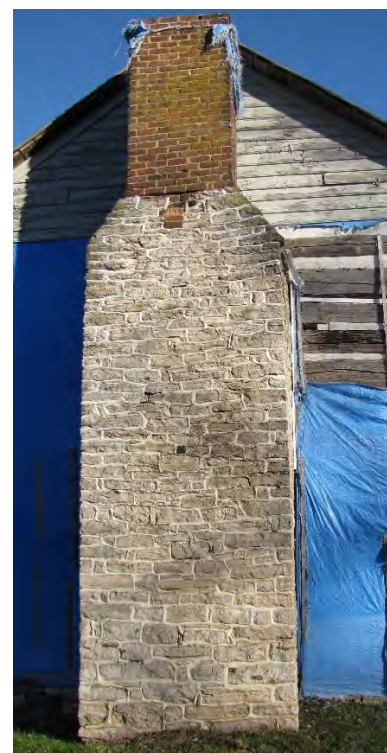
Chimney (west side).
