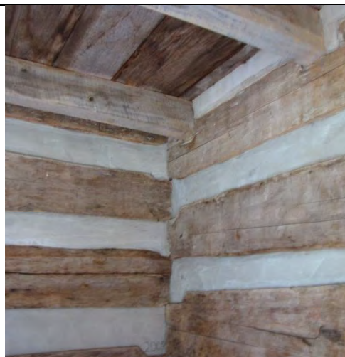
Corner notching on restored log house in Forkland.
