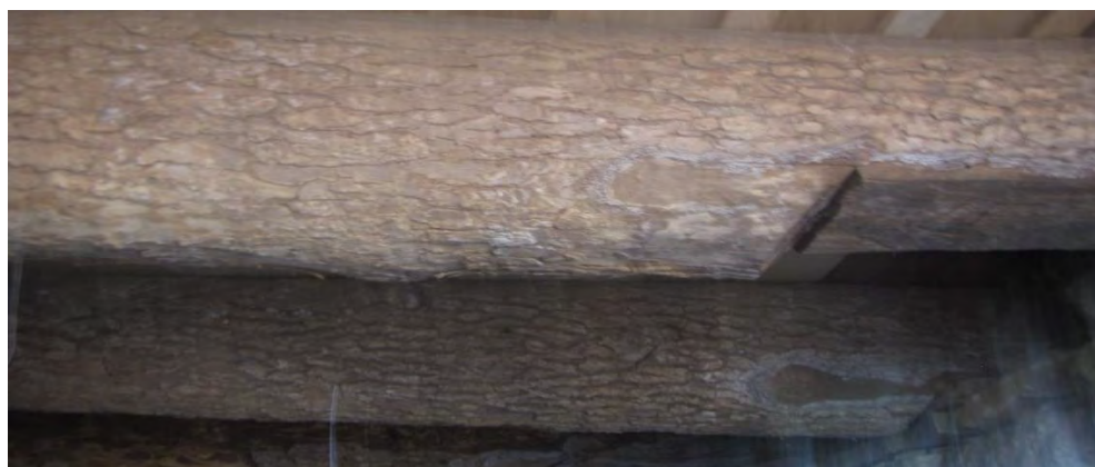
Floor joists as seen from the basement.
