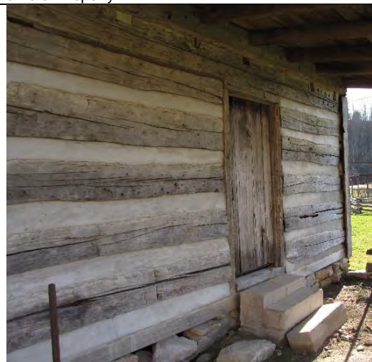
Restored log house in Forkland, with uniform gaps between logs.
