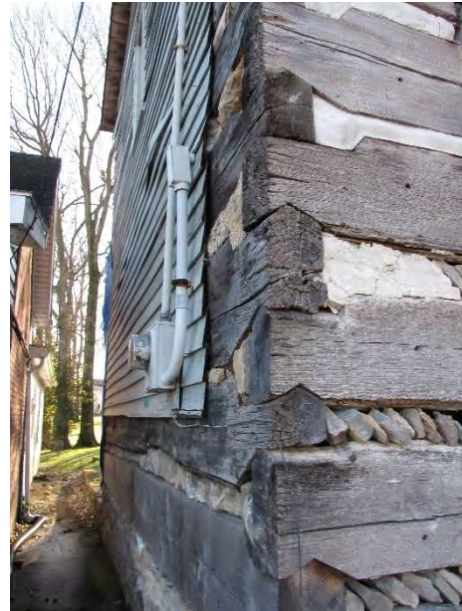
Northeast corner, showing notching
