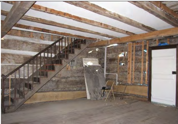
Downstairs, the rear door at right.
