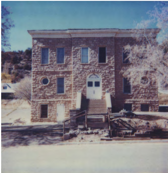
HP6. The Animas City School/ Animas Museum in 1987 with the flat roof. Camera looking west
