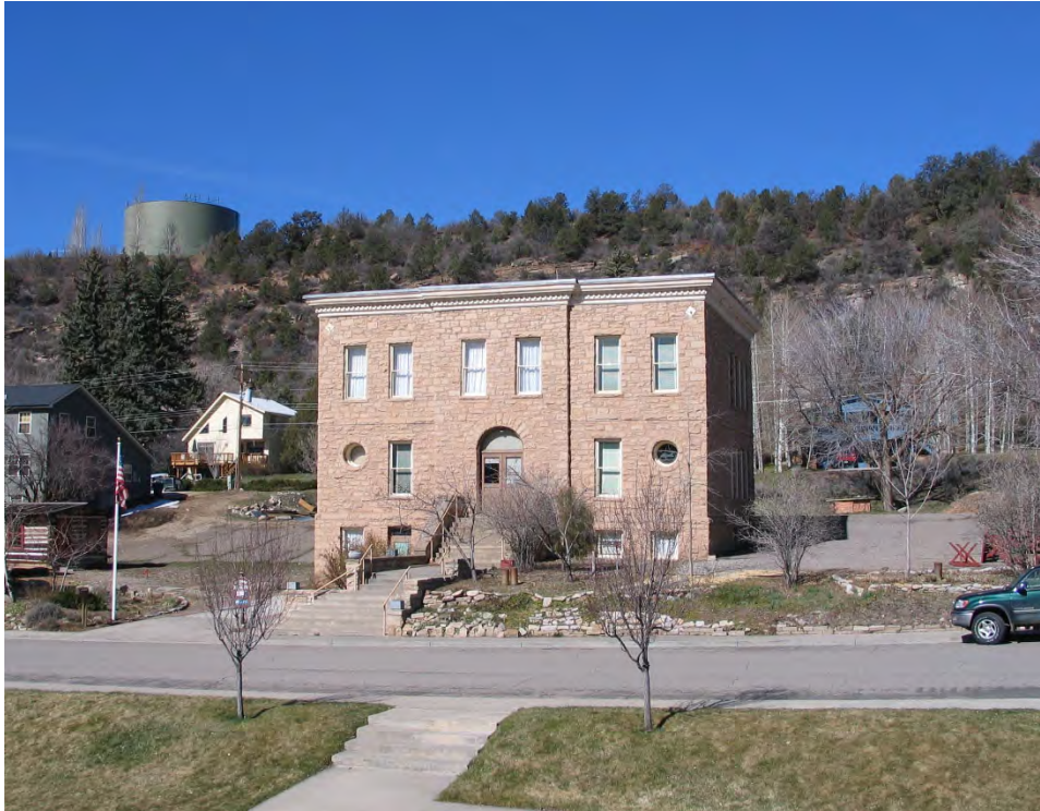
HP7. The Animas City School/ Animas Museum in 2004 with the flat roof. Camera looking west
