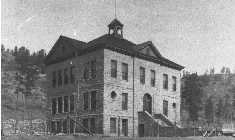
HP1. The Animas City School between 1905 and 1919 before the 1919 fire. Camera looking northwest.
