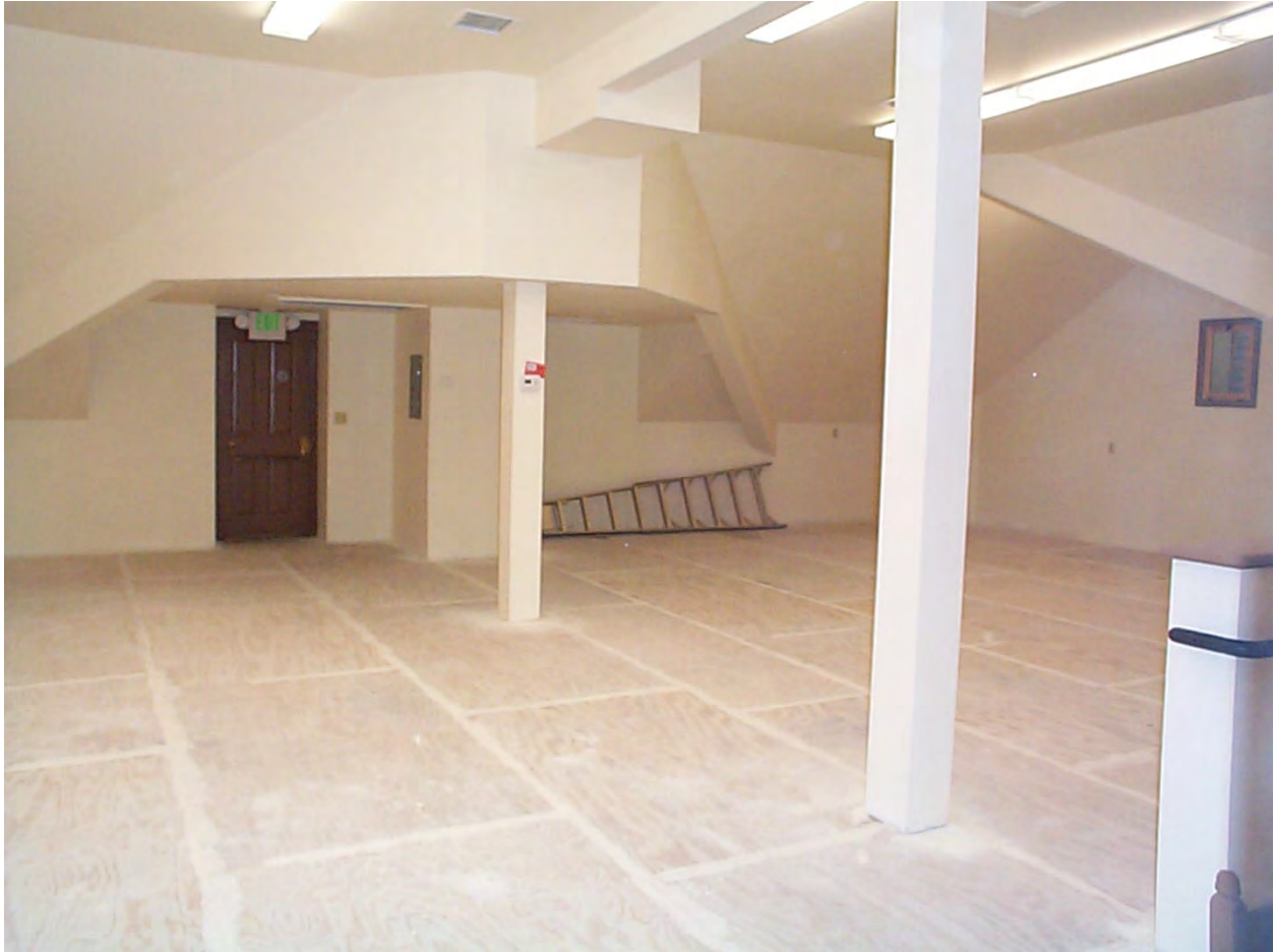
HP9. The Animas City School/ Animas Museum in 2008 inside the reconstructed roof/new Collections area. Camera looking northwest.
