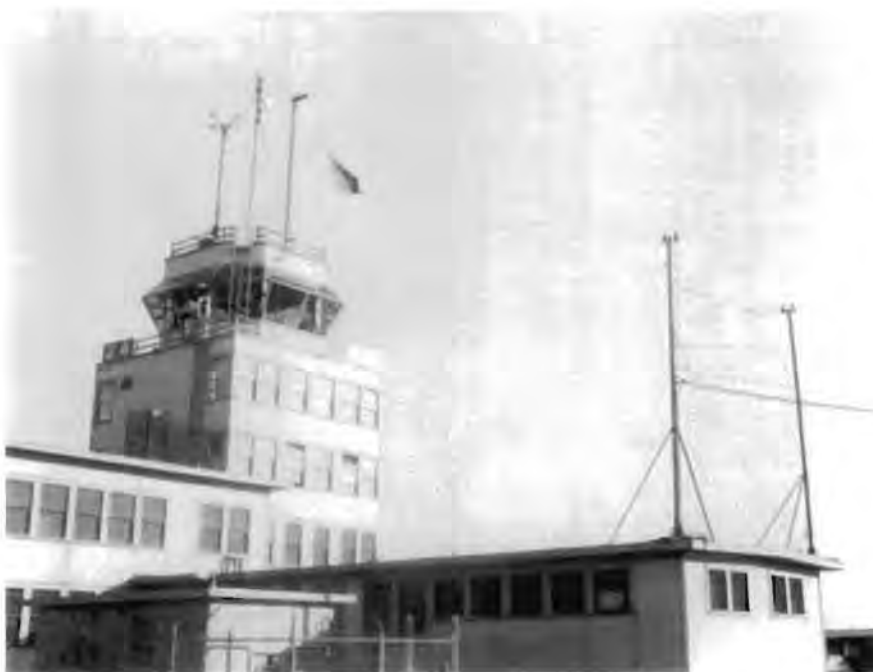
Figure 2: close-up photograph of the control tower with the sewage pump house shown in the foreground. Ca. 1946? View northeast.
