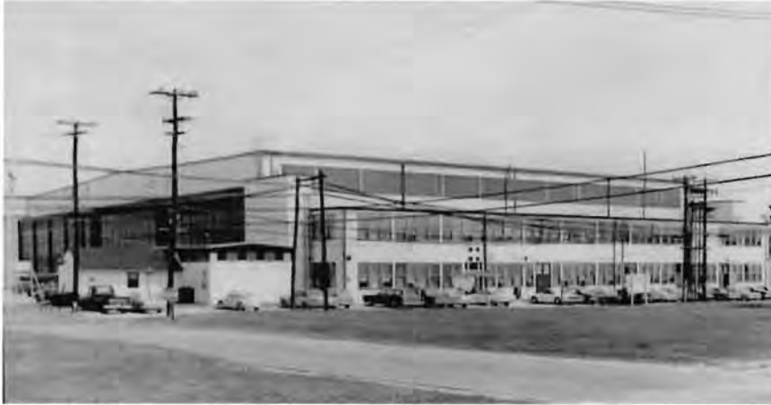
Figure 10 (left): Hangar at Naval Air Station Atlantic City, ca. 1960. This structure shows the similarity in hangar design with those at USNASW.
