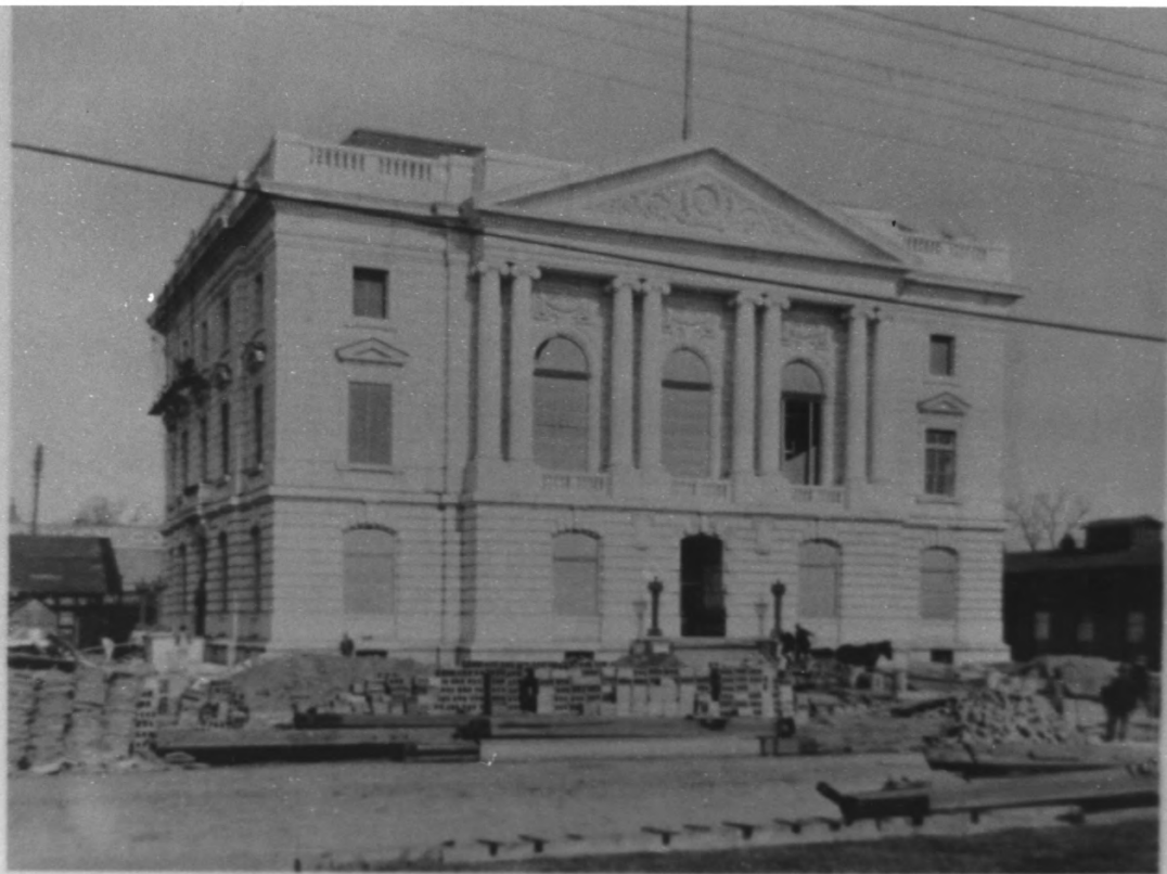
GOVERNMENT BUILDING (Under Construction).
