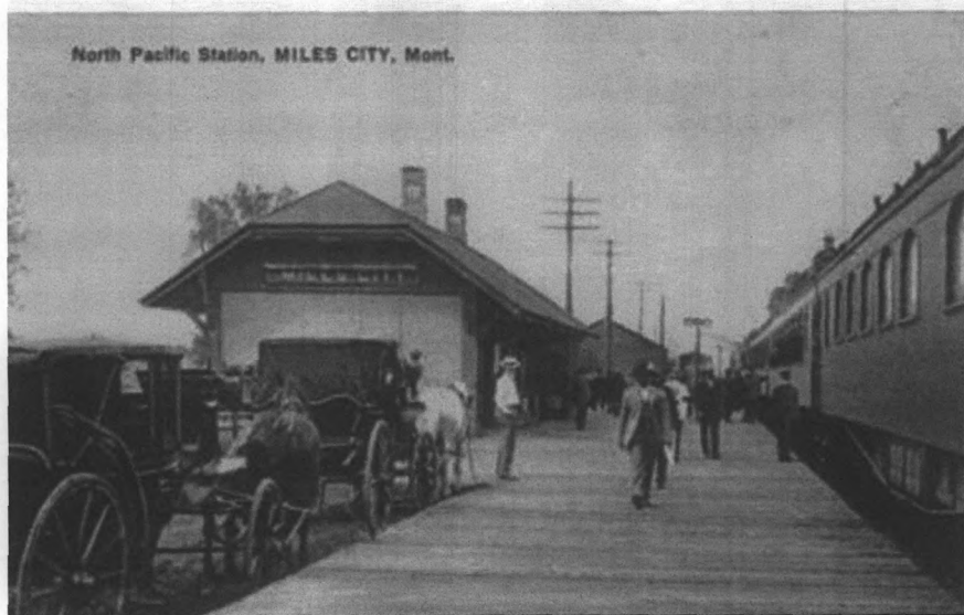
Historic postcard showing c. 1883 depot, view to north-northeast.
