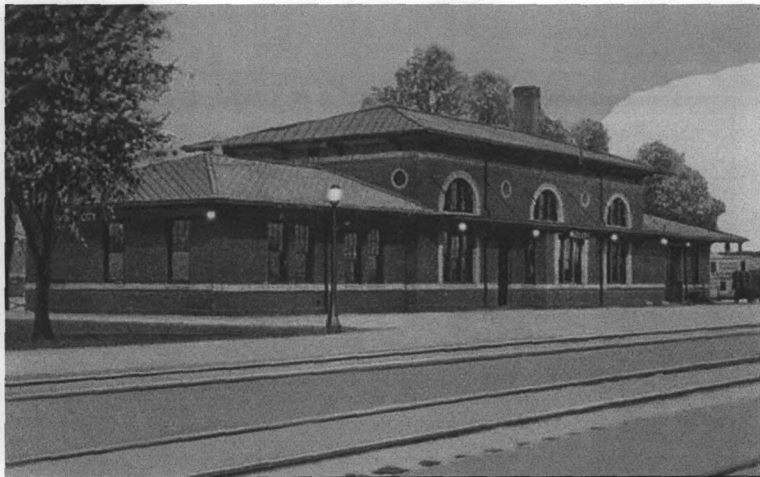
Undated postcard showing east elevation (track side) of the Miles City Depot.
