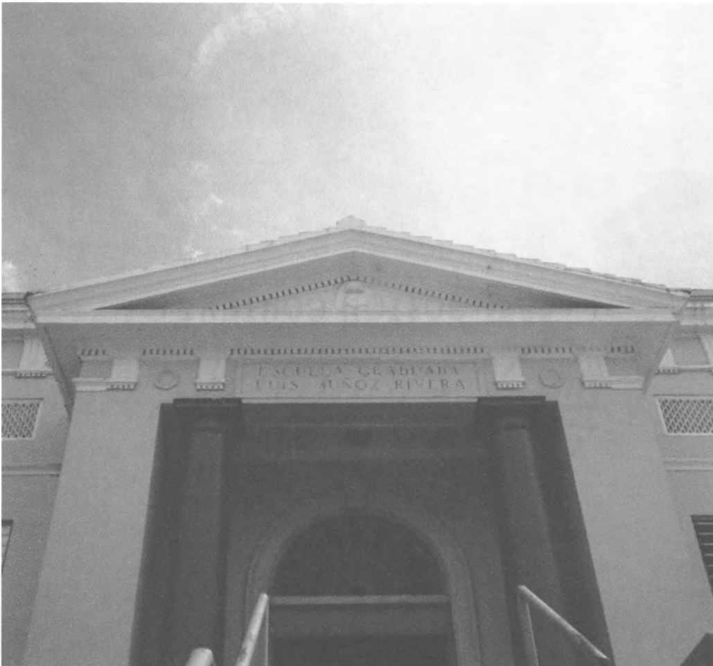
FIG. 5: Luis Muñoz Rivera School west elevation, looking northeast - portico detail, in Lajas Puerto Rico. The porch displays Greek revival features. Next to the columns, solid, plain piers support the entablature on which two pairs of triglyphs appear in frieze-like manner. The continuity of the frieze is interrupted by the school's name at what architects refer to as a table : Escuela Graduada Luis Muñoz Rivera , engraved in bas-relief manner, at center. Left and right of the triglyphs at each end of the front portico, a molding/cornice starts its run north/south along the rest of the façade. Symmetry is further underlined by the subtle placement of raised circular panel medallions placed above, left and right, of each Tuscan column. Photo: Eduardo Miranda, October 24, 2012. Source: Jorge Rigau Arquitectos, San Juan Puerto Rico.
