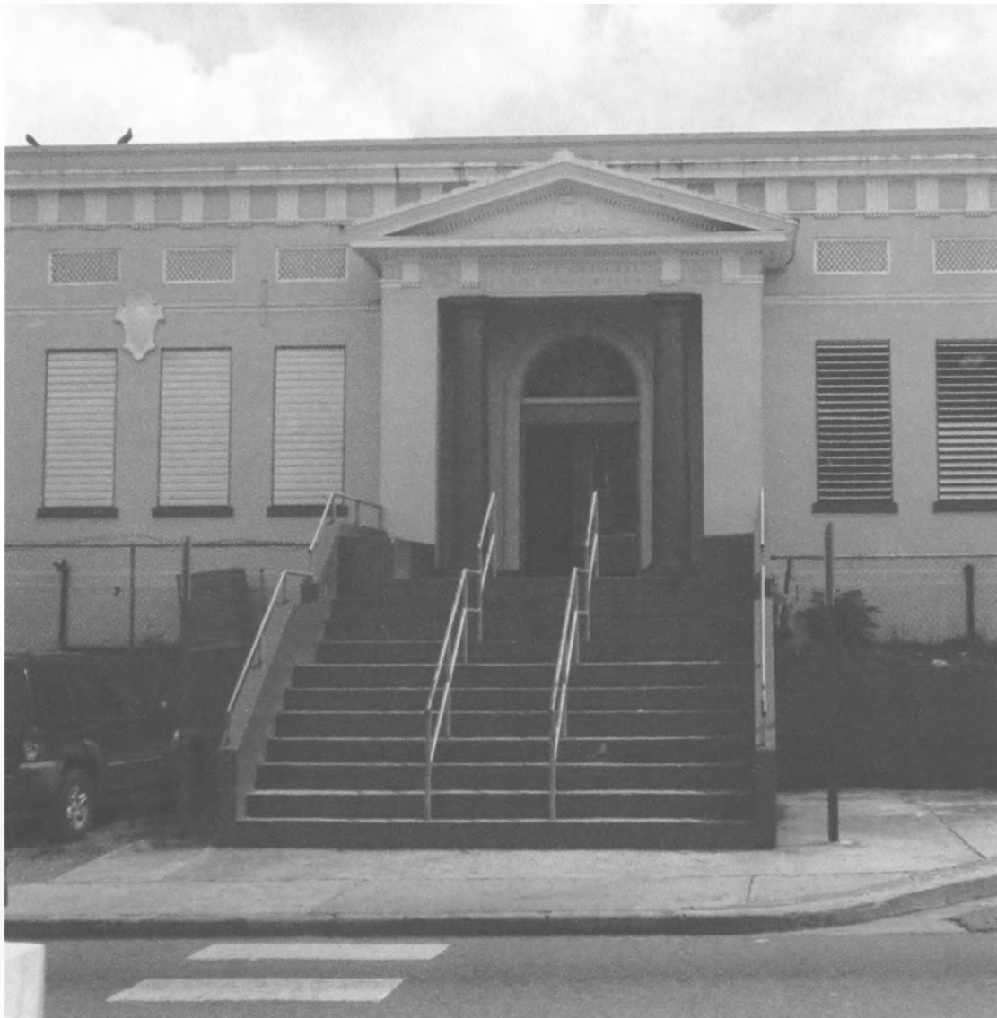
FIG. 3: Luis Muñoz Rivera School west elevation, looking east, in Lajas Puerto Rico. An open-air, straight-run staircase built in reinforced concrete reaches the building itself. Fourteen feet wide, the stair's run is articulated into two flights with a landing in between. Photo: Eduardo Miranda, October 24, 2012. Source: Jorge Rigau Arquitectos, San Juan Puerto Rico.
