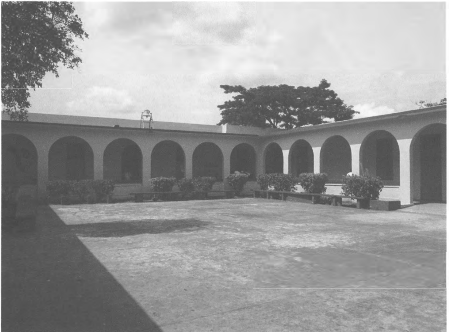
FIG. 7: Luis Muñoz Rivera School east interior elevation, looking west – U-shaped patio, in Lajas Puerto Rico. The open space provides corridors and classrooms with natural light and ventilation. From the court, trees and other school buildings are visible. Around the perimeter of this concrete paved patio, seven long benches, five 2'-0" long planting strips and the arcaded corridors become key transition elements between the school's exterior and interior spaces. The wrap around arcade comprises 24 Roman arches. Six face west, nine to the north and another nine face south. Photo: Eduardo Miranda, October 24, 2012. Source: Jorge Rigau Arquitectos, San Juan Puerto Rico.
