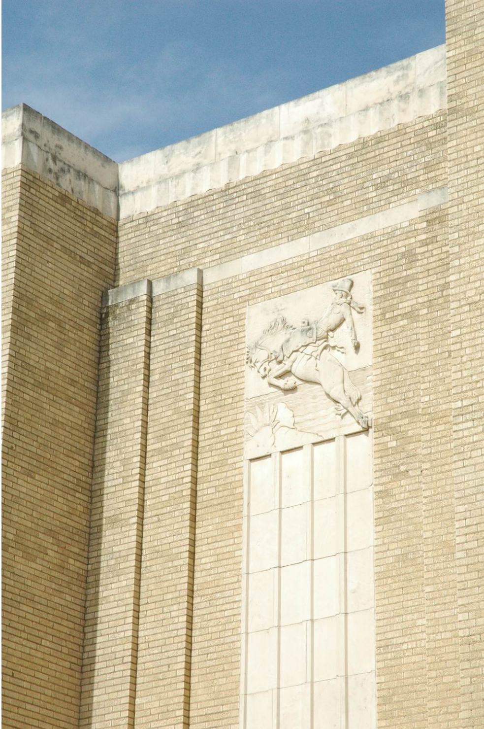
Photo 6 Will Rogers Coliseum cast stone Panel, from east side, south end
