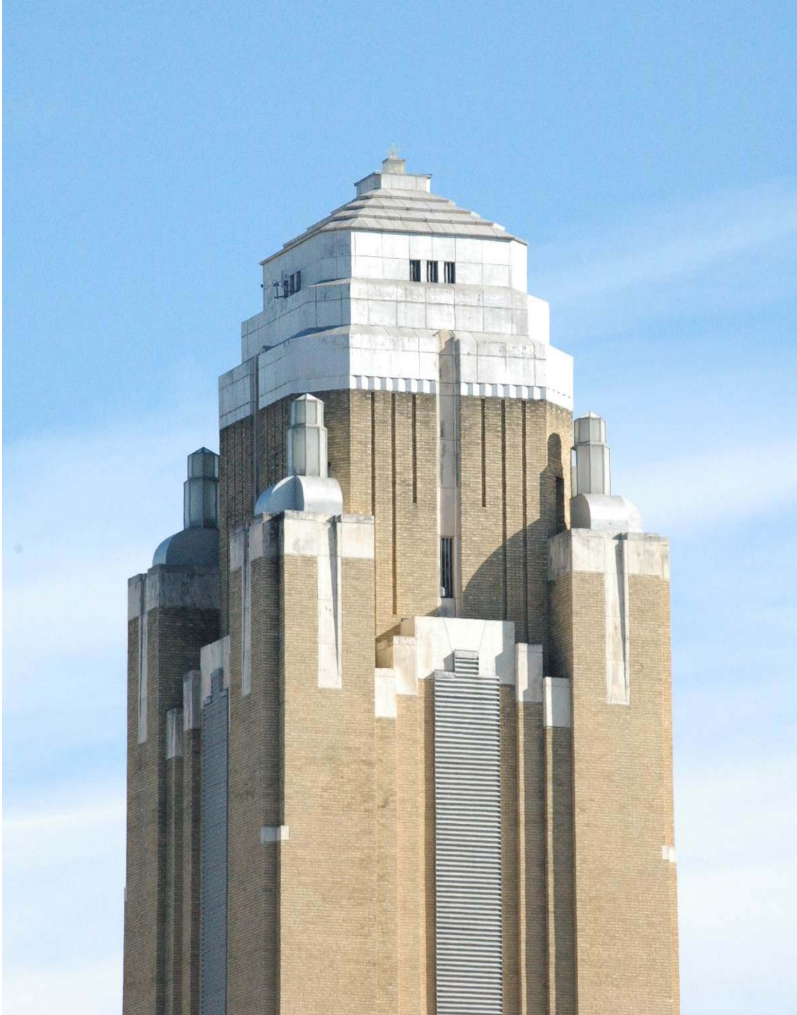
Photo 2 Tower detail Camera facing east
