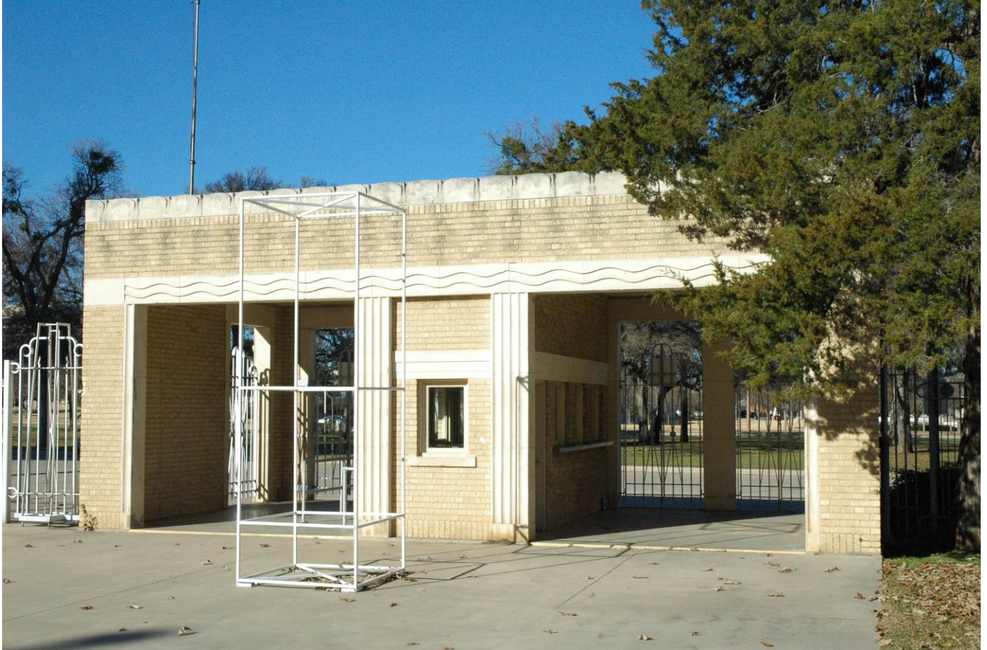
Will Rogers Center, ticket sales building, northwest corner entry Plaza
