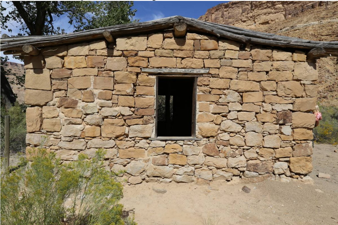
2 of 14. Southeast Façade. Camera facing northwest.
