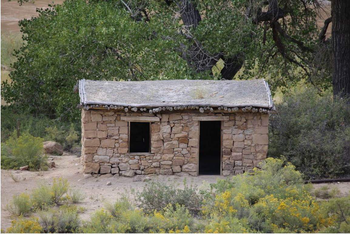
1 of 14. Northeast (Front) Façade. Camera facing southwest.
