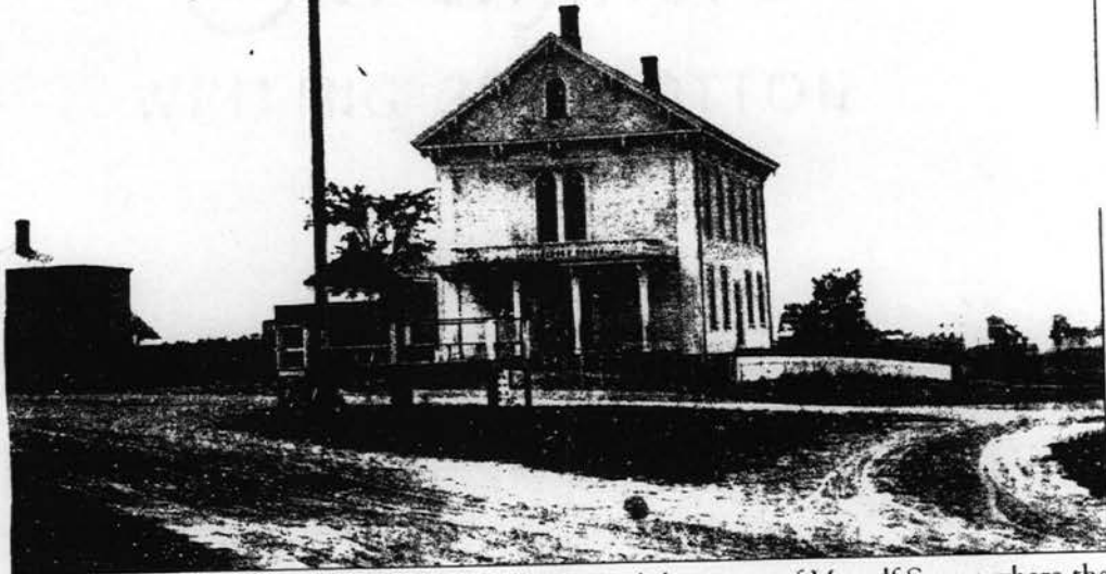
Winthrop's original town hall, built in 1856, occupied the corner of Metcalf Square where the old post office was and where the new police station now stands. The first floor was devoted to two schoolrooms and town offices, while town business was conducted on the second floor. The total cost of this building was $4,990 and served the town well until the present town hall was erected in 1929. Note the bandstand in the center of what is now the square.
