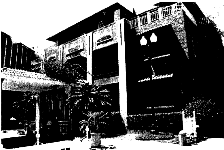
Figure 4: General view of the North facade.
