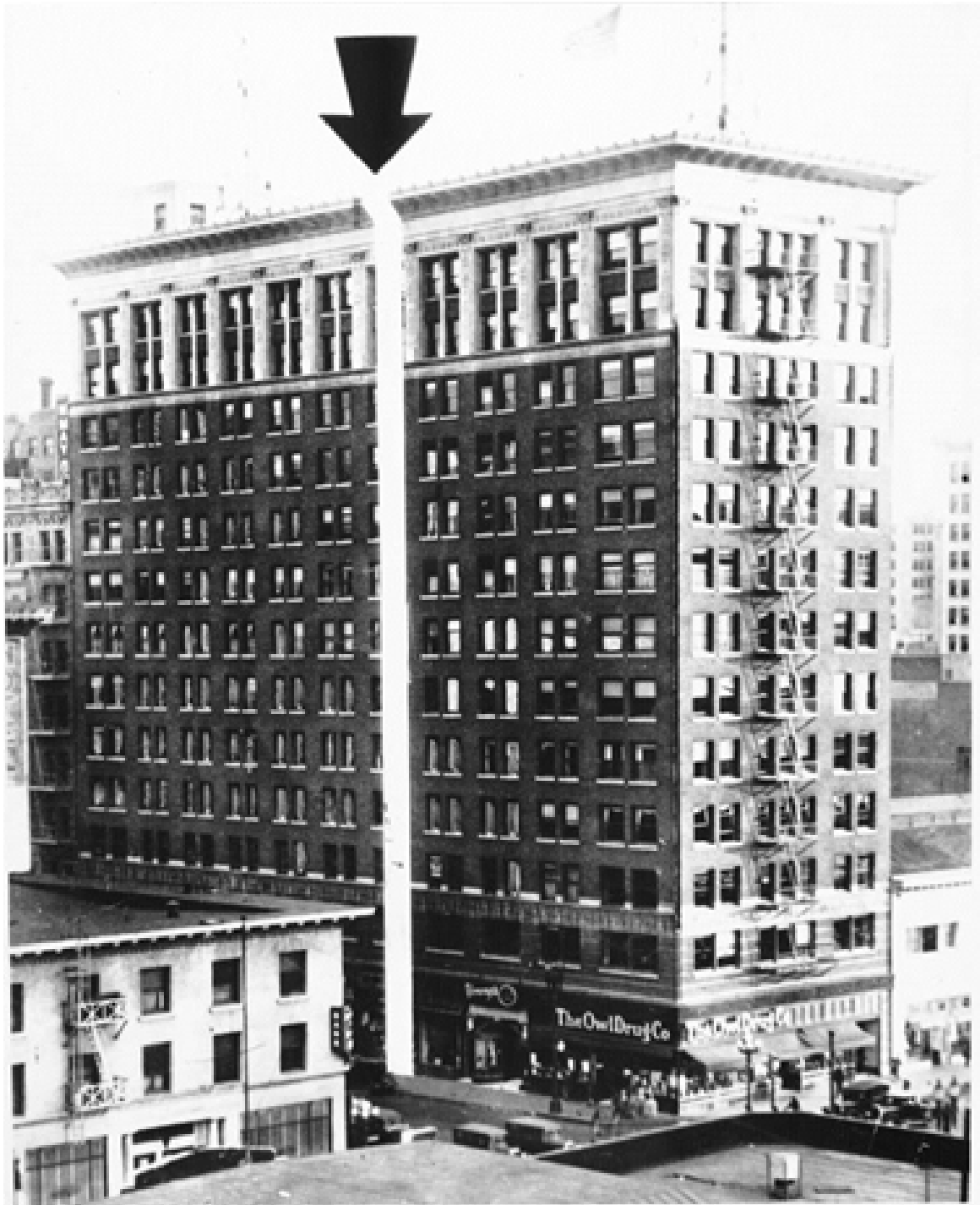
Figure 4. Image illustrates the location and scale of the cut made through the building to accommodate the move of the west portion in 1935. Los Angeles Examiner , USC Special Collection (EXM-P-S-LOS-ANG-CIT-BUI-055)
