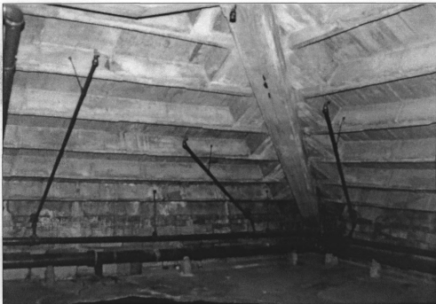
Figure 2: Cast concrete attic roof, 1940 east annex, view southeast (Conard, 1991)
