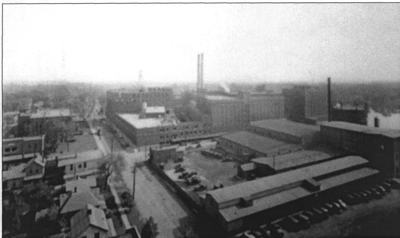
Figure 14: The Administration Building and the Adams Store Building are visible at left center, just behind the tree line that separates them, post-1934 (HAER Documentation)
