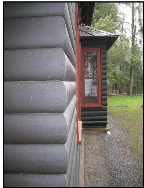
Figure 3. Mitered corners of log trim, southeast corner, 2017.
