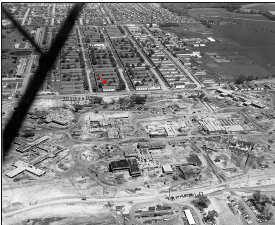
Figure 4. Aerial view of the Topeka VA Hospital during construction, August 1956 (Kansas State Historical Society, Copy and Reuse Restrictions Apply). Highlighted is the chapel that served the Winter General Hospital (then Winter VA Hospital) community; its location relative to the new hospital provided opportunity for continued service. This, however, was met with criticism. See Section 8 below.
