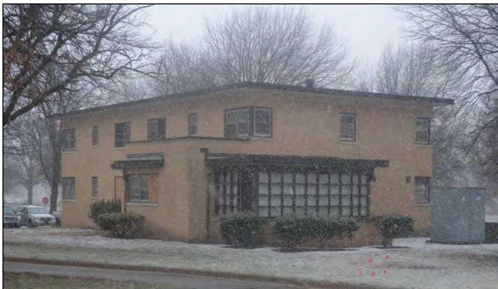
Figure 8. (above) Perspective view looking northeast to the attendants' quarters (mental hygiene) building, 2013; and (below) architectural drawings for the quarters (Building Nos. 60 and 61), 1955 (VA).
