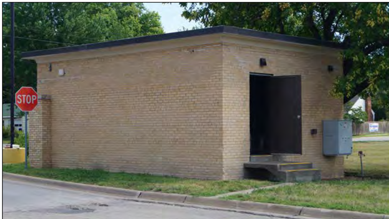
(Perspective view of Building No. 45, looking northeast, courtesy Frances Smith, 2018, VA)
