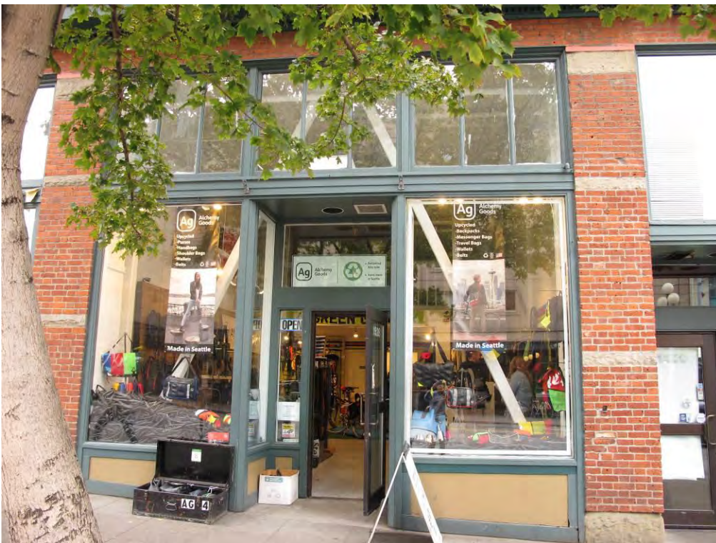
9 of 16. Colonnade Hotel 107 Pine Street, Seattle, King County, WA Photo: The Johnson Partnership, October 5, 2016. Detail at storefront.
