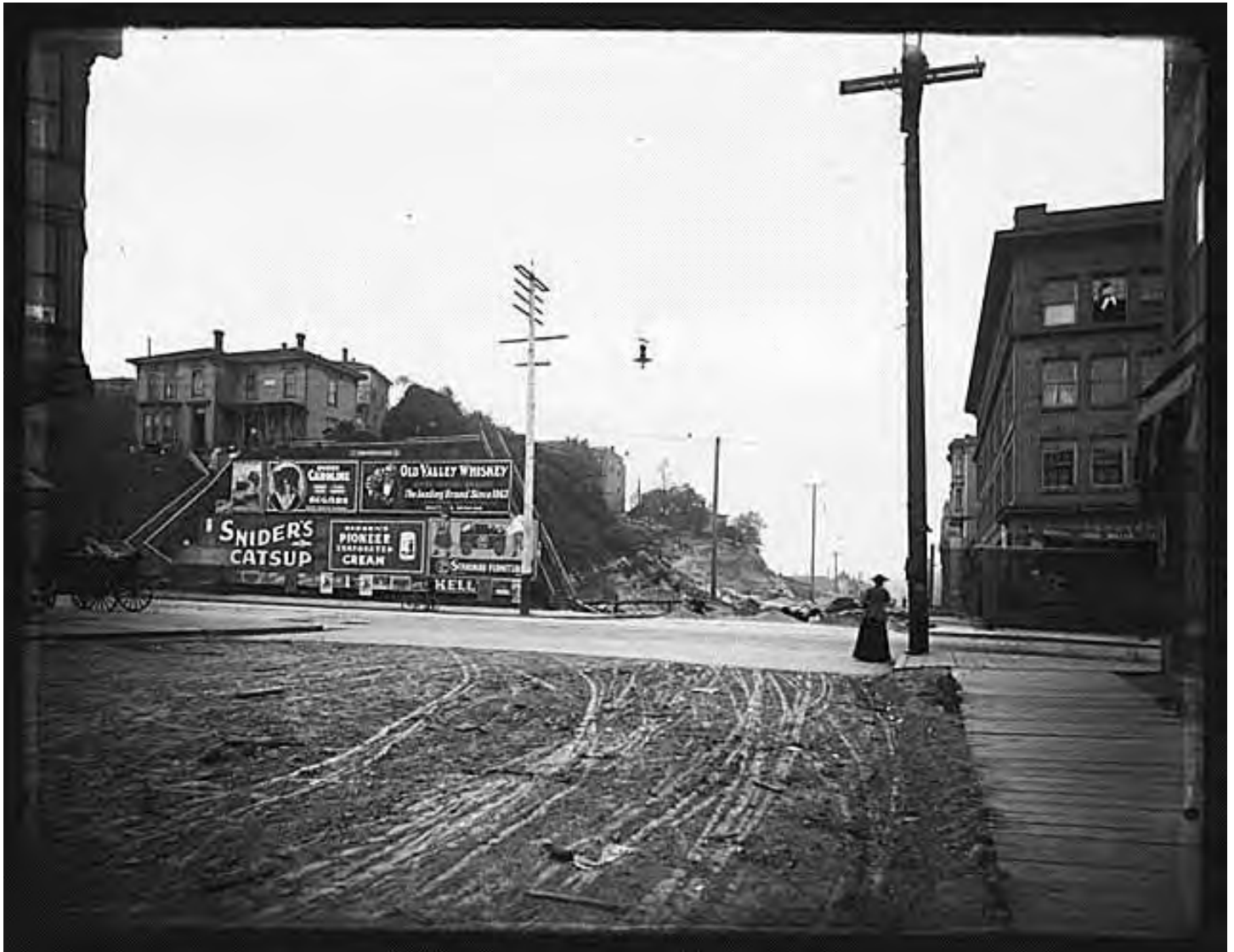
University of Washington Libraries Special Collections. Negative # Warner 269. Collection: PHColl 273 Arthur Churchill Warner Collection. Photographer Warner, Arthur Churchill, 1864-1943. Description: Pine Street looking northeast at 1 st Avenue, Seattle, probably before the second phase of the Denny Hill regrade, ca. 1904.
