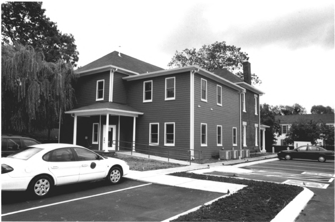
JOHN C. SPENCE HOUSE RUTHERFORD COUNTY, TN
