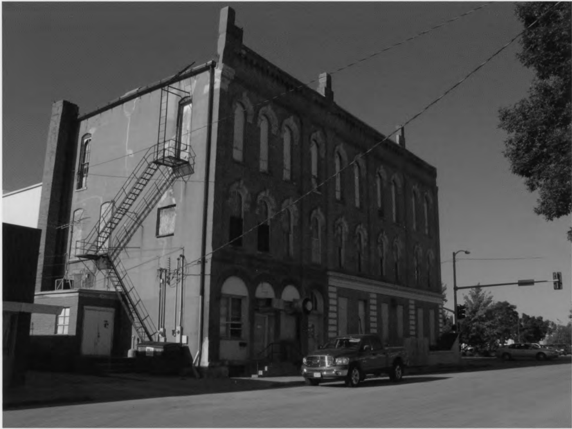
Masonic Building Clarke County, IA #0005
