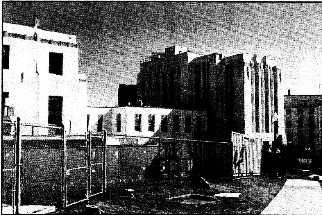
SFVAMC Historic District Building 2- Photograph No. 8 Building 2 is a contributing building in the Historic District Date: October 2008 View: West wing-NW facade & south facade Camera facing: NE
