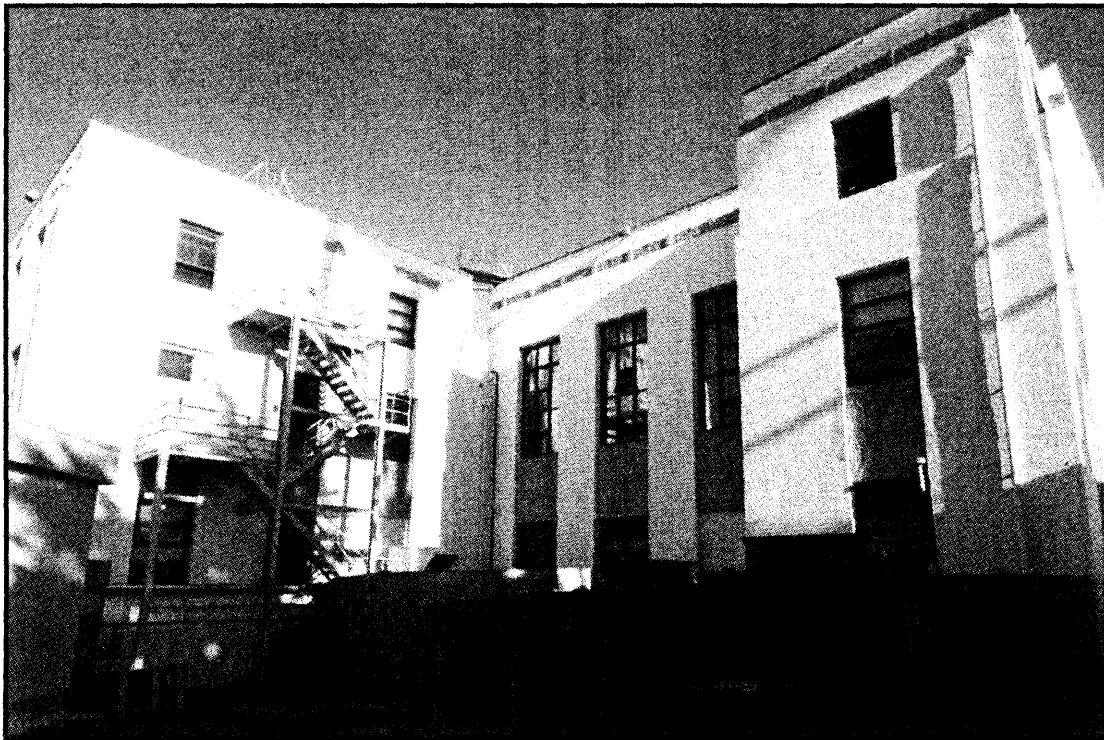
SFVAMC Historic District Building 6 - Photograph No. 8 Building 6 is a contributing building in the Historic District Date: October 2008 View: West interior facade Camera facing: SW
