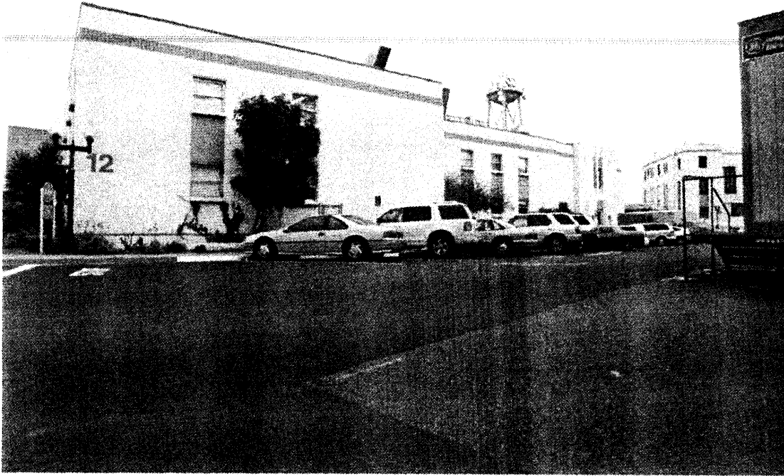
SFVAMC Building 12- Photograph No.1 Building 12 is outside the boundaries of SFVAMC Historic District View East facade - addition (original bay on far right of image) Date: November 26, 2008 Camera facing West
