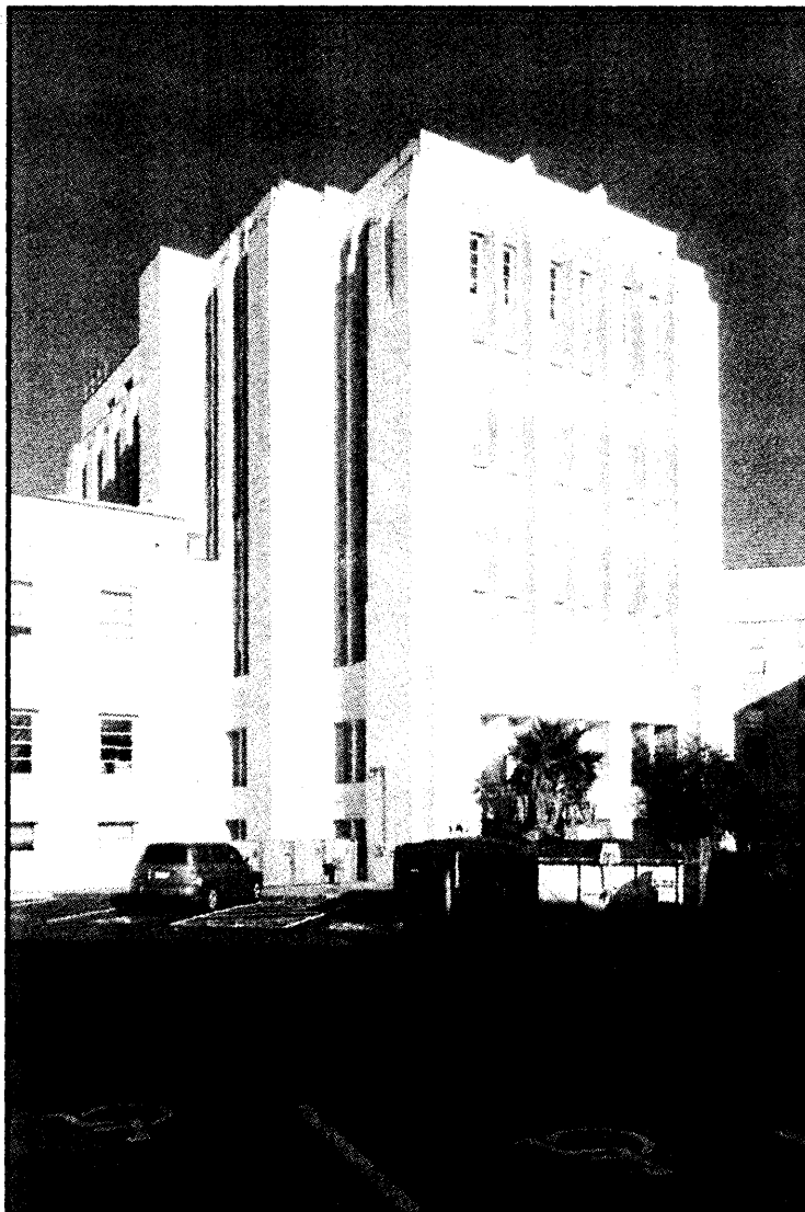
SFVAMC Historic District Building 2- Photograph No. 5 Building 2 is a contributing building in the Historic District Date: October 2008 View: West wing- west & south facade Camera facing: NE
