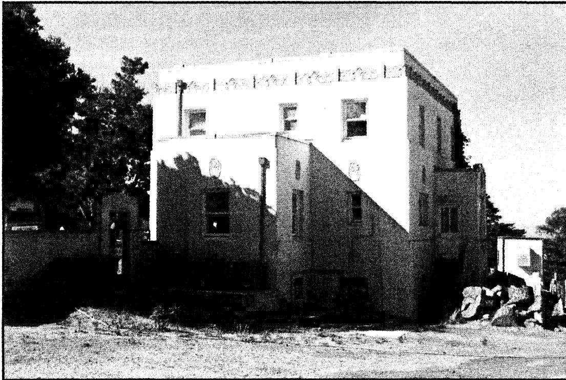
SFVAMC Historic District Building 11- Photograph No. 3 Building 11 is a contributing building in the Historic District Date: October 2008 View: East and North ( rear) facade Camera facing SW
