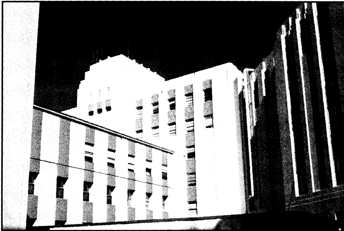
SFVAMC Historic District Building 2- Photograph No. 6 Building 2 is a contributing building in the Historic District Date: October 2008 View: Center (former front) and East wing-south facade Camera facing: N
