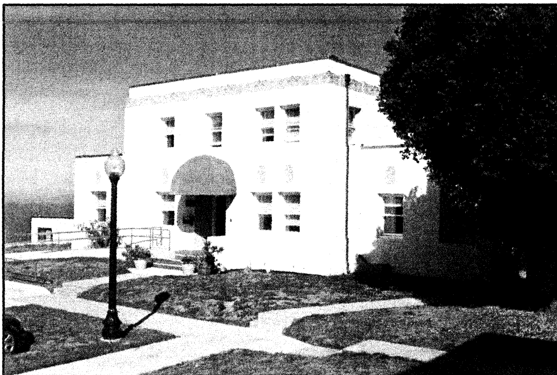
SFVAMC Historic District Building 11- Photograph No. 2 Building 11 is a contributing building in the Historic District Date: October 2008 View: South (Prime) facade Camera facing NW
