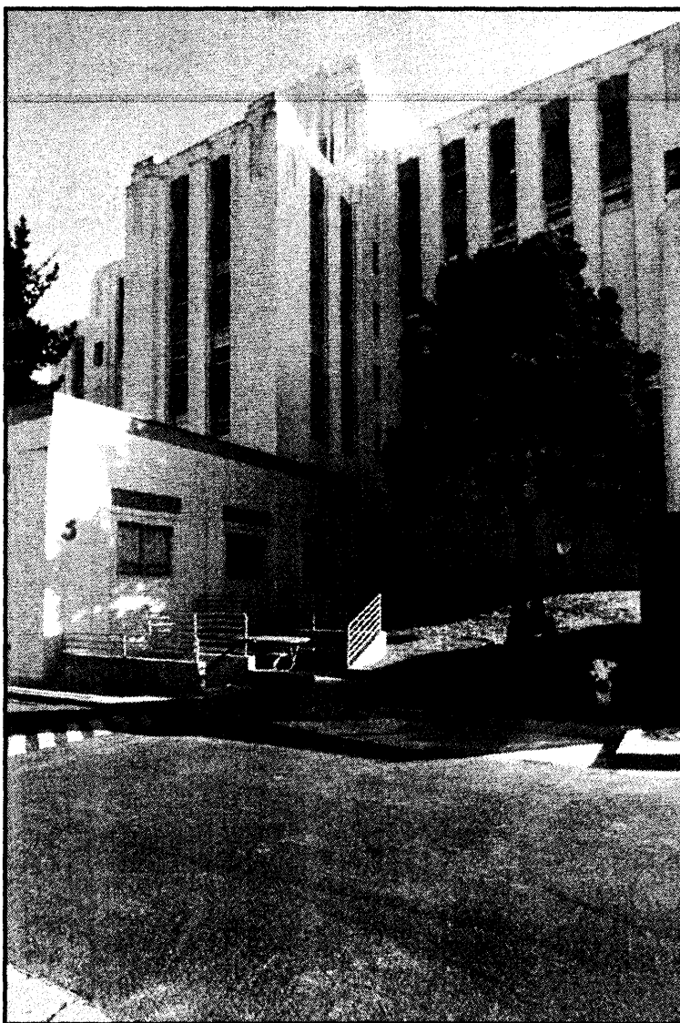
SFVAMC Historic District Building 2- Photograph No. 10 Building 2 is a contributing building in the Historic District Date: October 2008 View: North facade - Center Camera facing: S
