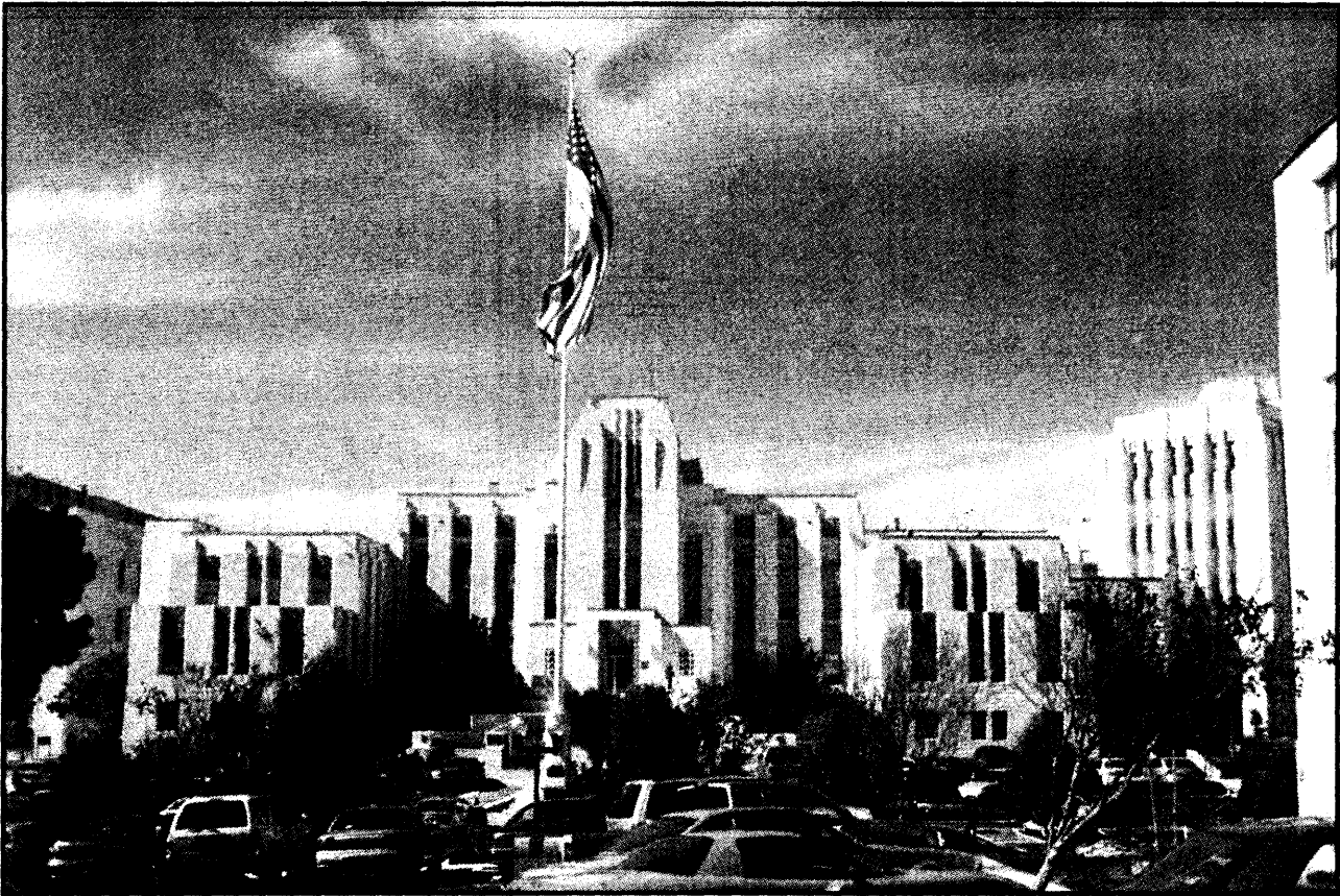
SFVAMC Historic District Building 1- Photograph No. 6 Building 1 is a contributing building in the Historic District Date: October 2008 View: Front facade Camera facing: W
