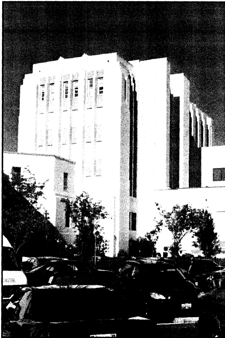
SFVAMC Historic District Building 2- Photograph No. 3 Building 2 is a contributing building in the Historic District Date: October 2008 View West wing-rear-north facade Camera facing: SW
