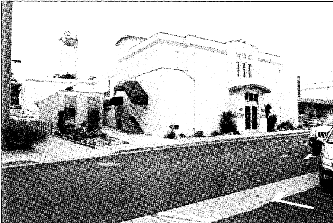
SFVAMC Building 13- Photograph No.1 Building 13 is outside the boundaries of SFVAMC Historic District View West facade-entry bay (remodeled) Date: November 26, 2008 Camera facing NE
