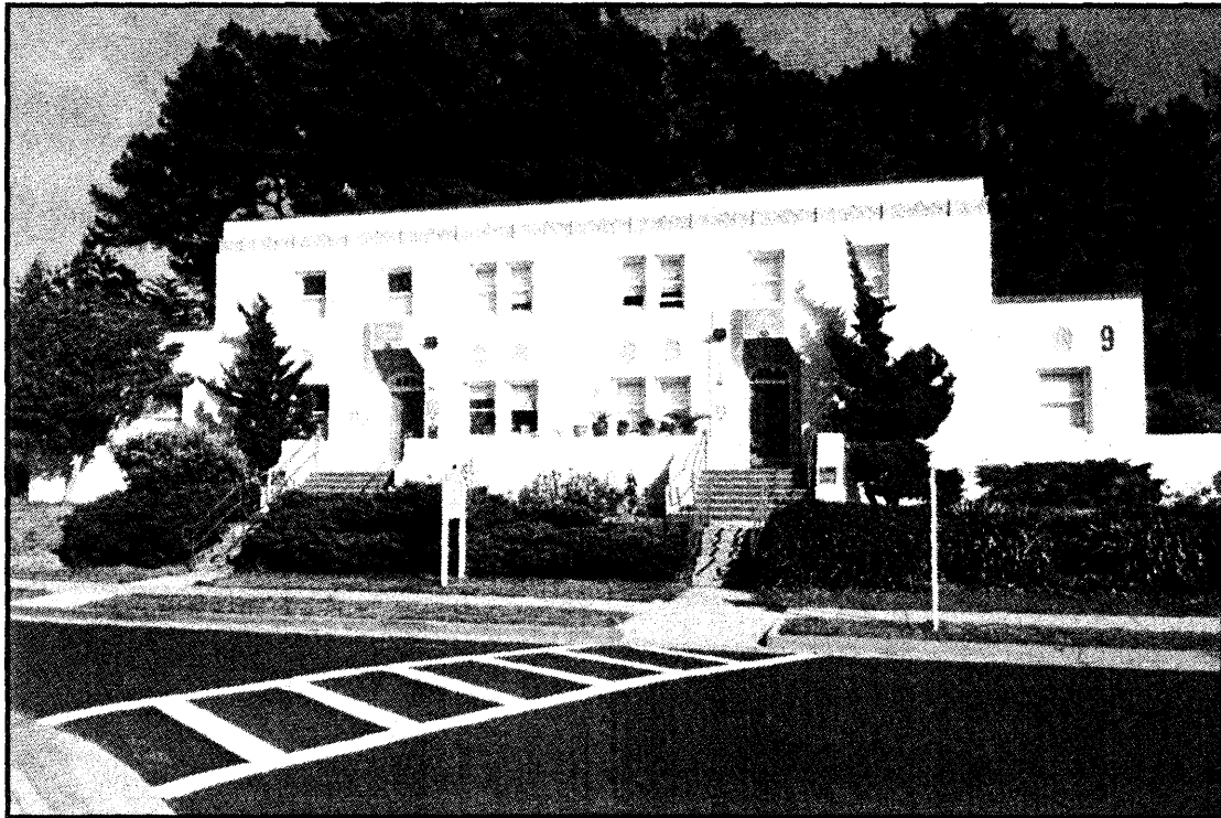
SFVAMC Historic District Building 9- Photograph No. 1 Building 9 is a contributing building in the Historic District Date: October 2008 View: South and west (rear) facade Camera facing NE
