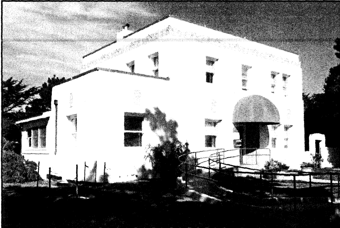
SFVAMC Historic District Building 11- Photograph No. 1 Building 11 is a contributing building in the Historic District Date: October 2008 View: South (Prime) facade Camera facing NE
