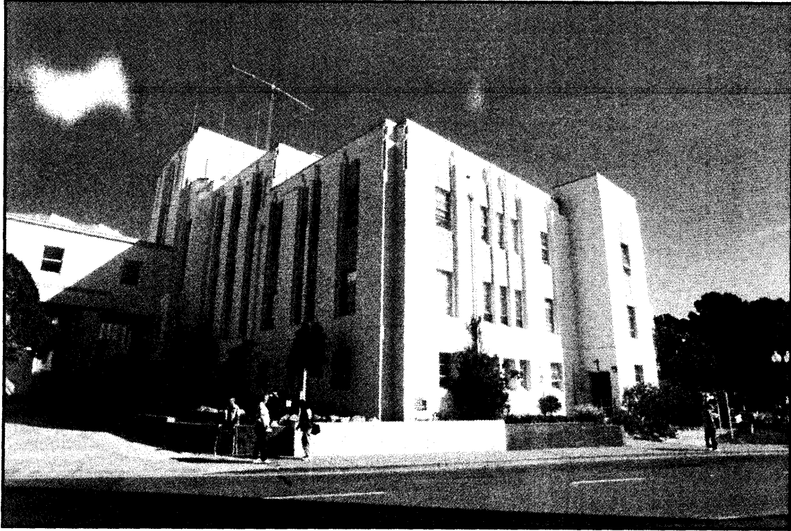
SFVAMC Historic District Building 1- Photograph No. 3 Building 1 is a contributing building in the Historic District Date: October 2008 View: West & South facades Camera facing: NE
