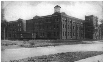
Figure 7-2 The northside railroad spur and loading dock area are evident in this postcard view dated 1908. Also shown is the wing expansion constructed east of the original north side (to the left of the box car), which repeated the architectural program of the original block. The extant power house was constructed later in the grassy area in the far left center of this view. Collection of Jan Olive Nash.
