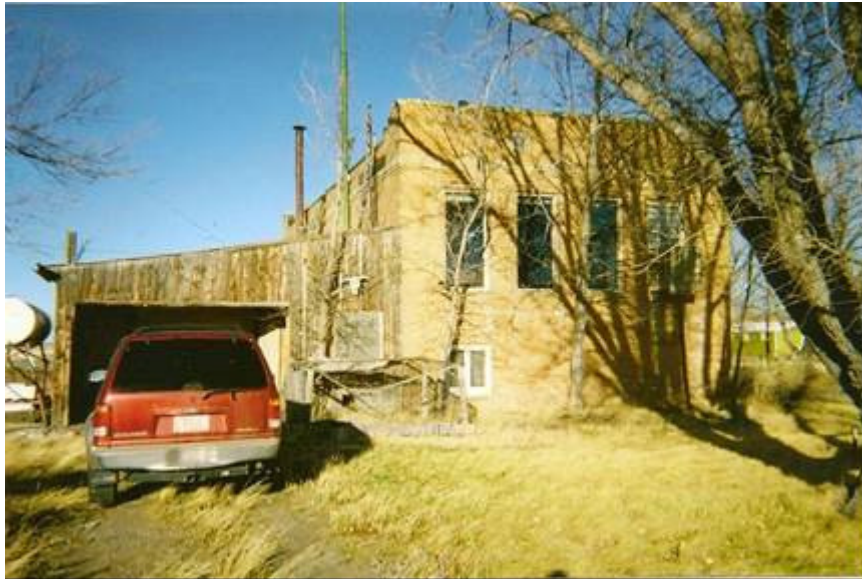
Photo# 0004: south elevation, view to the north.
