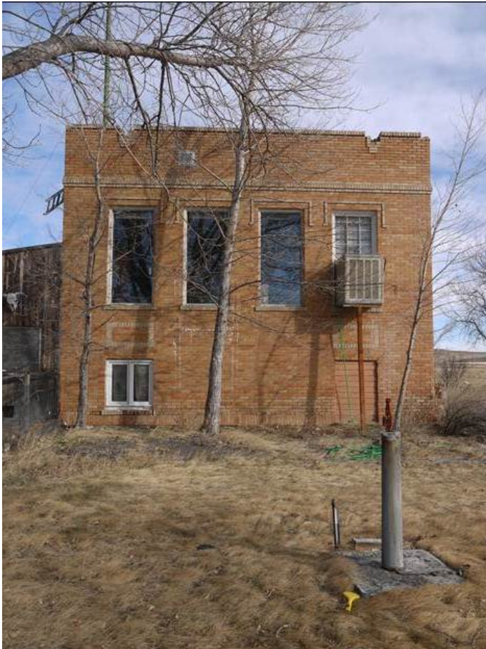
Photo# 0003: south elevation, view to the north.
