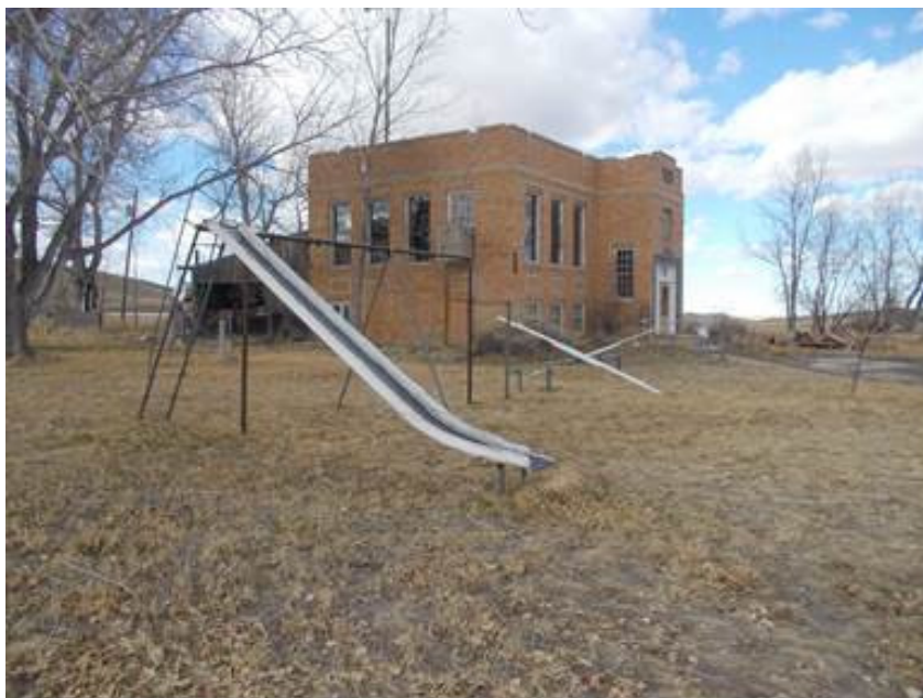
Photo# 0007: Playground equipment, view to the northwest.
