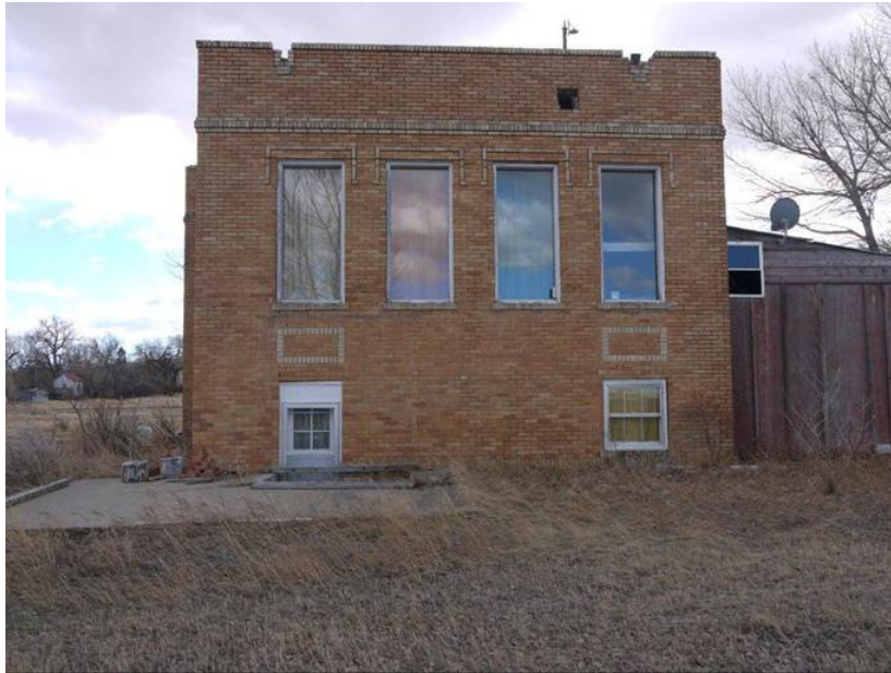
Photo# 0002: North elevation, view to the south.
