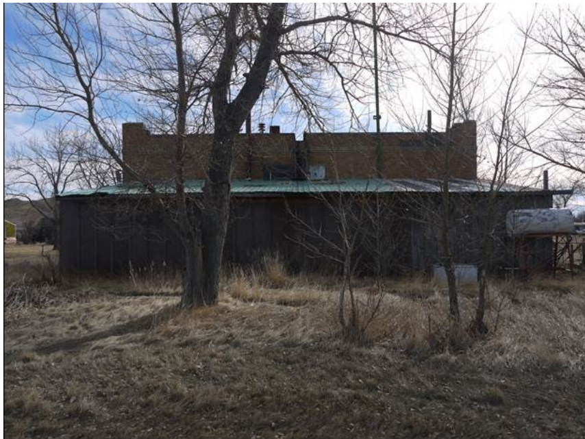
Photo# 0005: west elevation, view to the east.
