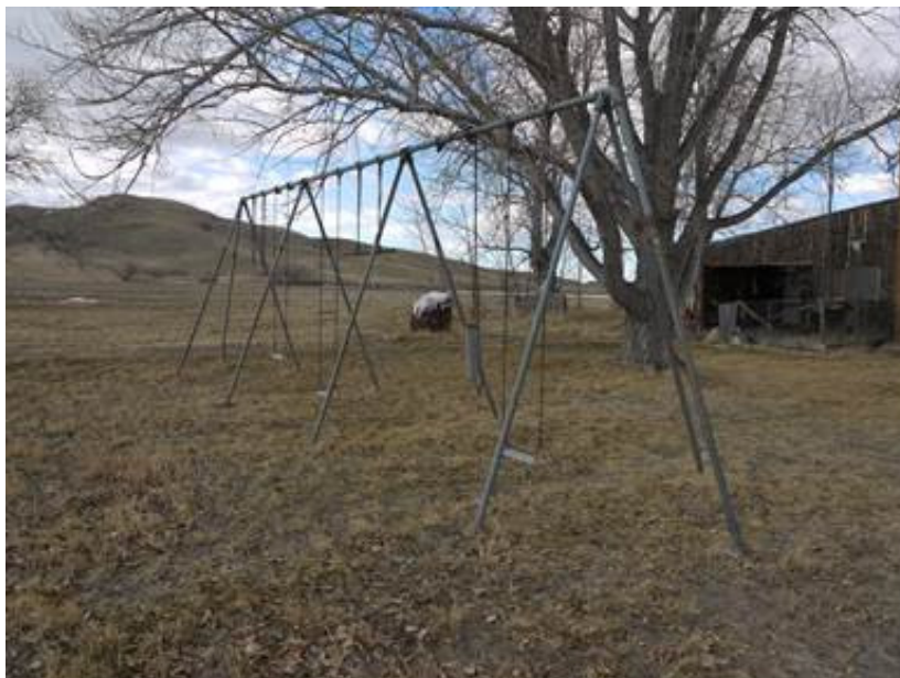
Photo# 0009: Playground equipment, view to the northwest.
