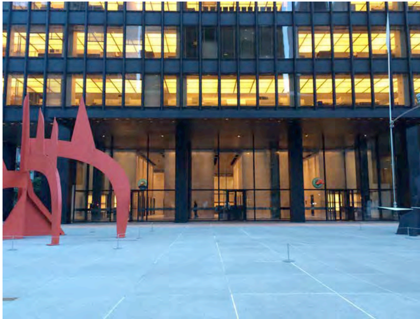
Figure 28: Seagram Building façade as seen from the top of the plaza. Recessed first floor shows travertine walls inside; the upper curtain wall suspends above the colonnade. (Jennifer James)
