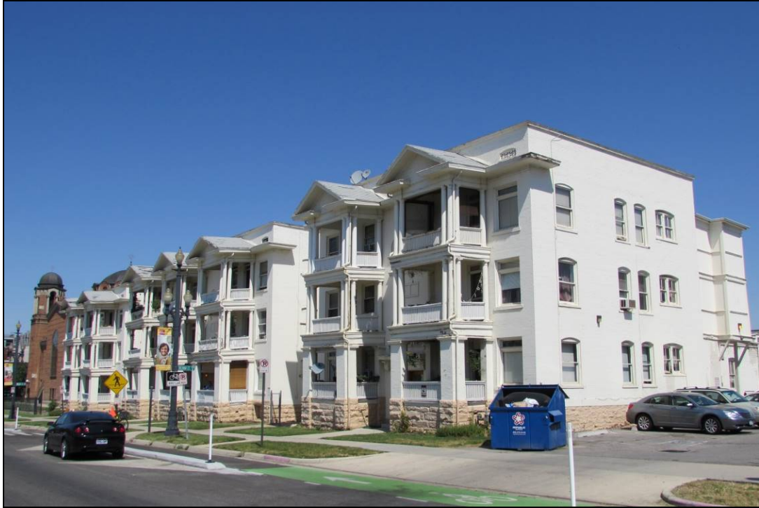
Photograph 13 of 34: Covey Flats/La France walk-up apartments, east (right) and south elevations; camera facing northwest
