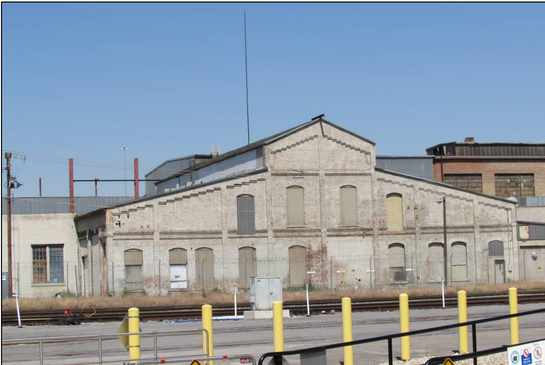
Photograph 10 of 34: D&RGW Boiler House, 669 W. 200 S., east elevation; camera facing west
