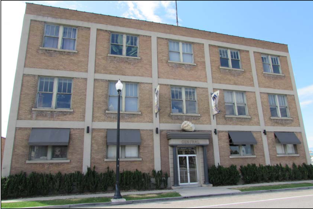
Photograph 31 of 34: International Harvester Building; 435 W. 400 S.; camera facing south
