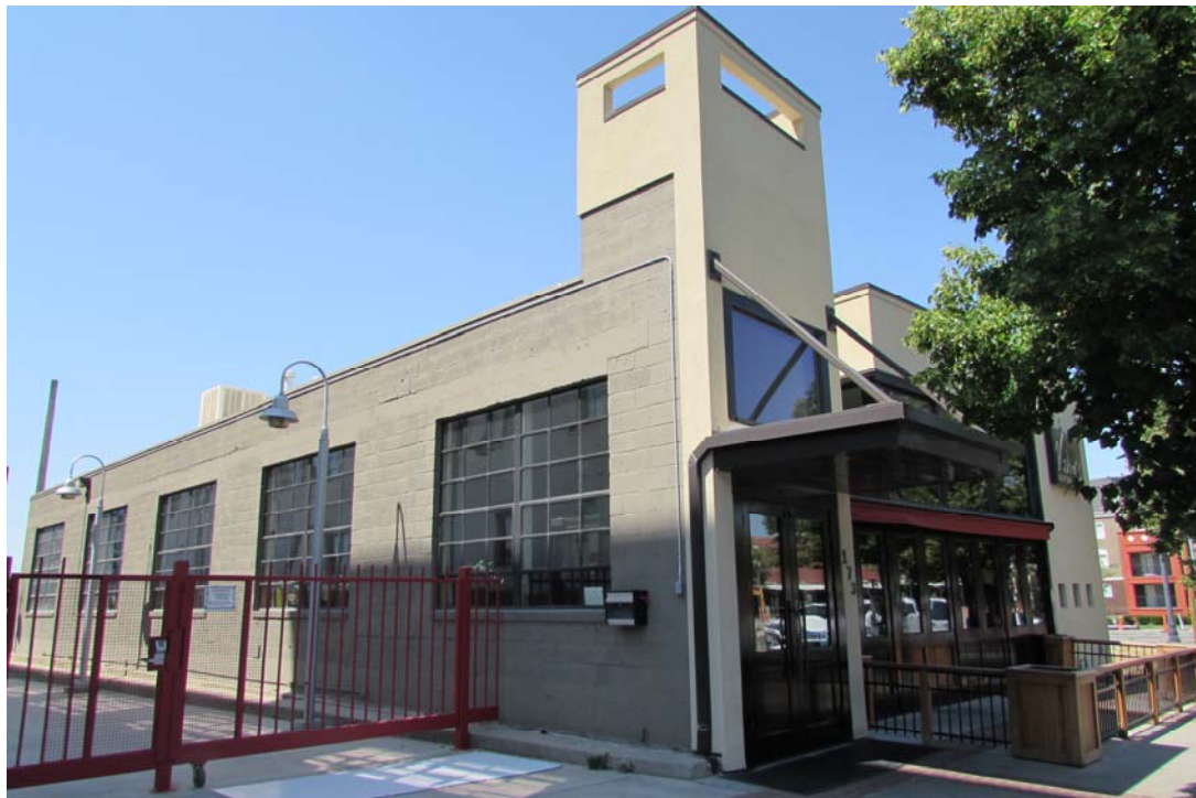
Photograph 6 of 34: Example of non-contributing resource in the district; 173 W. 300 S., east (left) and north elevations; camera facing southwest
