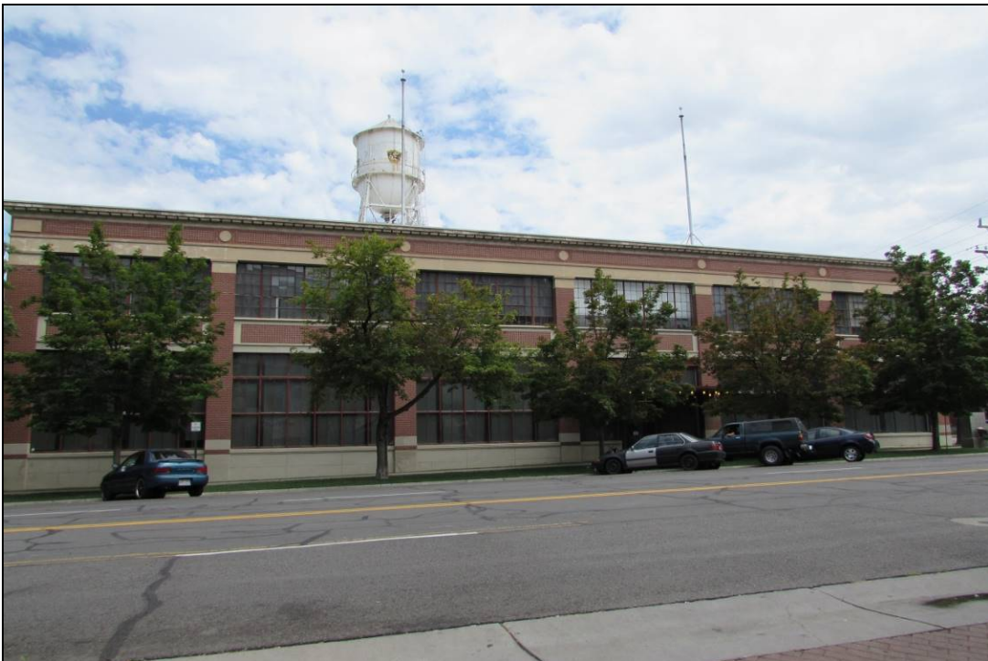
Photograph 12 of 34: Example of 1900-1929 era warehouse; 414 W. 300 S., south elevation; camera facing north
