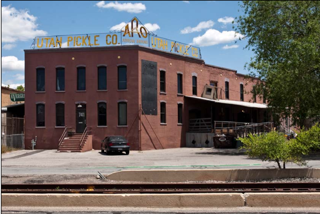
Photograph 29 of 34: Grant Soap/Utah Pickle Factory; 741 S. 400 W.; camera facing east
