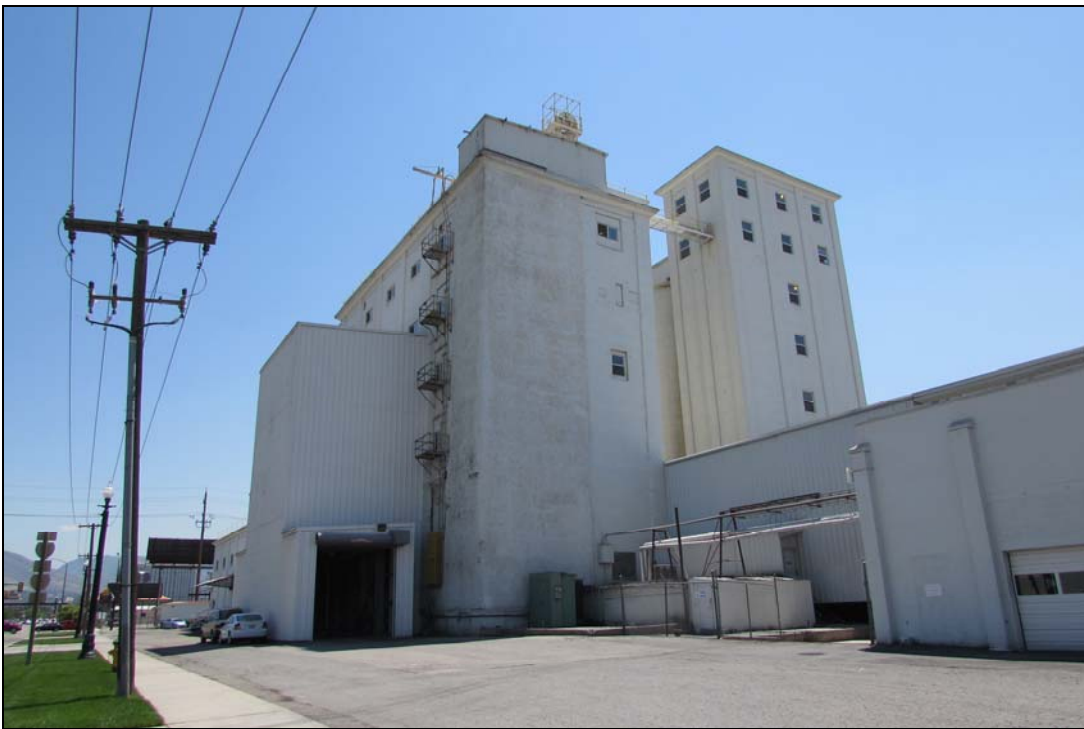
Photograph 32 of 34: Husler Mill/Utah Flour; 425 W. 500 S.; camera facing southwest
