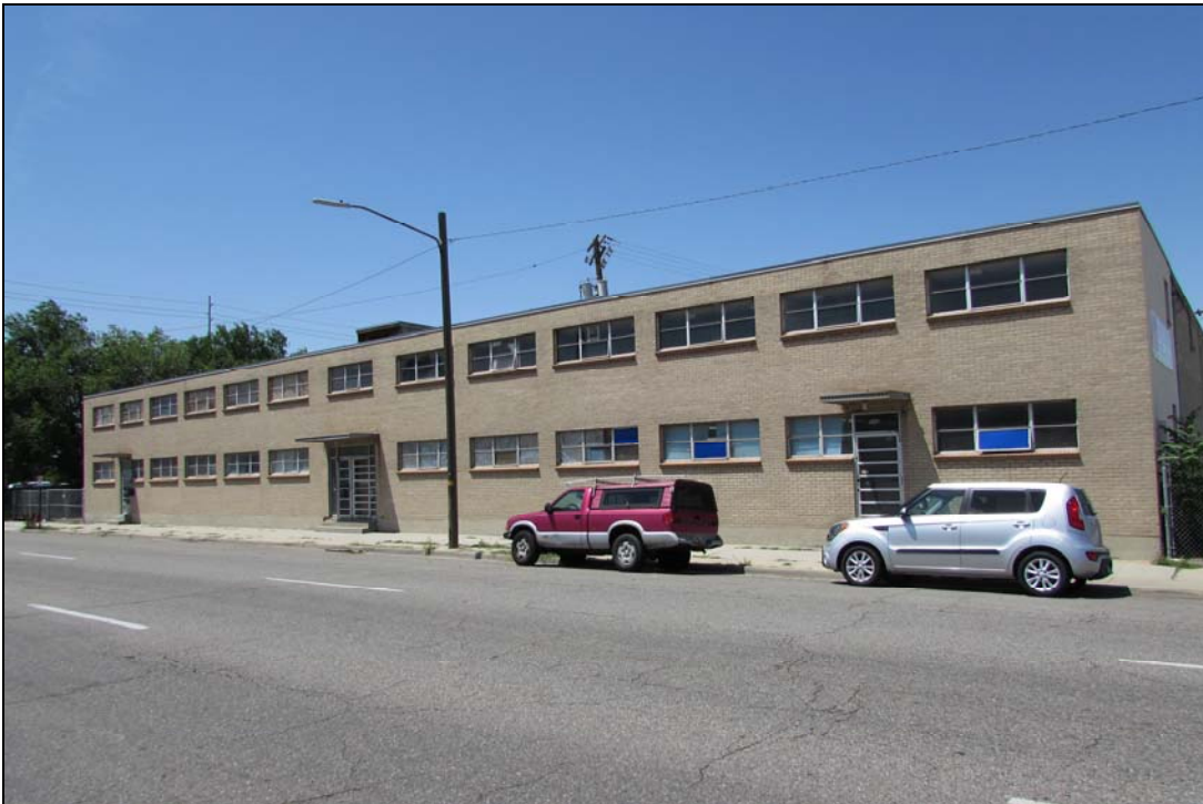
Photograph 34 of 34: Wycoff building; 540-560 S. 300 W.; camera facing southwest
