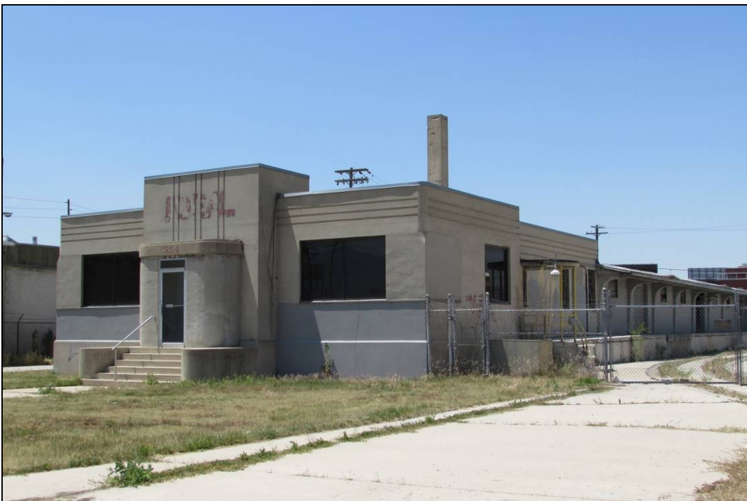
Photograph 22 of 34: Ideal Cement Co.; 554 S. 400 W., north (right) and east elevations; camera facing southwest
