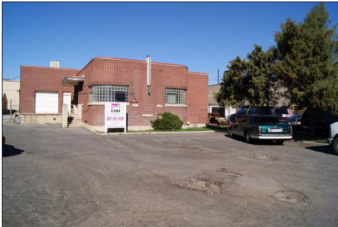
Photograph 26 of 34: 726 S. 400 W., east elevation; camera facing west
