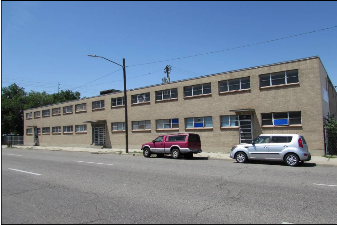
Photograph 25 of 34: 540-560 S. 300 W., east elevation; camera facing southwest
