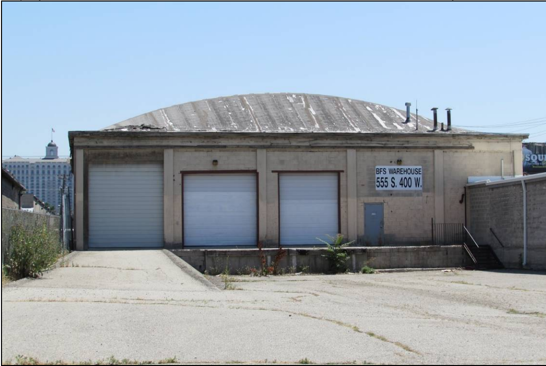
Photograph 23 of 34: Drive-up warehouse; 555 S. 400 W., west elevation; camera facing east
