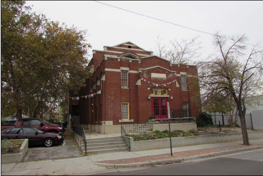
Photograph 17 of 34: LDS Fifth Ward Chapel; 740 S. 300 W., east elevation; camera facing northwest
