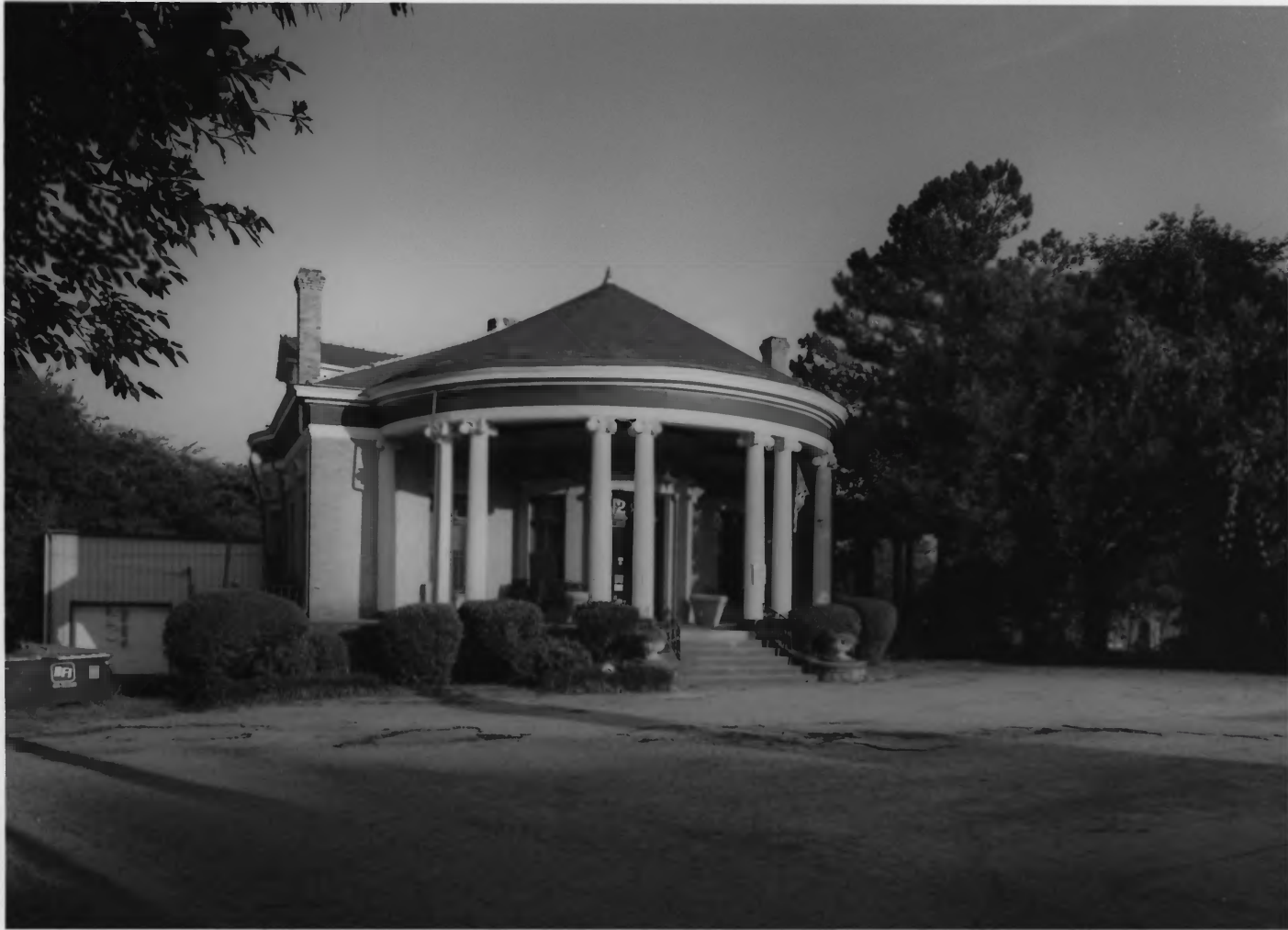
INMAN PARK-MORELAND HISTORIC DISTRICT AMENDMENT ATLANTA, FULTON COUNTY, GEORGIA PHOTOGRAPH 15 OF 42
