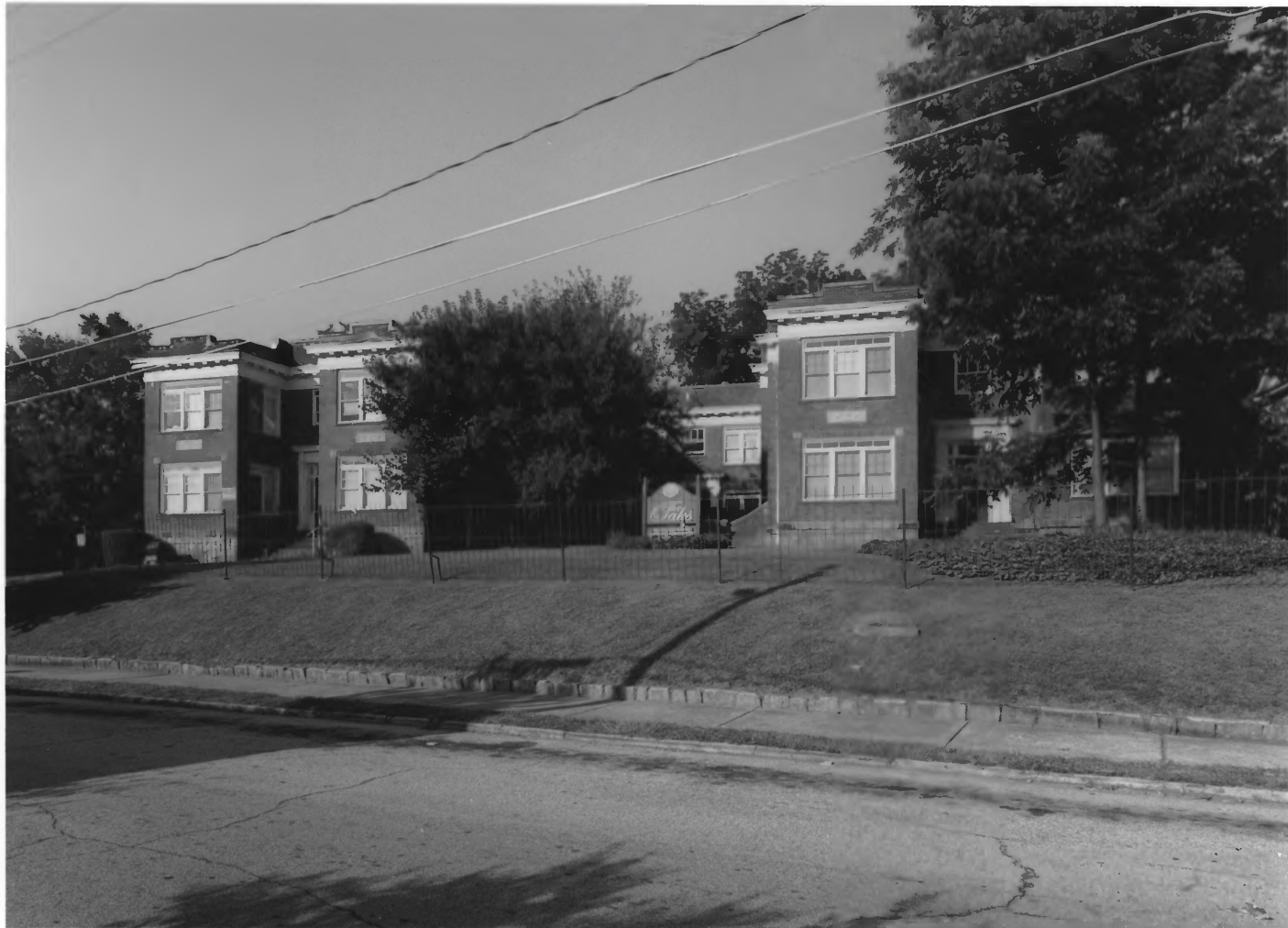
INMAN PARK-MORELAND HISTORIC DISTRICT AMENDMENT ATLANTA, FULTON COUNTY, GEORGIA PHOTOGRAPH 32 OF 42
