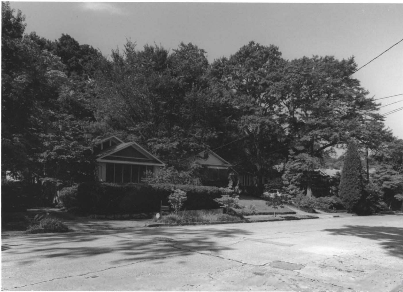
INMAN PARK-MORELAND HISTORIC DISTRICT AMENDMENT ATLANTA, FULTON COUNTY, GEORGIA PHOTOGRAPH 2 OF 42
