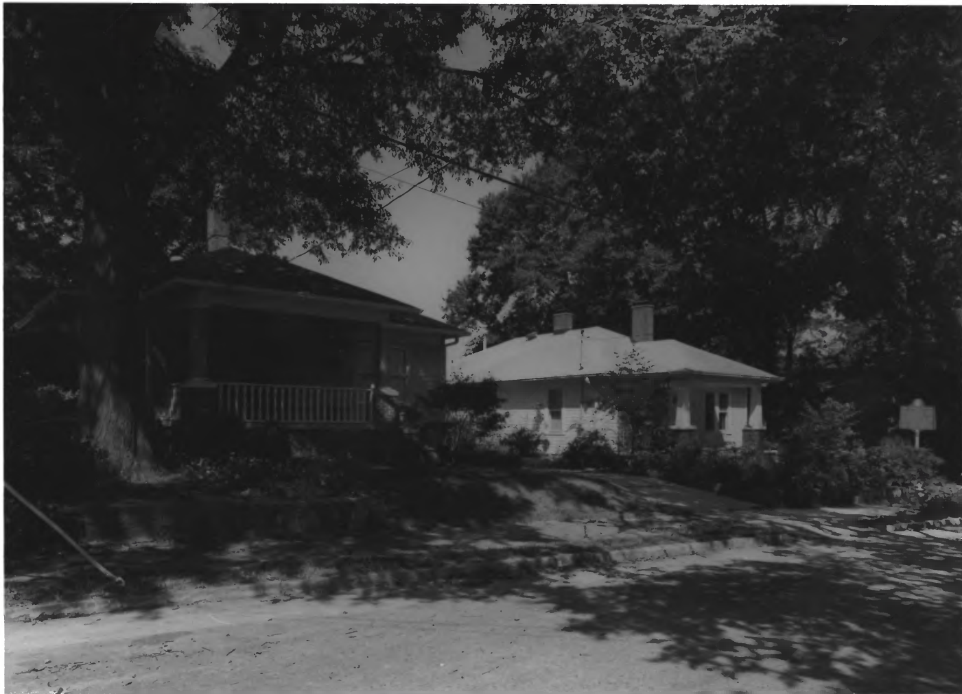
INMAN PARK - MORELAND HISTORIC DISTRICT AMENDMENT ATLANTA, FULTON COUNTY, GEORGIA PHOTOGRAPH 7 OF 42
