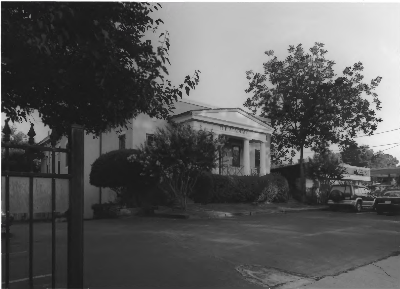
INMAN PARK-MORELAND HISTORIC DISTRICT AMENDMENT ATLANTA, FULTON COUNTY, GEORGIA PHOTOGRAPH 17 OF 42
