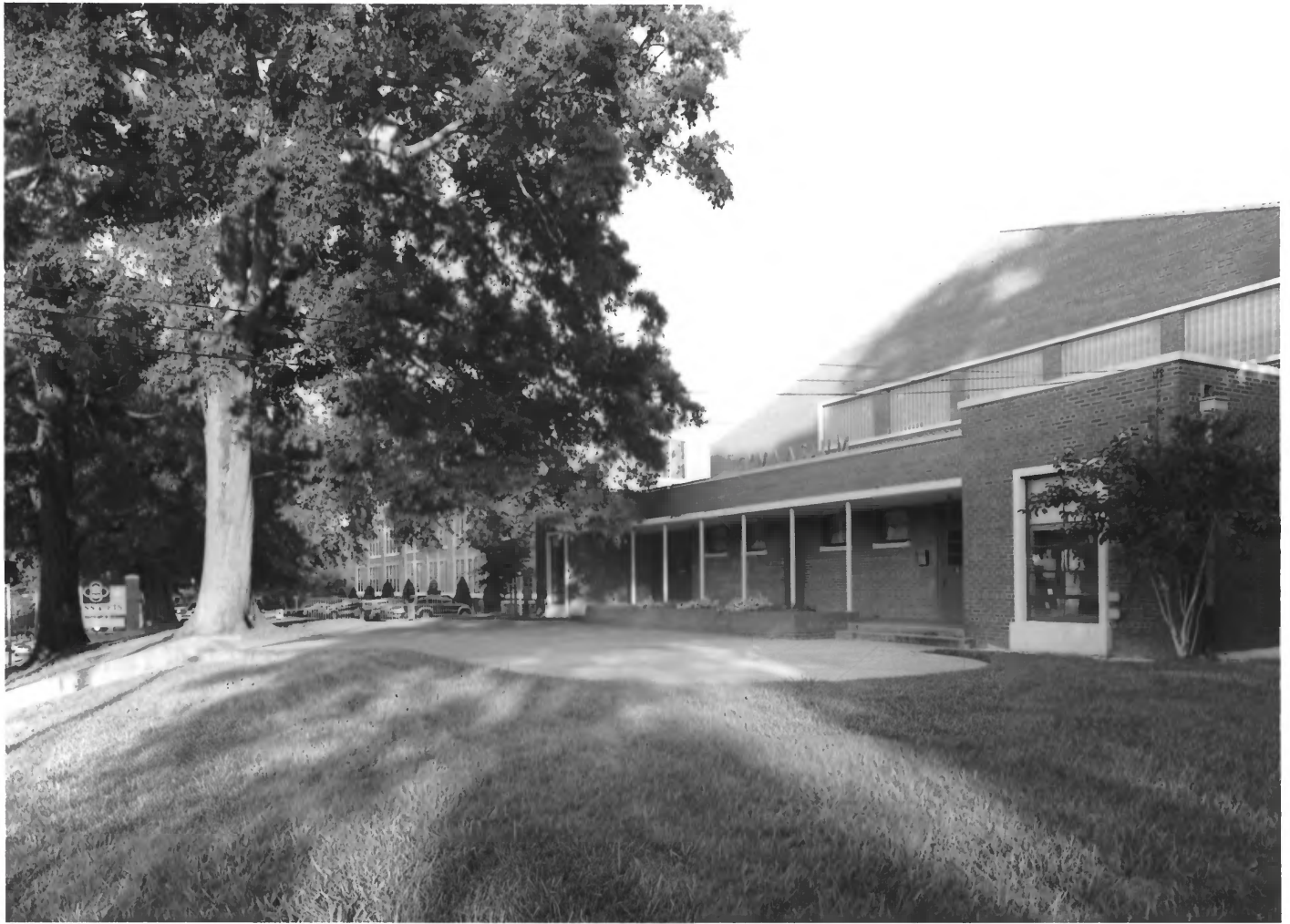
INMAN PARK-MORELAND HISTORIC DISTRICT AMENDMENT ATLANTA, FULTON COUNTY, GEORGIA PHOTOGRAPH 24 OF 42
