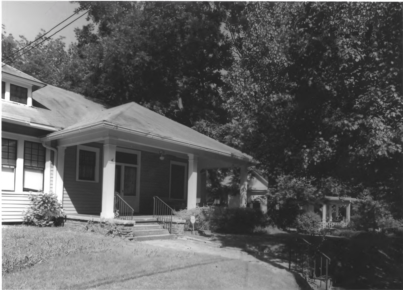
INMAN PARK-MORELAND HISTORIC DISTRICT AMENDMENT ATLANTA, FULTON COUNTY, GEORGIA PHOTOGRAPH 4 OF 42
