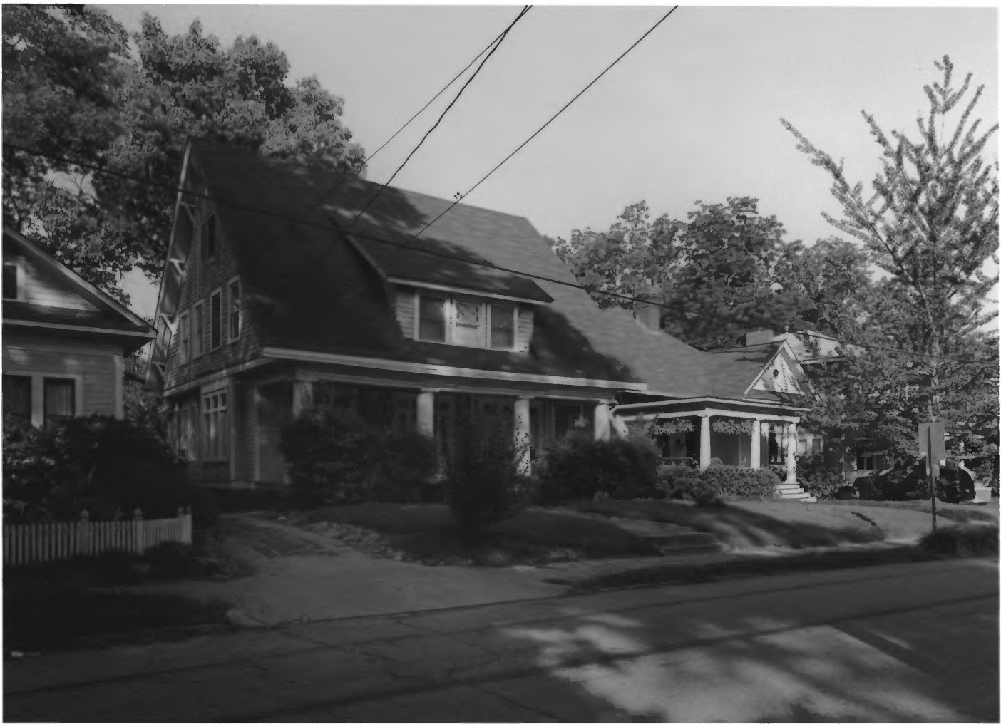
INMAN PARK-MORELAND HISTORIC DISTRICT AMENDMENT ATLANTA, FULTON COUNTY, GEORGIA PHOTOGRAPH 37 of 42
