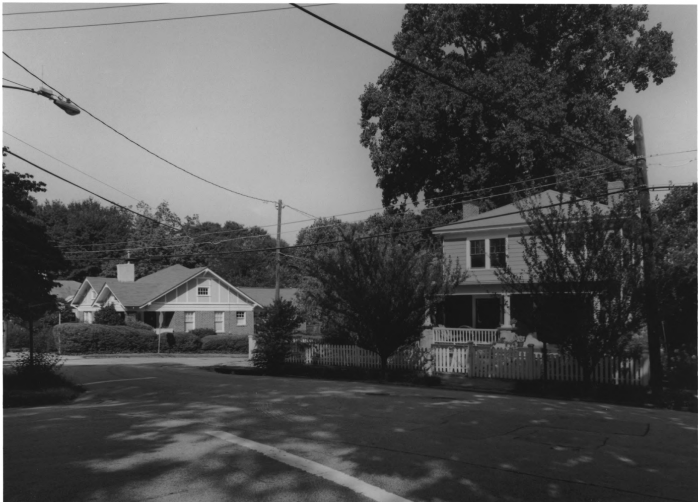
INMAN PARK-MORELAND HISTORIC DISTRICT AMENDMENT ATLANTA, FULTON COUNTY, GEORGIA PHOTOGRAPH 11 OF 42
