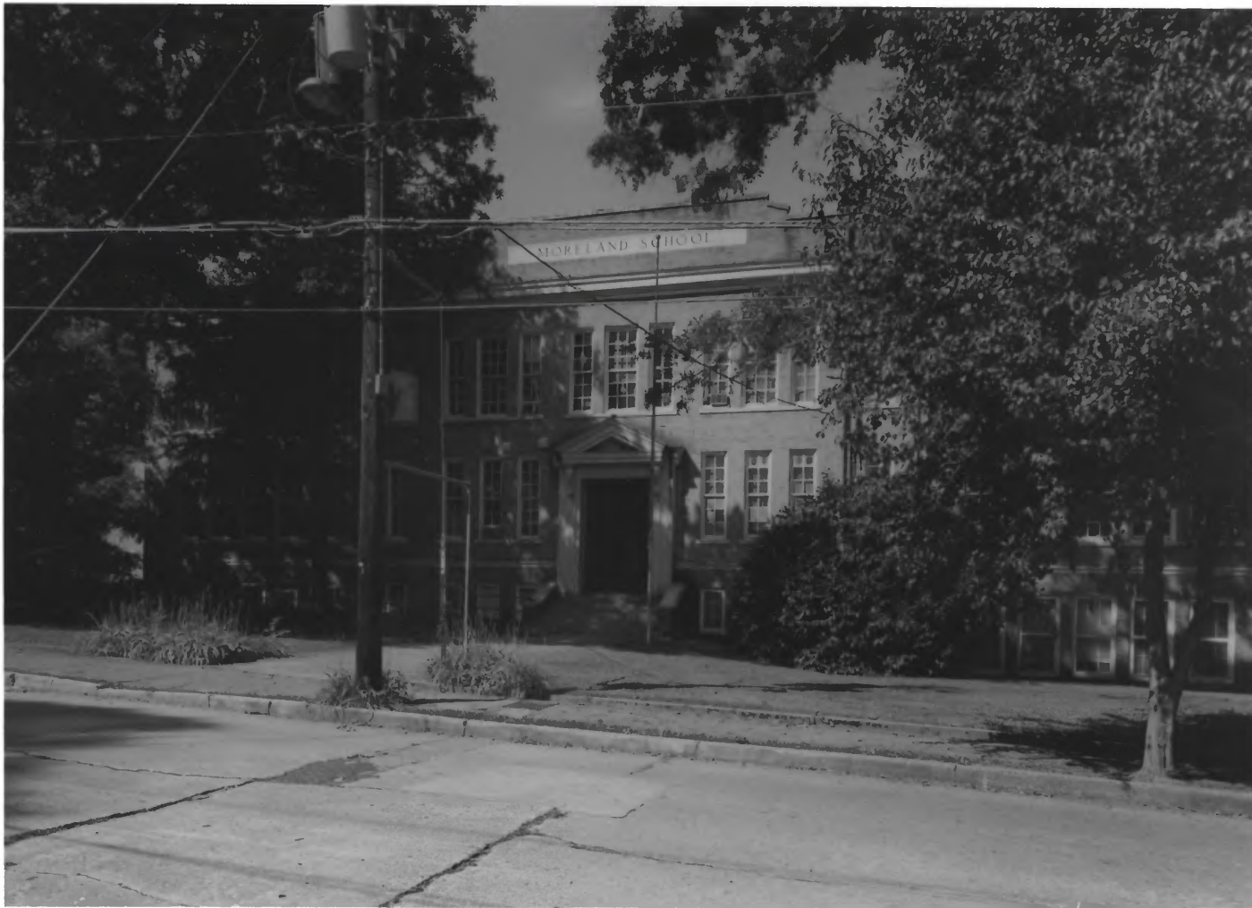
INMAN PARK-MORELAND HISTORIC DISTRICT AMENDMENT ATLANTA, FULTON COUNTY, GEORGIA PHOTOGRAPH 9 OF 42
