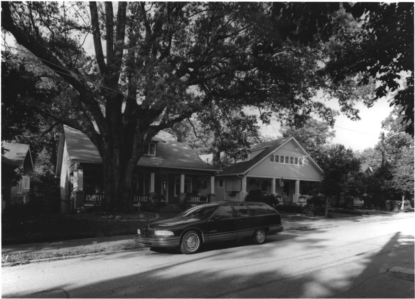
INMAN PARK-MORELAND HISTORIC DISTRICT AMENDMENT ATLANTA, FULTON COUNTY, GEORGIA PHOTOGRAPH 33 OF 42
