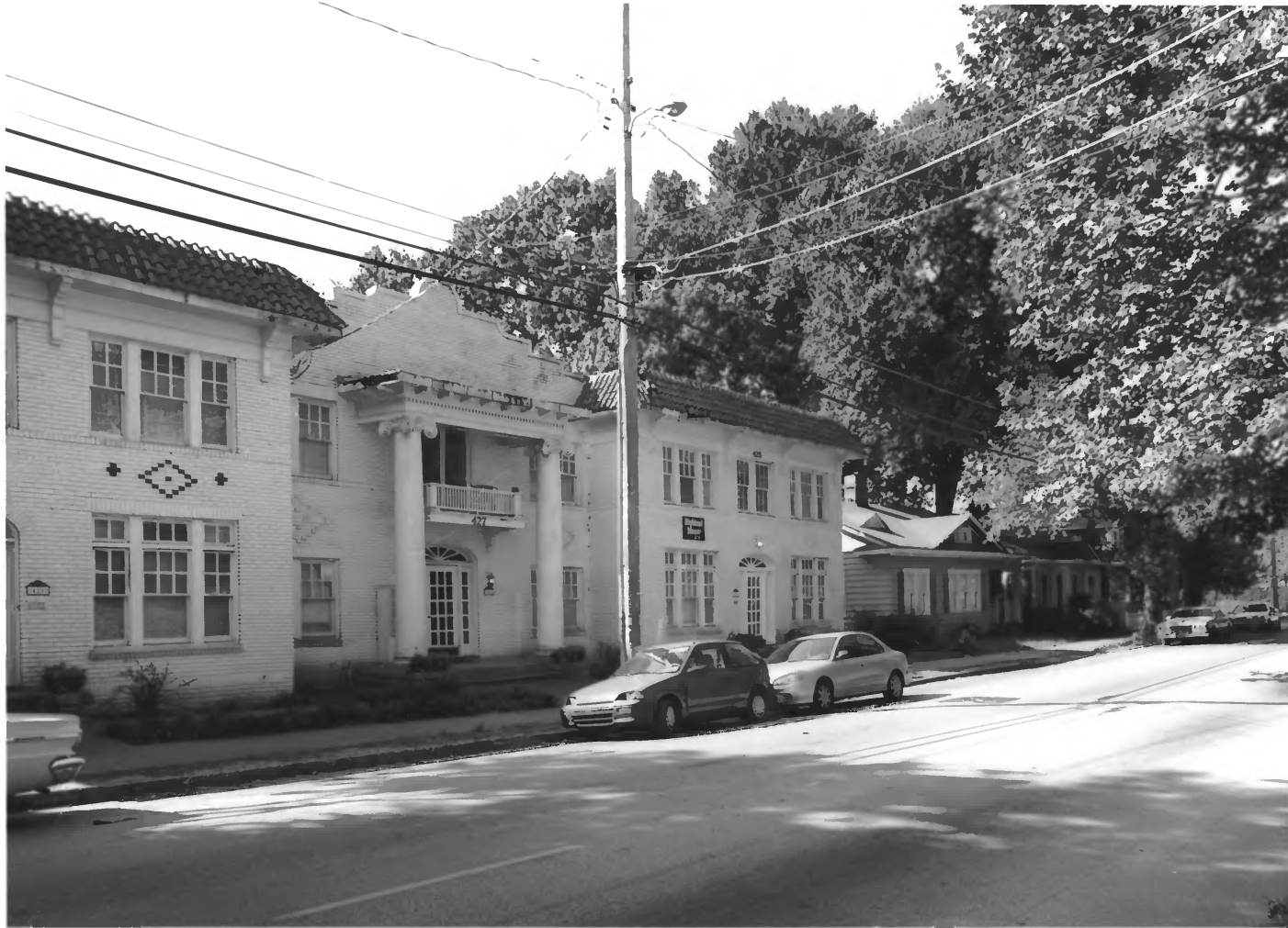
INMAN PARK-MORELAND HISTORIC DISTRICT AMENDMENT ATLANTA, FULTON COUNTY, GEORGIA PHOTOGRAPH 41 OF 42
