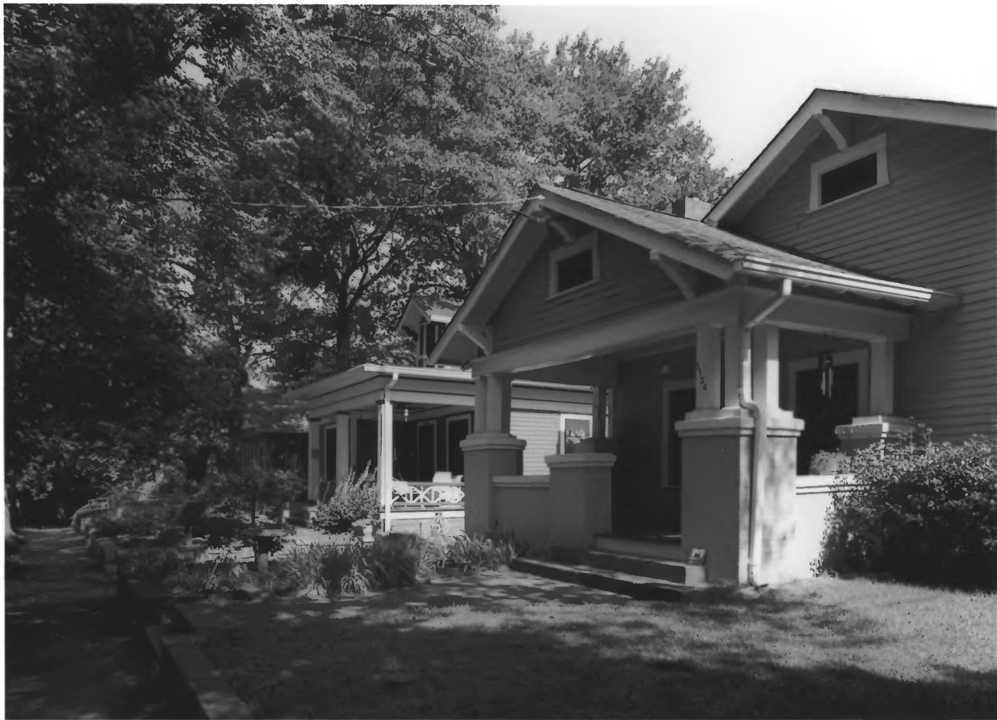
INMAN PARK-MORELAND HISTORIC DISTRICT AMENDMENT ATLANTA, FULTON COUNTY, GEORGIA PHOTOGRAPH 1 OF 42
