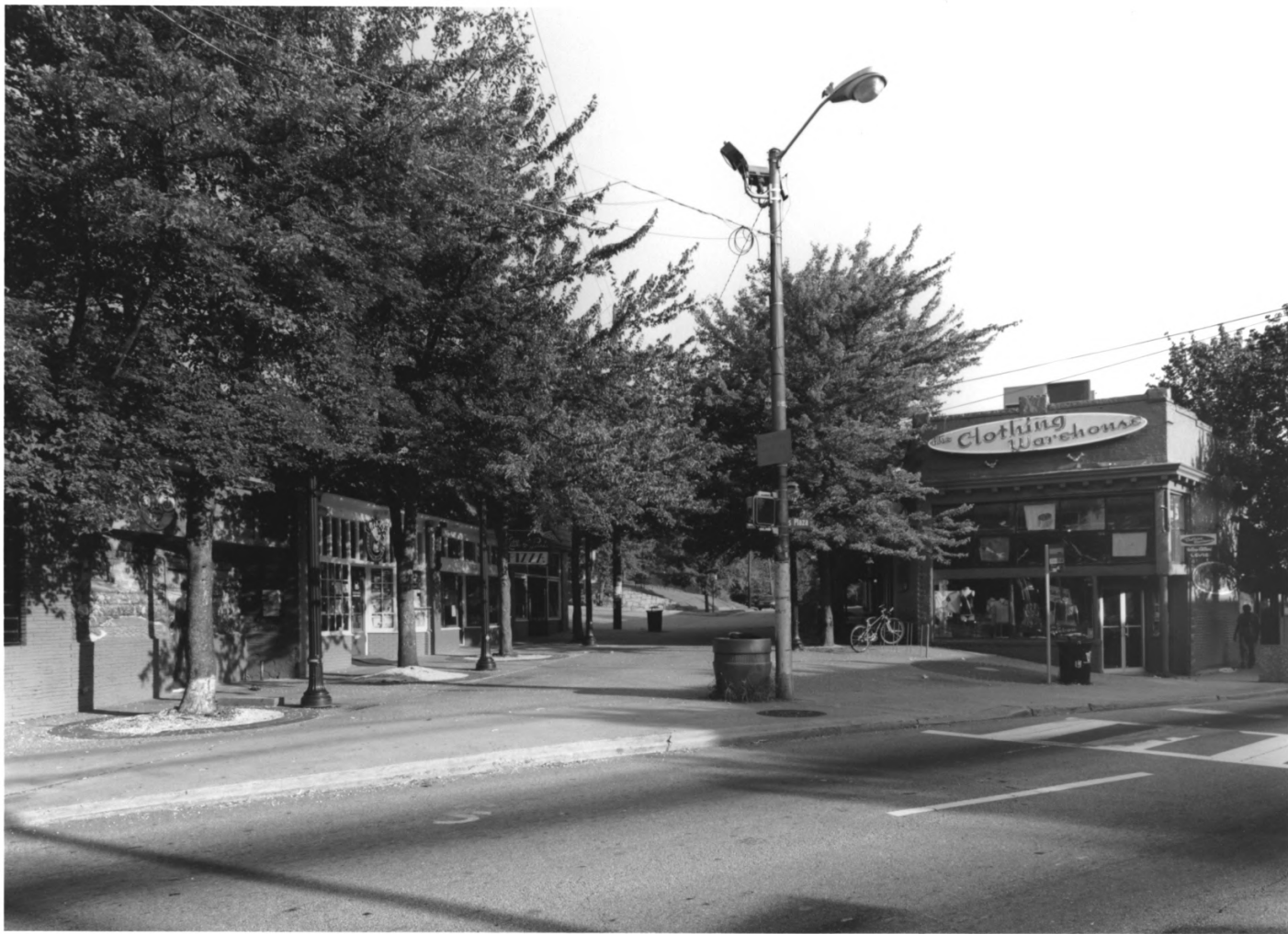
INMAN PARK-MORELAND HISTORIC DISTRICT AMENDMENT ATLANTA, FULTON COUNTY, GEORGIA PHOTOGRAPH 27 OF 42
