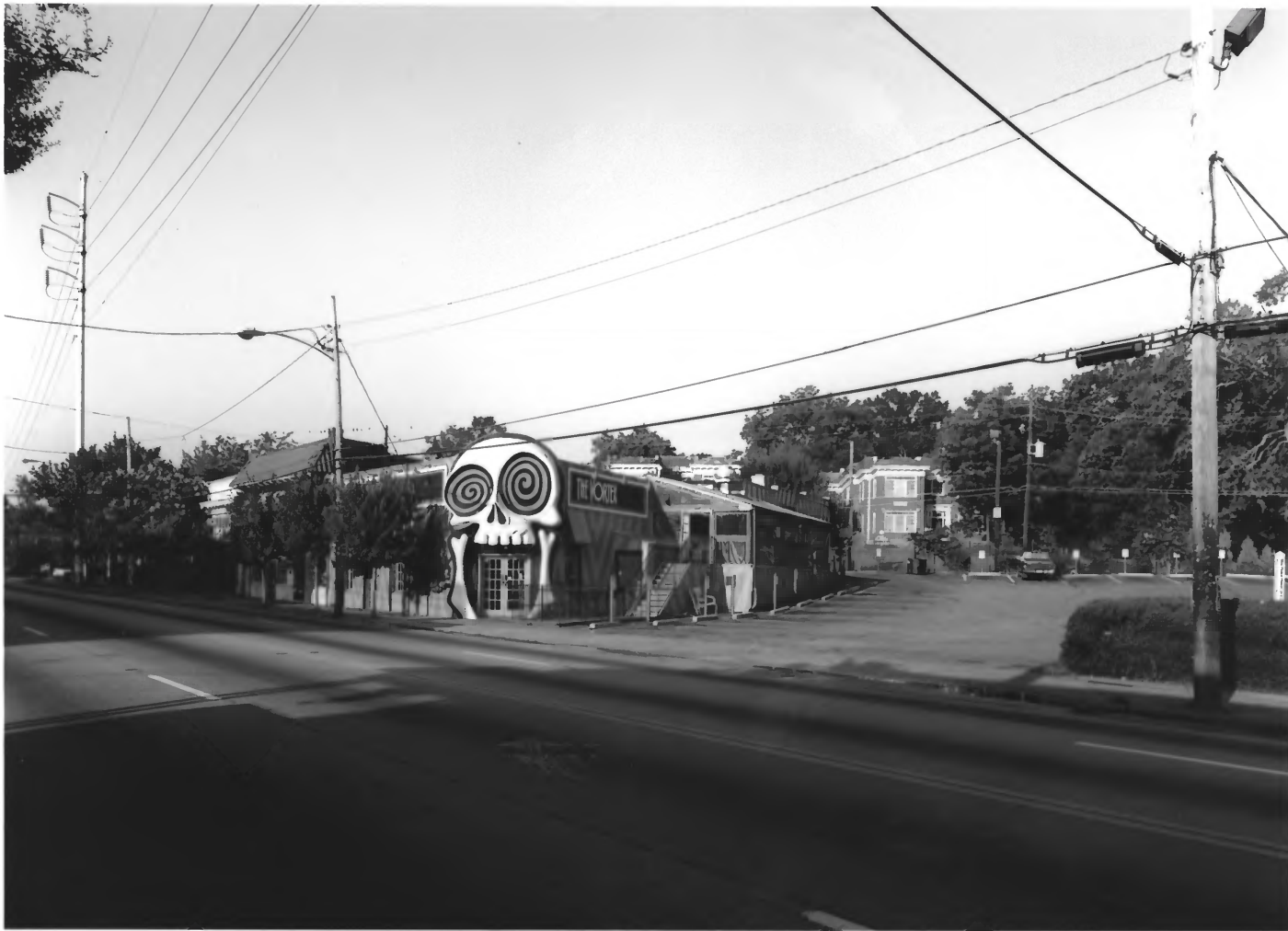
INMAN PARK - MORELAND HISTORIC DISTRICT AMENDMENT ATLANTA, FULTON COUNTY, GEORGIA PHOTOGRAPH 28 OF 42
