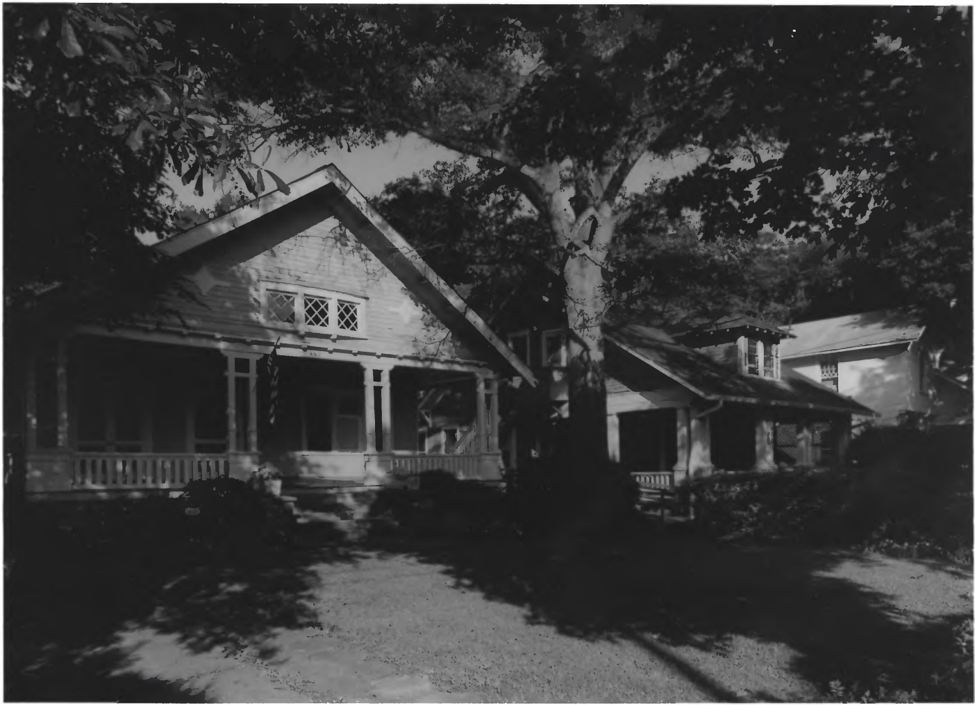
INMAN PARK-MORELAND HISTORIC DISTRICT AMENDMENT ATLANTA, FULTON COUNTY, GEORGIA PHOTOGRAPH 42 OF 42
