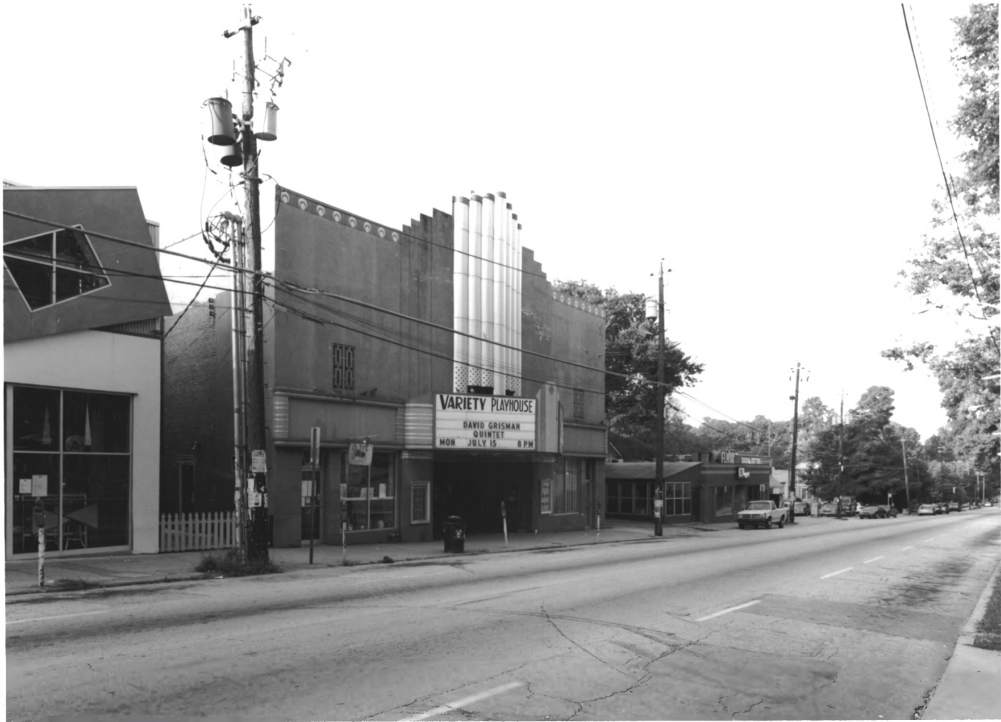
INMAN PARK-MORELAND HISTORIC DISTRICT AMENDMENT ATLANTA, FULTON COUNTY, GEORGIA PHOTOGRAPH 21 OF 42
