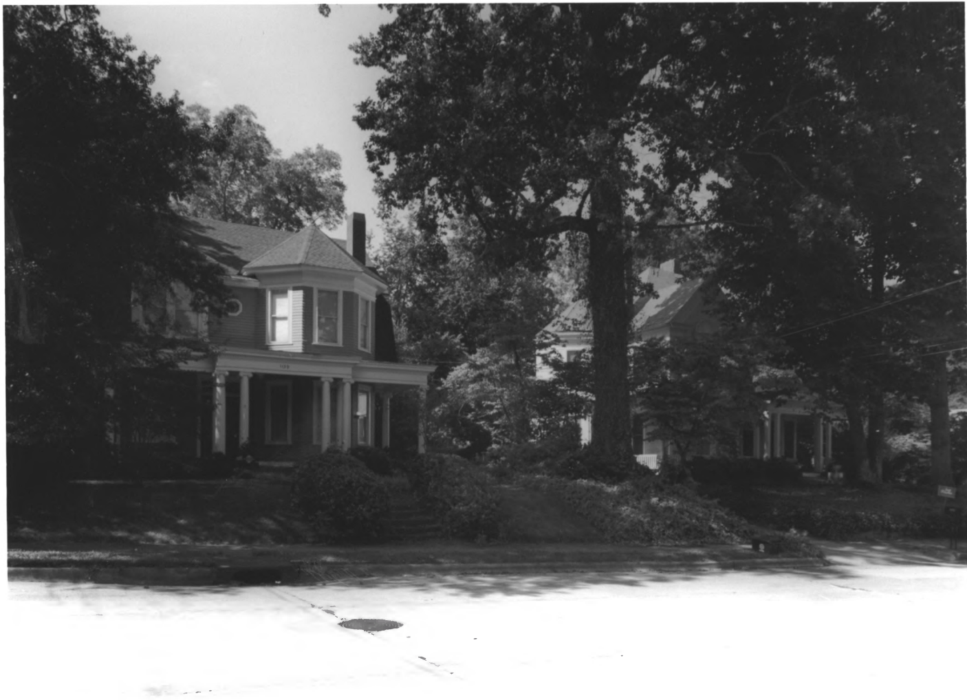
INMAN PARK-MORELAND HISTORIC DISTRICT AMENDMENT ATLANTA, FULTON COUNTY, GEORGIA PHOTOGRAPH 30 OF 42
