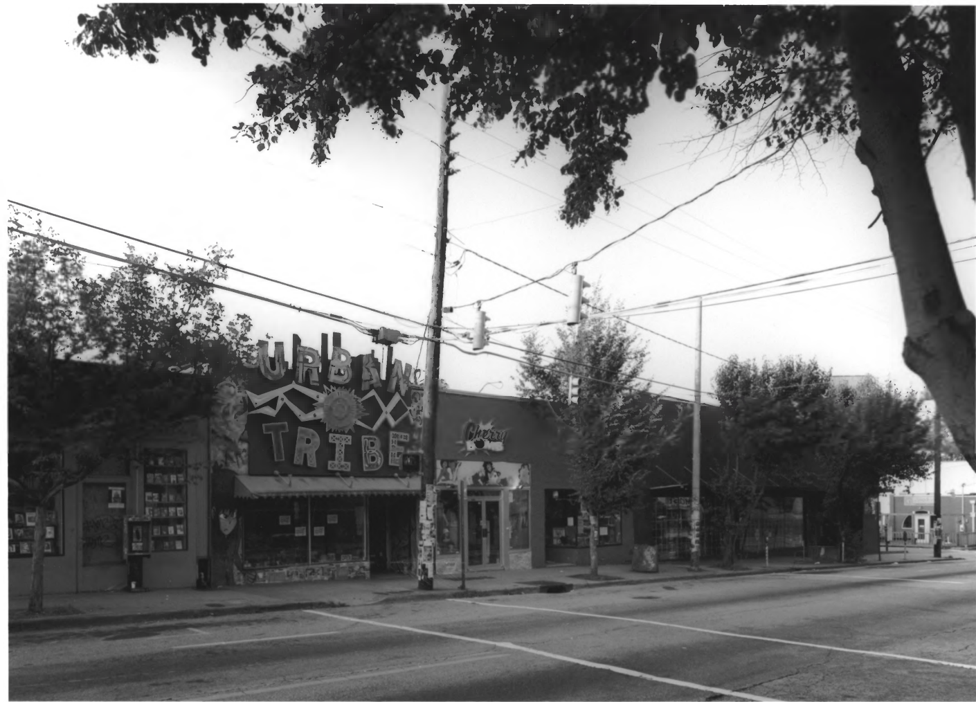
INMAN PARK-MORELAND HISTORIC DISTRICT AMENDMENT ATLANTA, FULTON COUNTY, GEORGIA PHOTOGRAPH 19 OF 42
