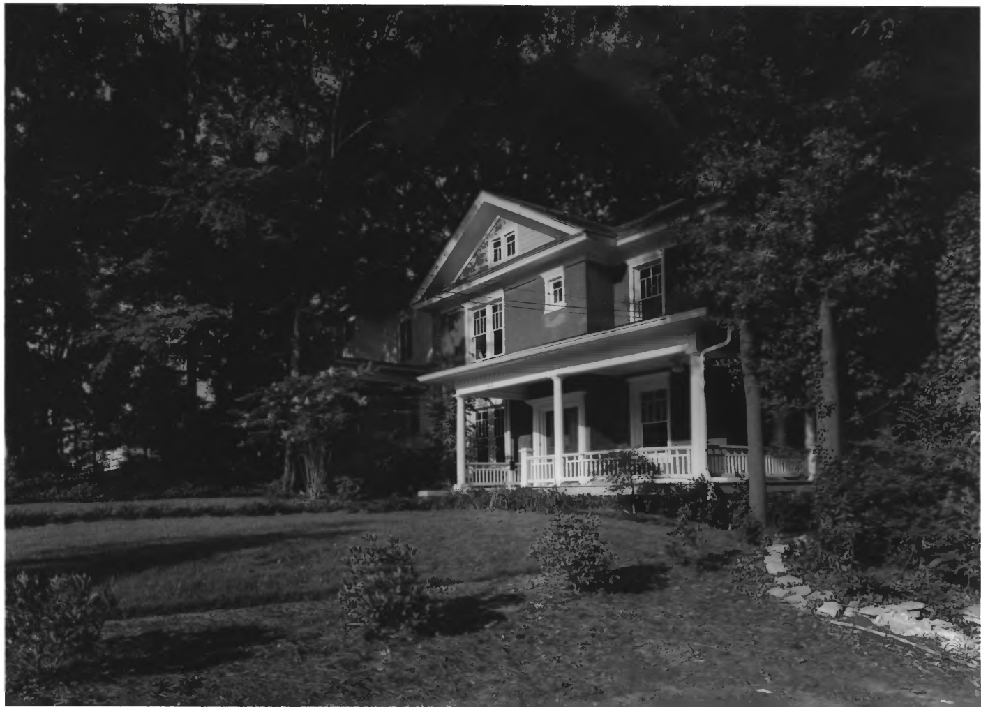
INMAN PARK-MORELAND HISTORIC DISTRICT AMENDMENT ATLANTA, FULTON COUNTY, GEORGIA PHOTOGRAPH 30 OF 42
