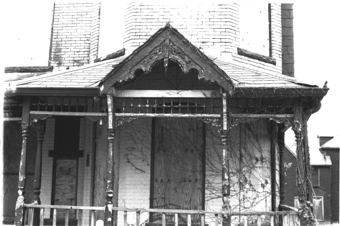
#7 824 N. Alabama St. (Detail) Marion County, Indiana
