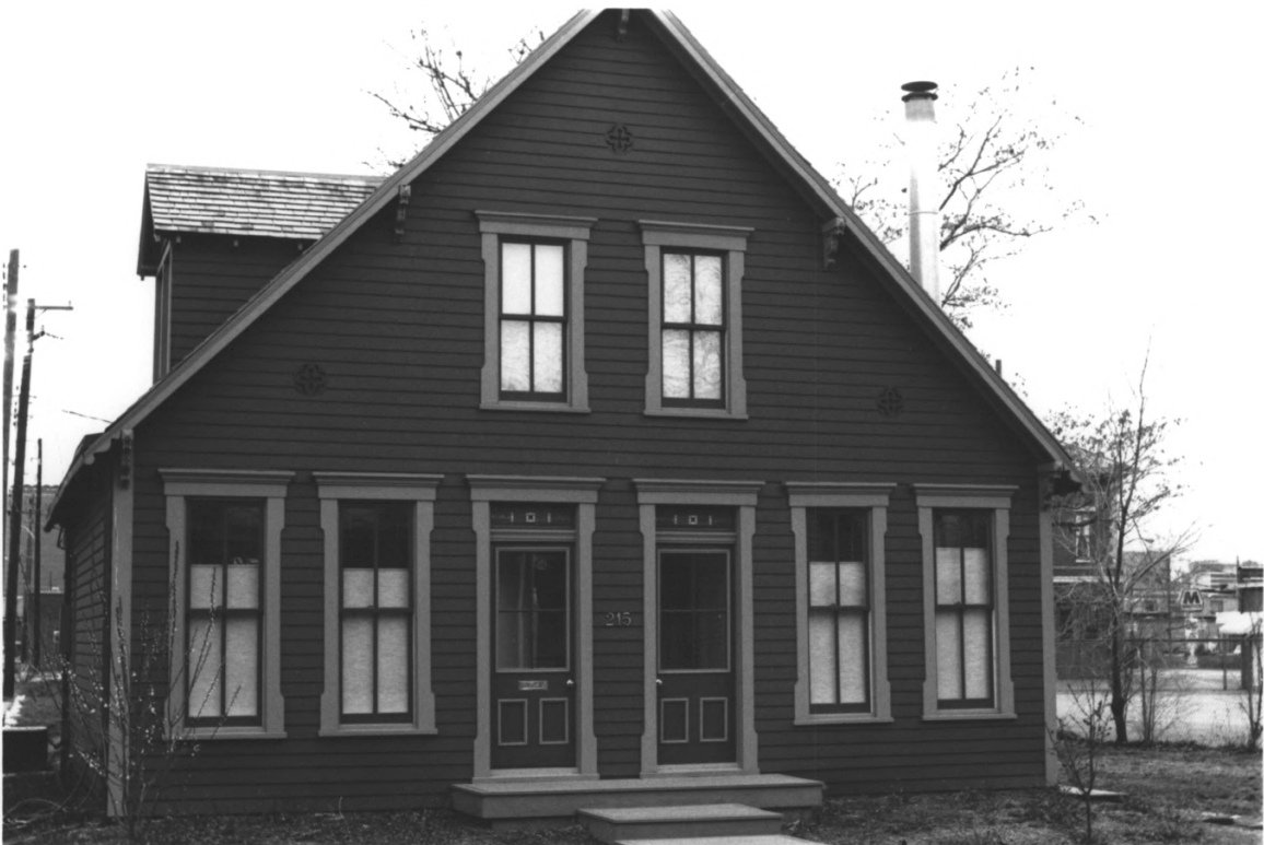
#63 215-217 E 10th St. (After renovation) Marion County, Indiana (See also photo #20)
